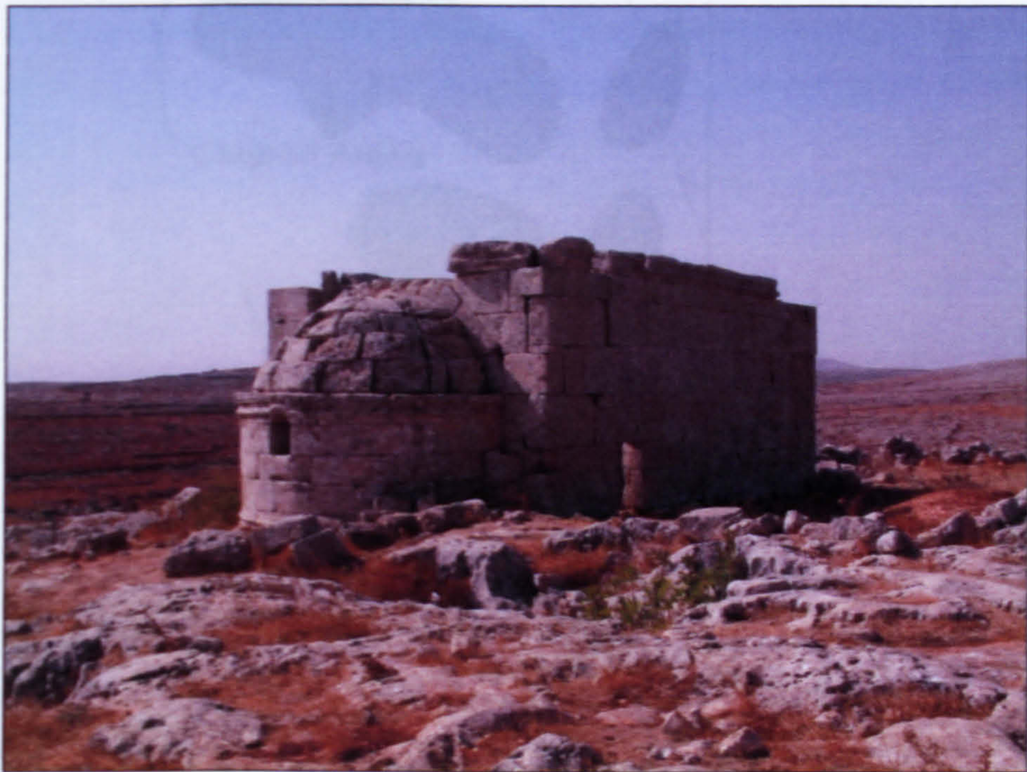
Figure 106: Kharab Shams monastic church from the north-east
