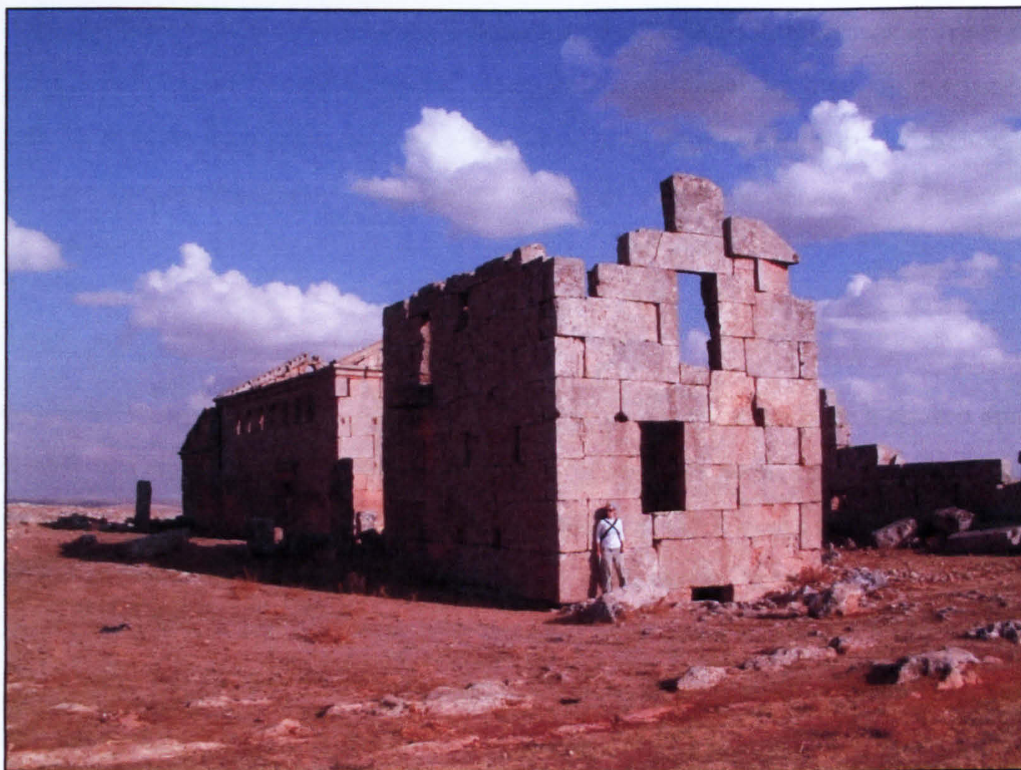
Figure 78: The monastic site of Sarjibla (south), showing the press in the foreground, the church behind and an accommodation block to the right.
