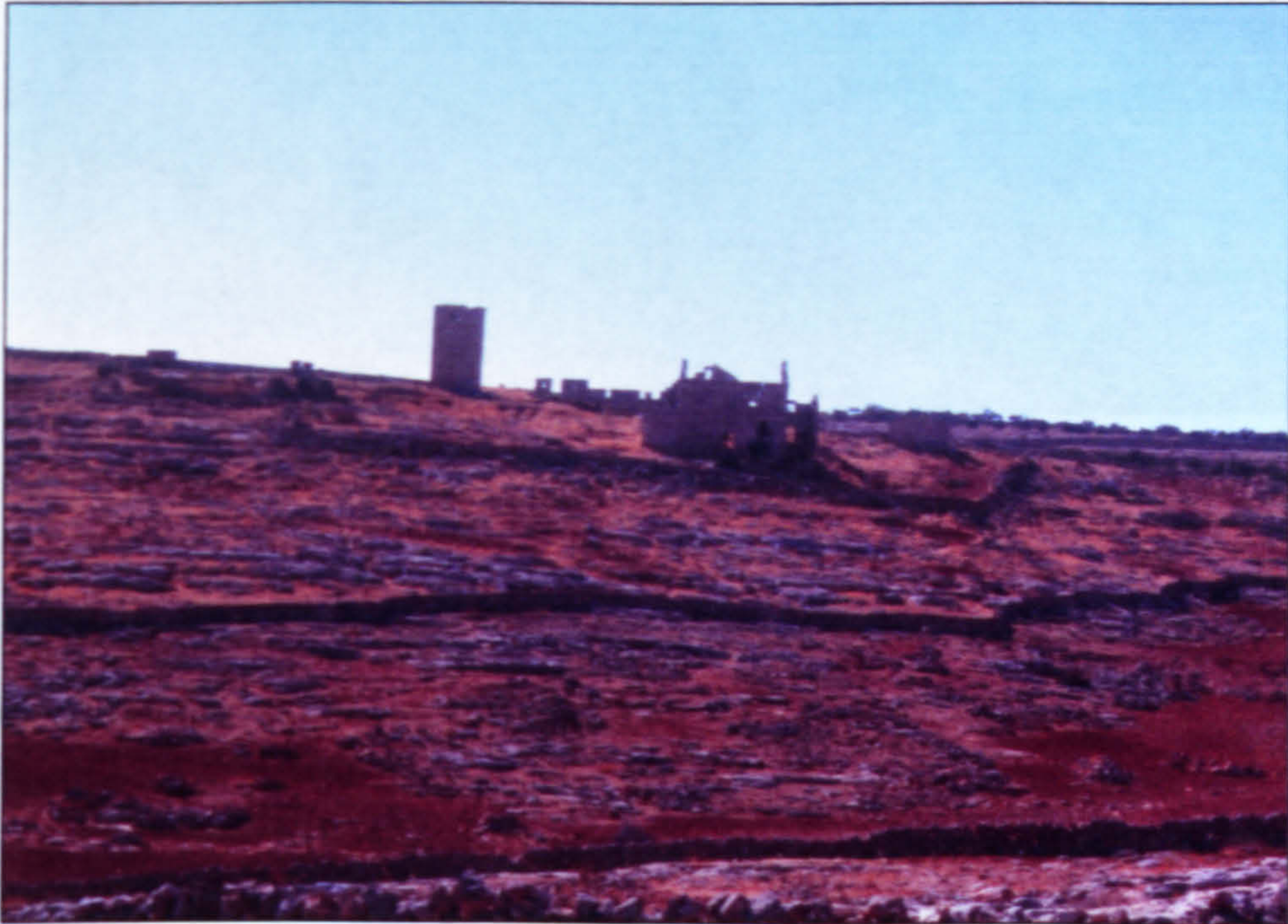
Figure 92: General view of Qasr al-Brad from the east
