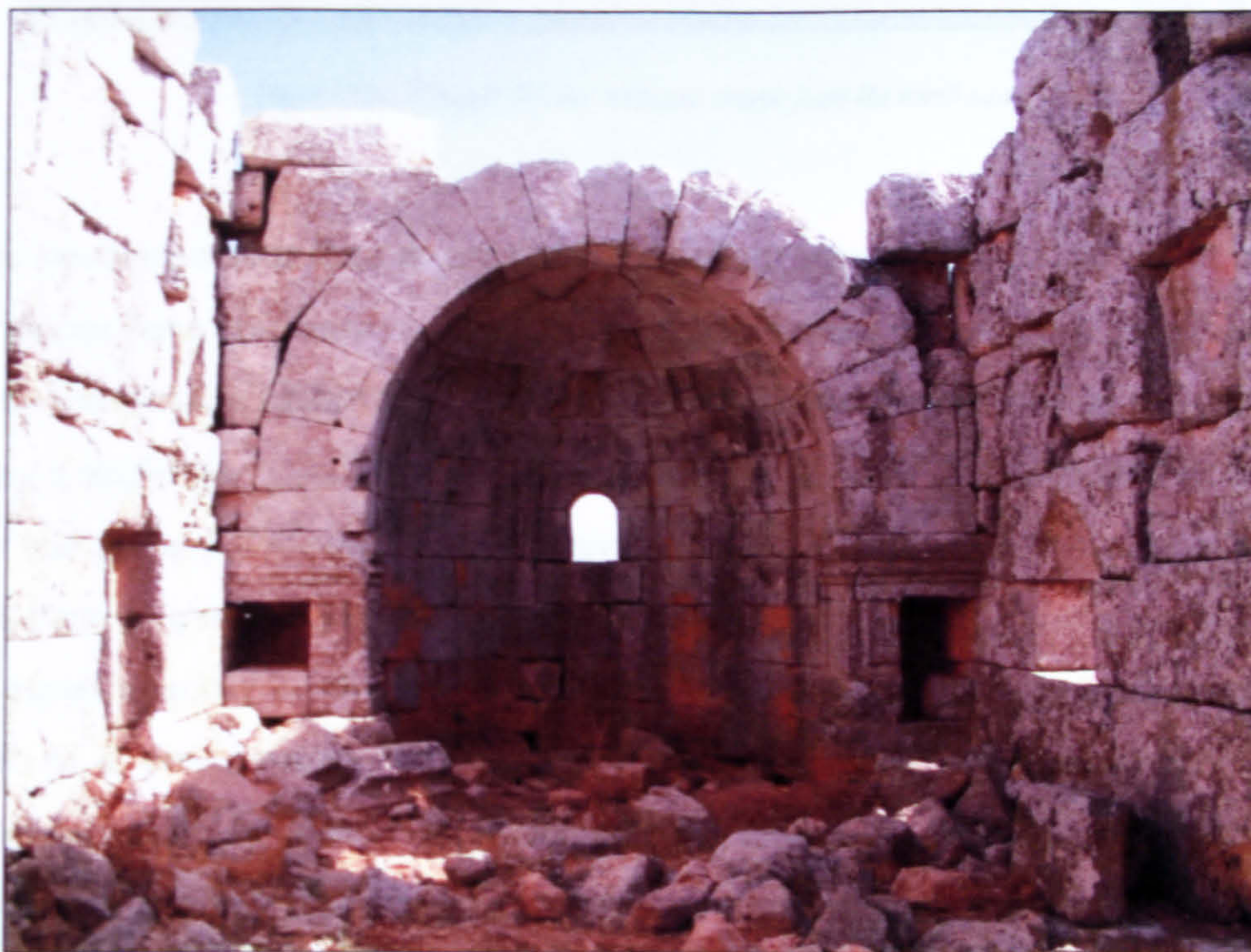
Figure 105: East end of monastic church, with possible reuse of masonry shown in the aumbries to left and right
