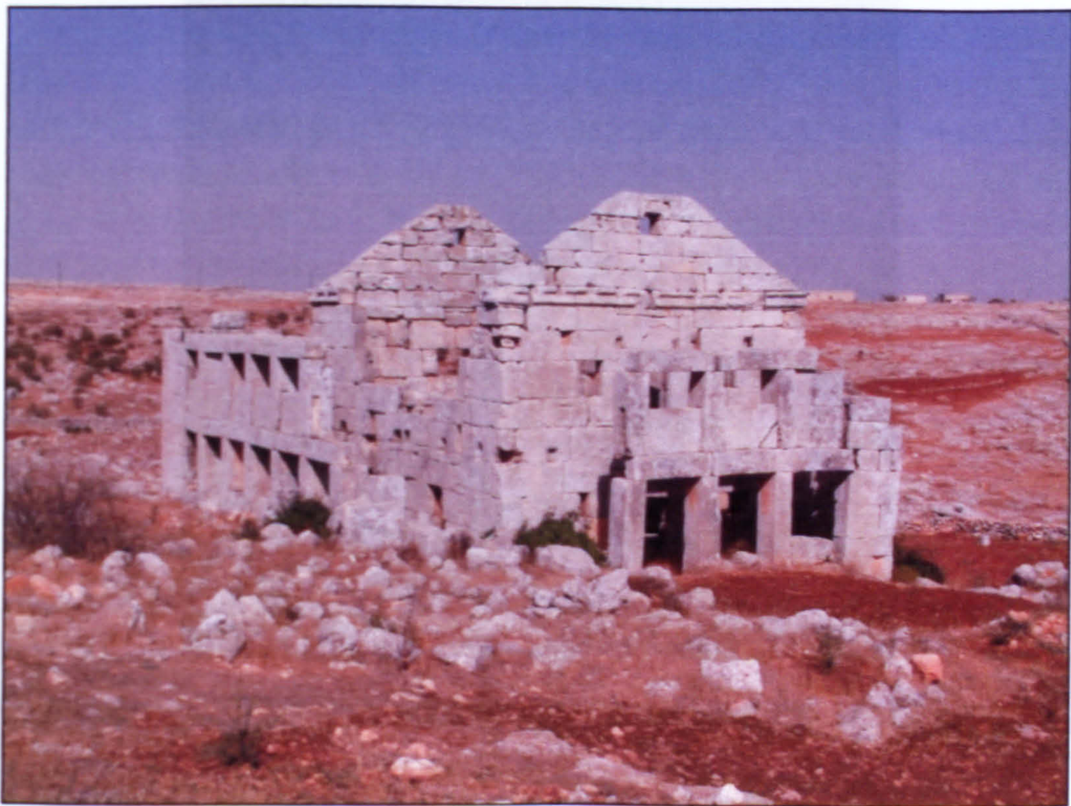
Figure 94: The main accommodation building at Qasr al-Brad
