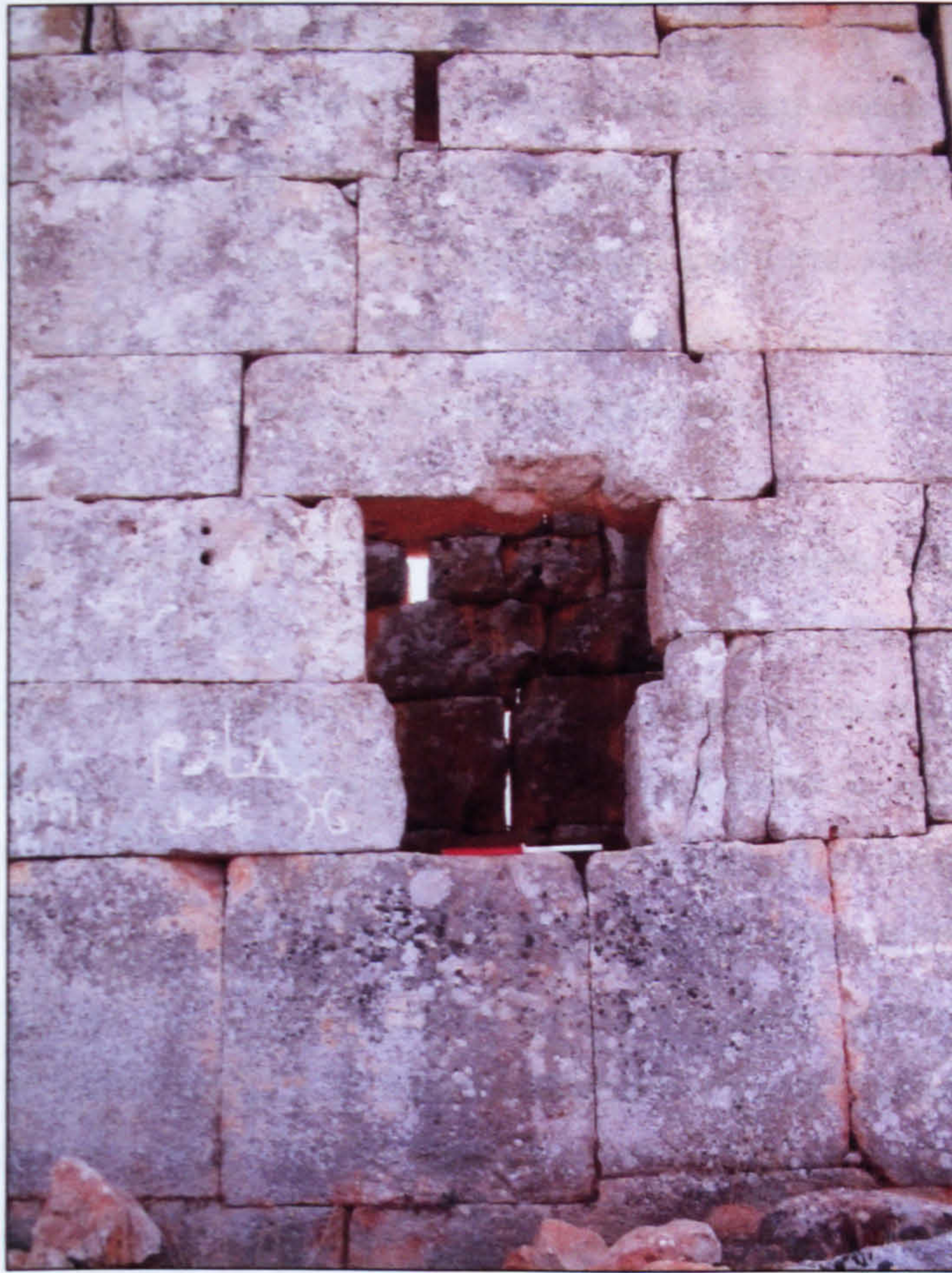
Figure 42: An example of Tate's 'single orthogonal' construction technique at Burj Jalabah
