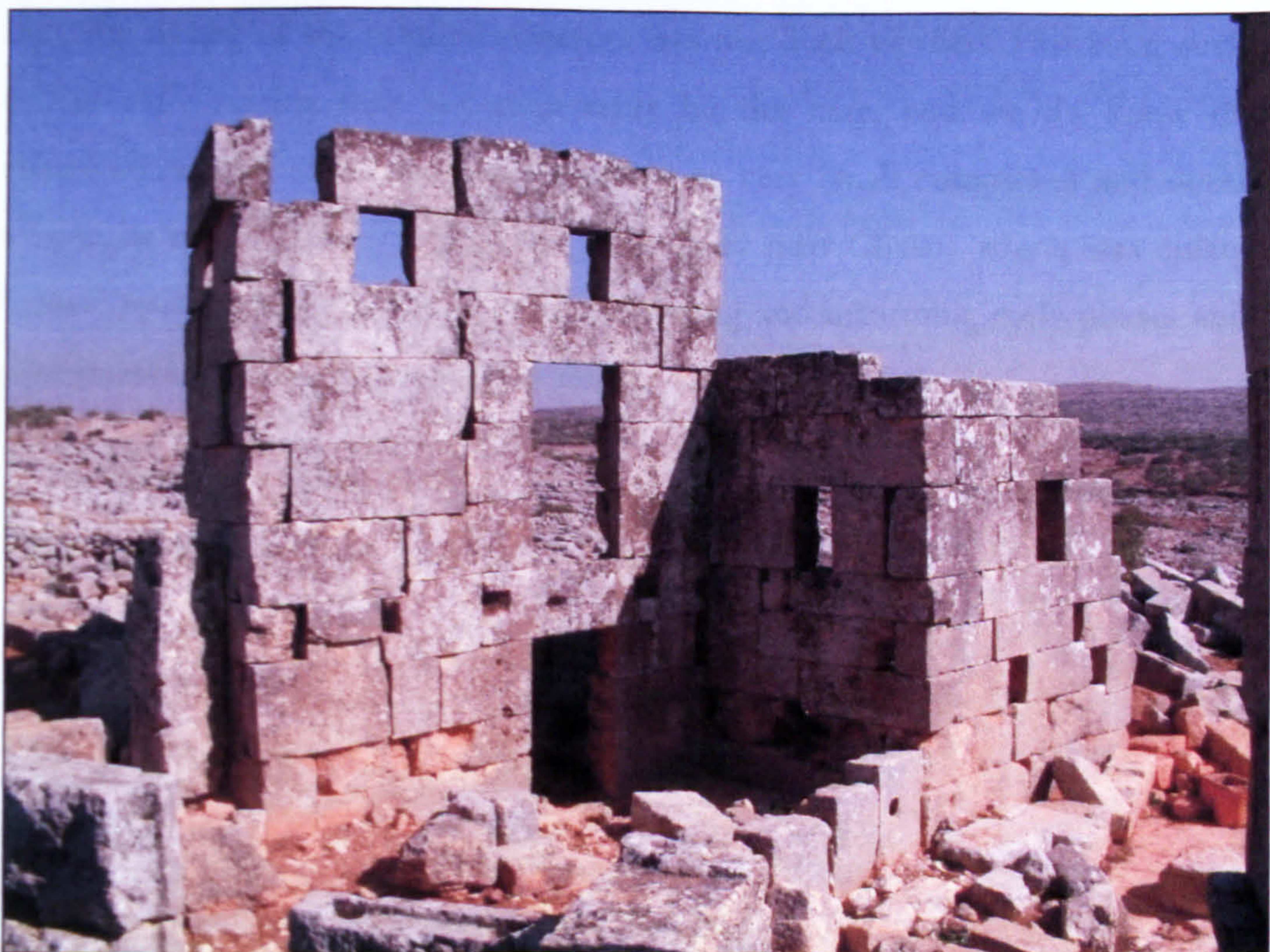
Figure 43: The 'communal habitation building' at Dayr Dehes, elements of which may date to the late fourth century
