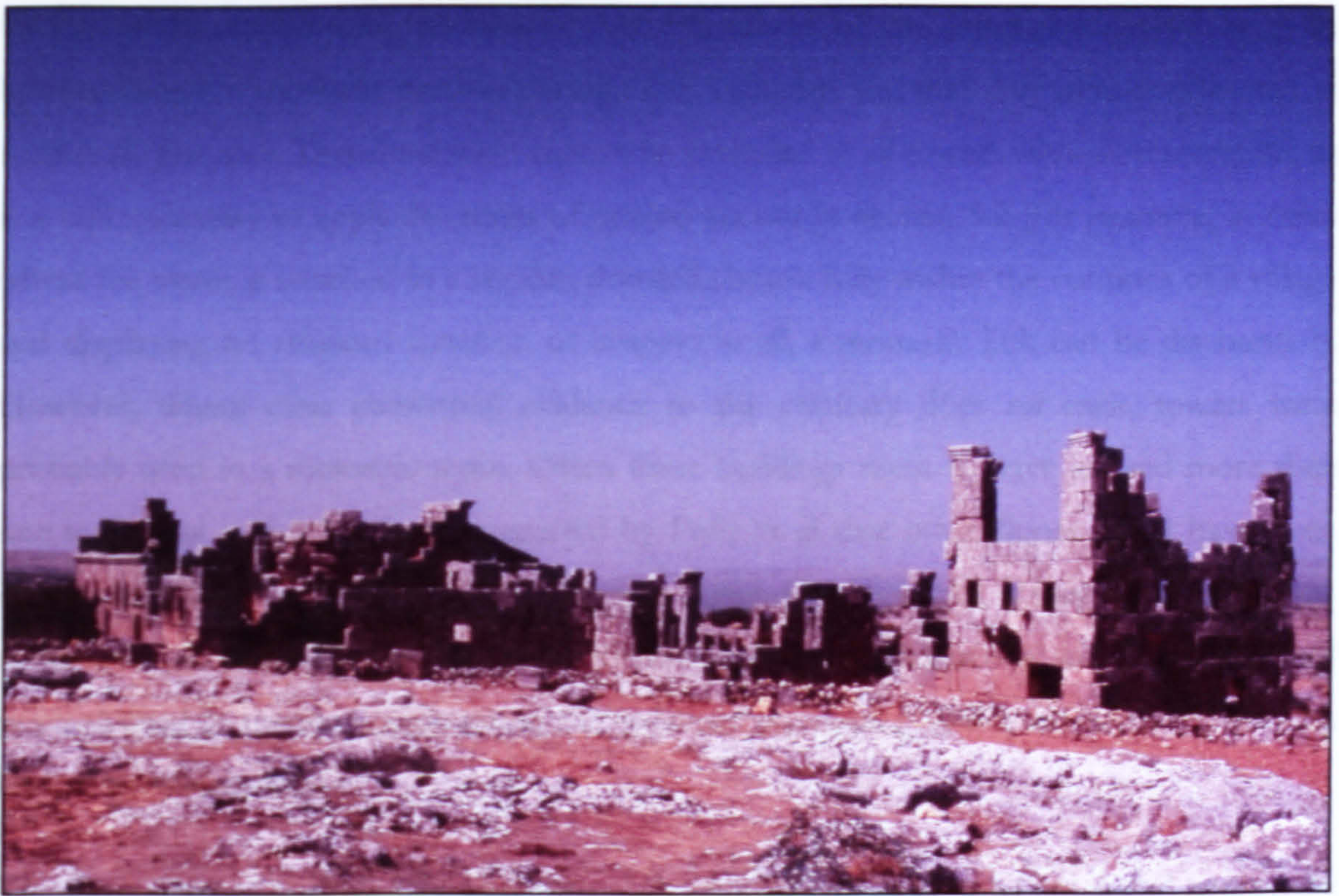
Figure 81: A monastic tower at the site of Dayr Sim'an (north-west; to the right of the picture)
