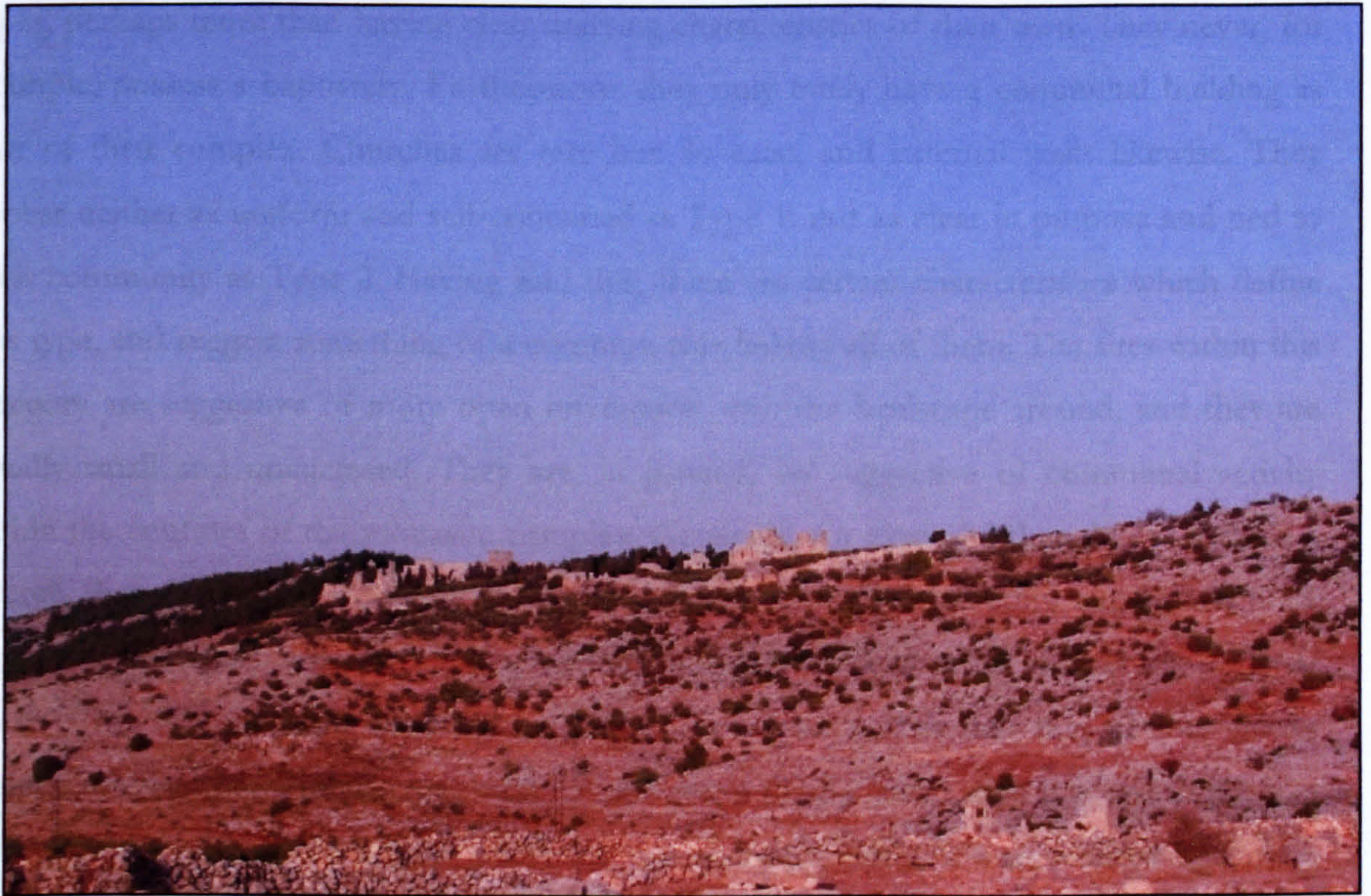
Figure 79: General view of Qal'at Sim'an, with the baptistery complex to the right
