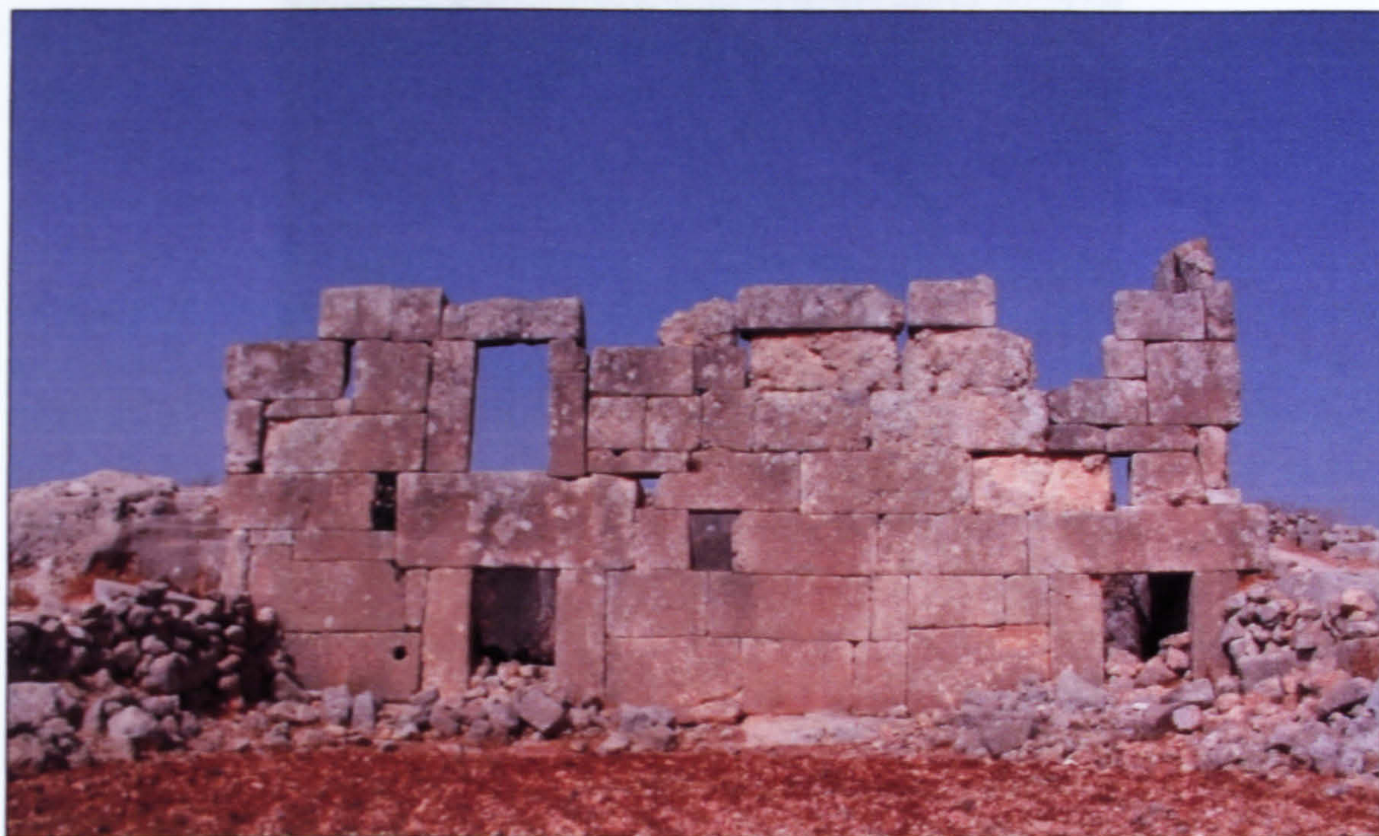
Figure 110: Kharab Shams press building from the south
