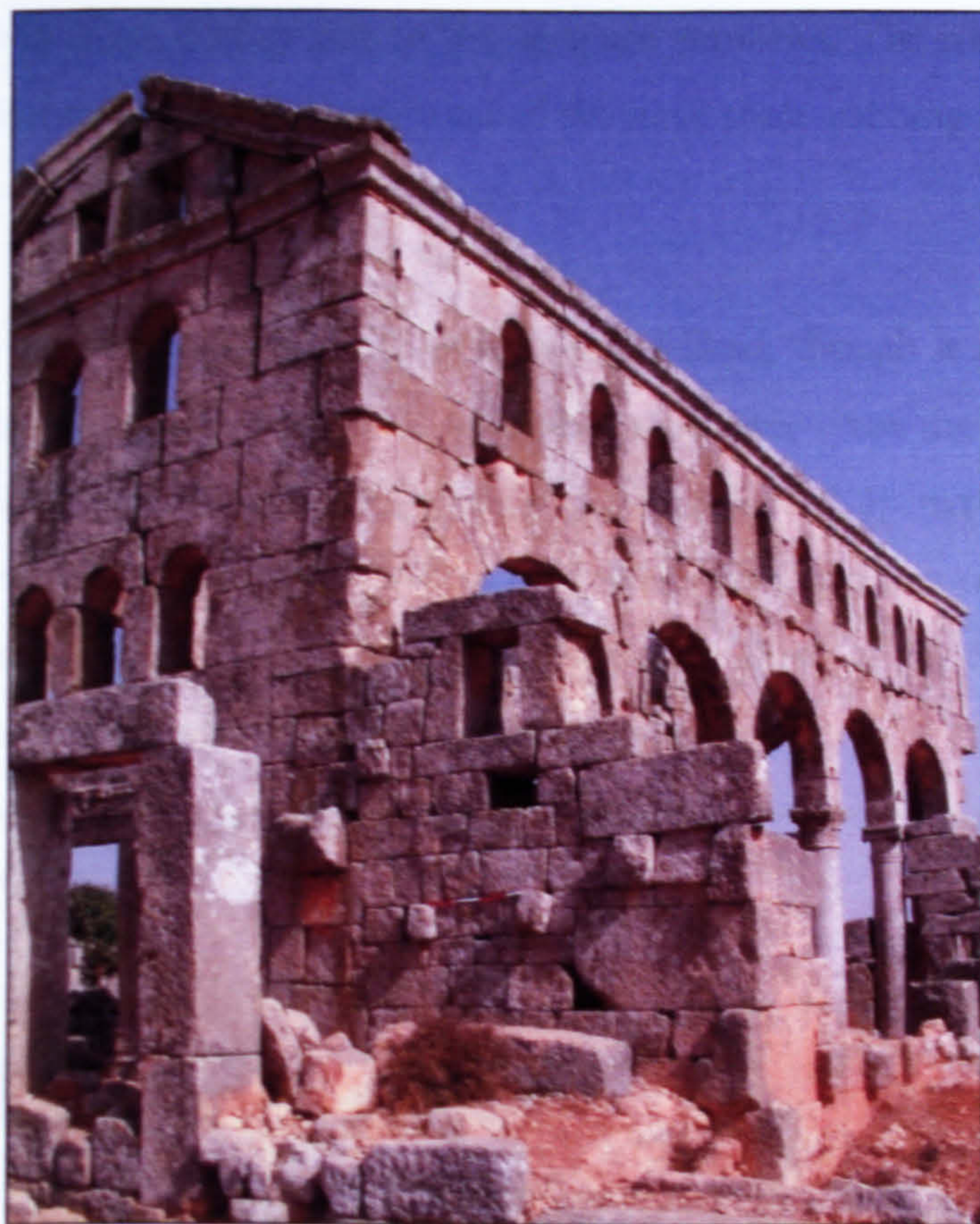
Figure 104: Kharab Shams church showing added south aisle (scale: 1 m)
