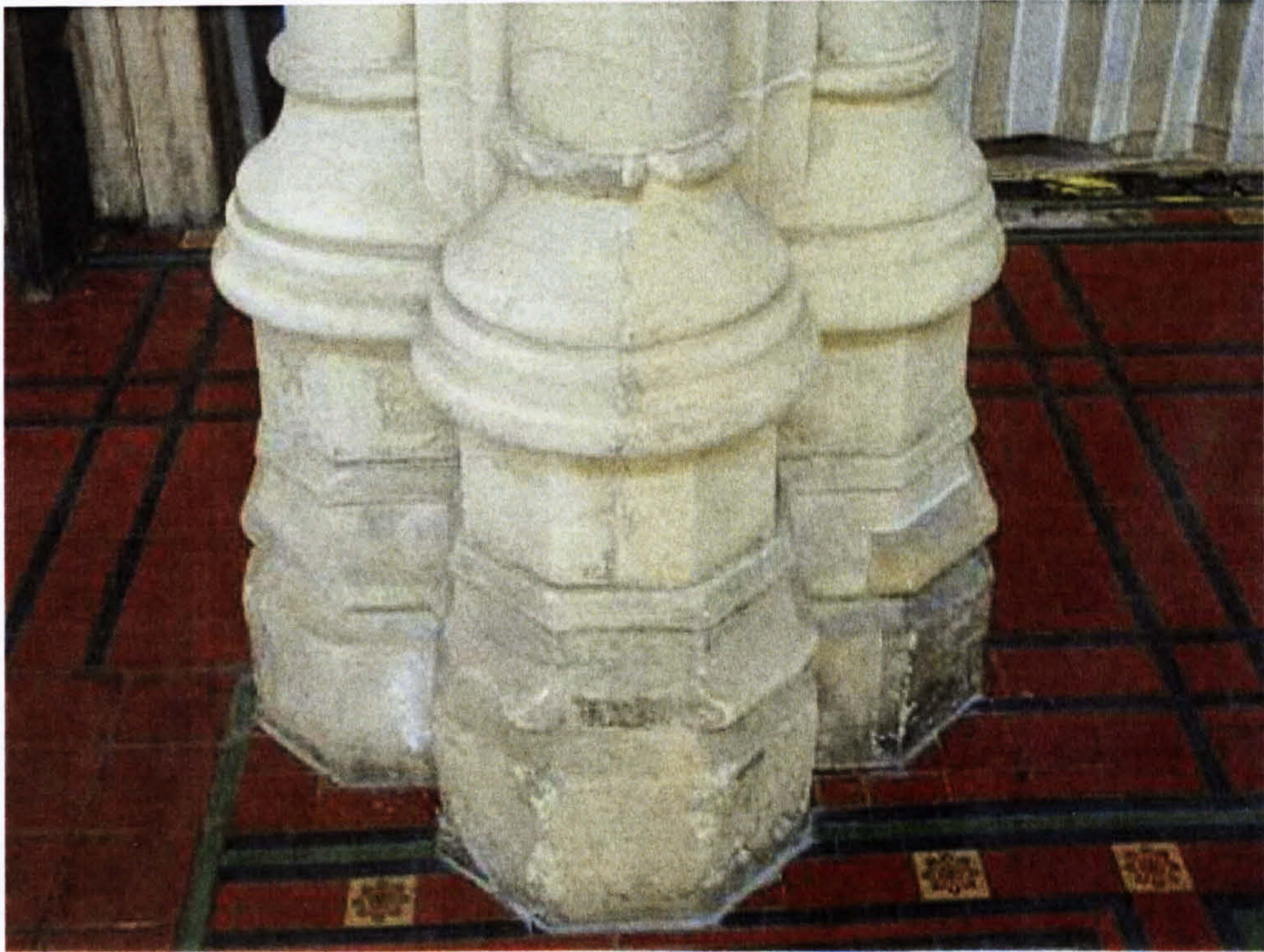
Plate 2 - St. Michael-le-Belfrey, York: Pier base
