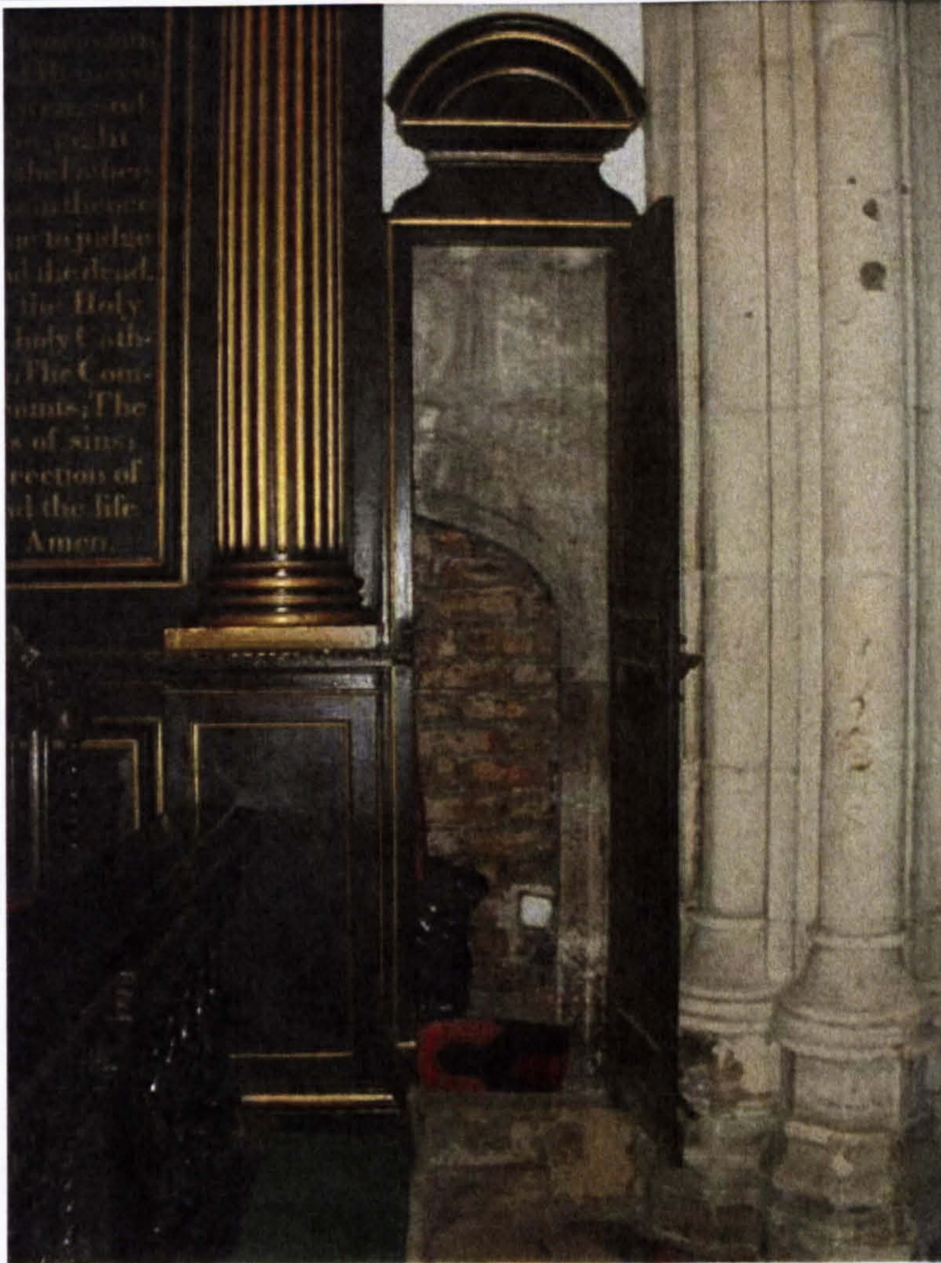
Plate 9 - St. Michael-le-Belfrey, York: Original vestry door (now behind early eighteenth century reredos)
