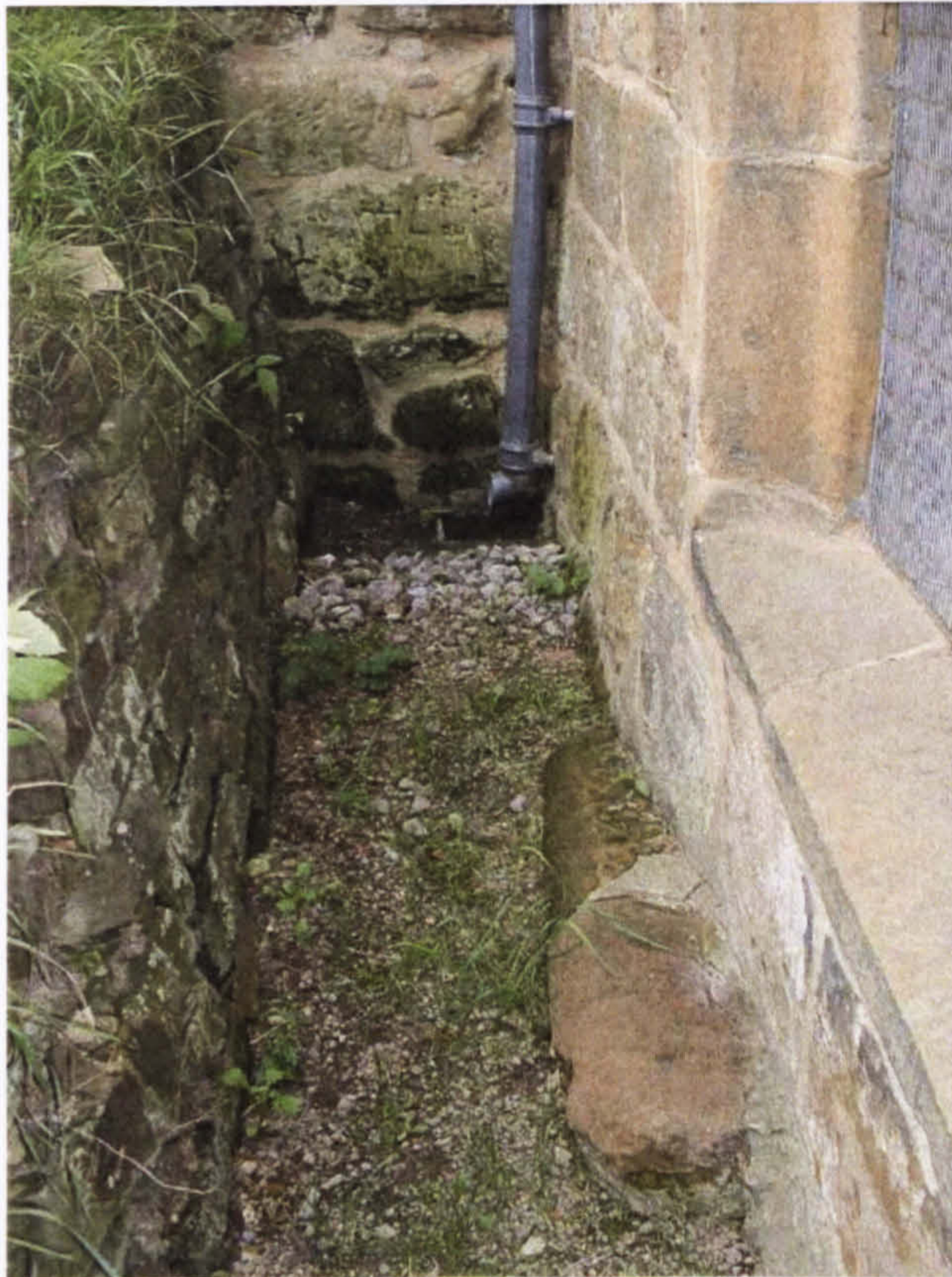
Plate 62 - St. Mary, Thirsk: Foundation of earlier chancel
