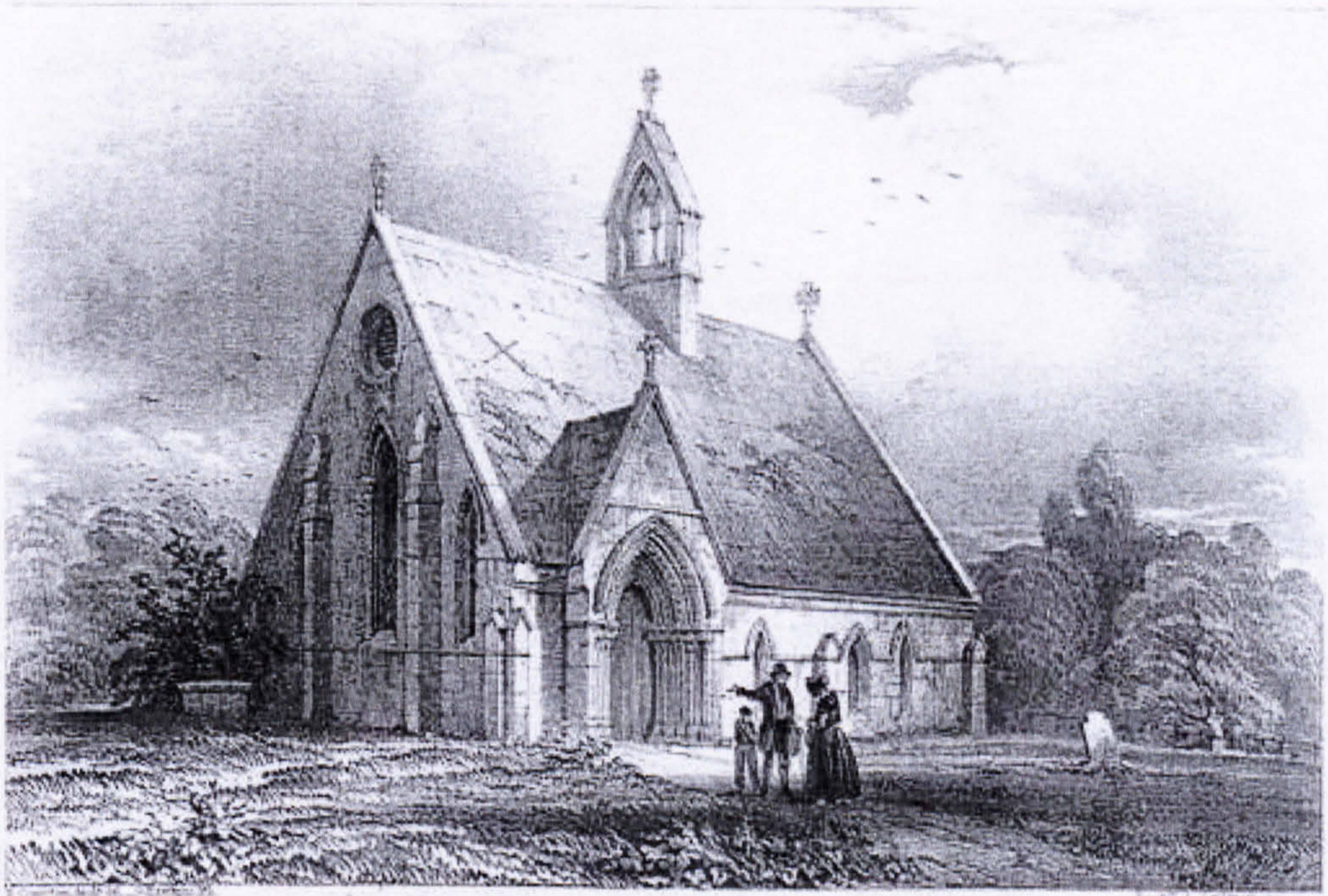
SKELTON CHURCH. South West View.
