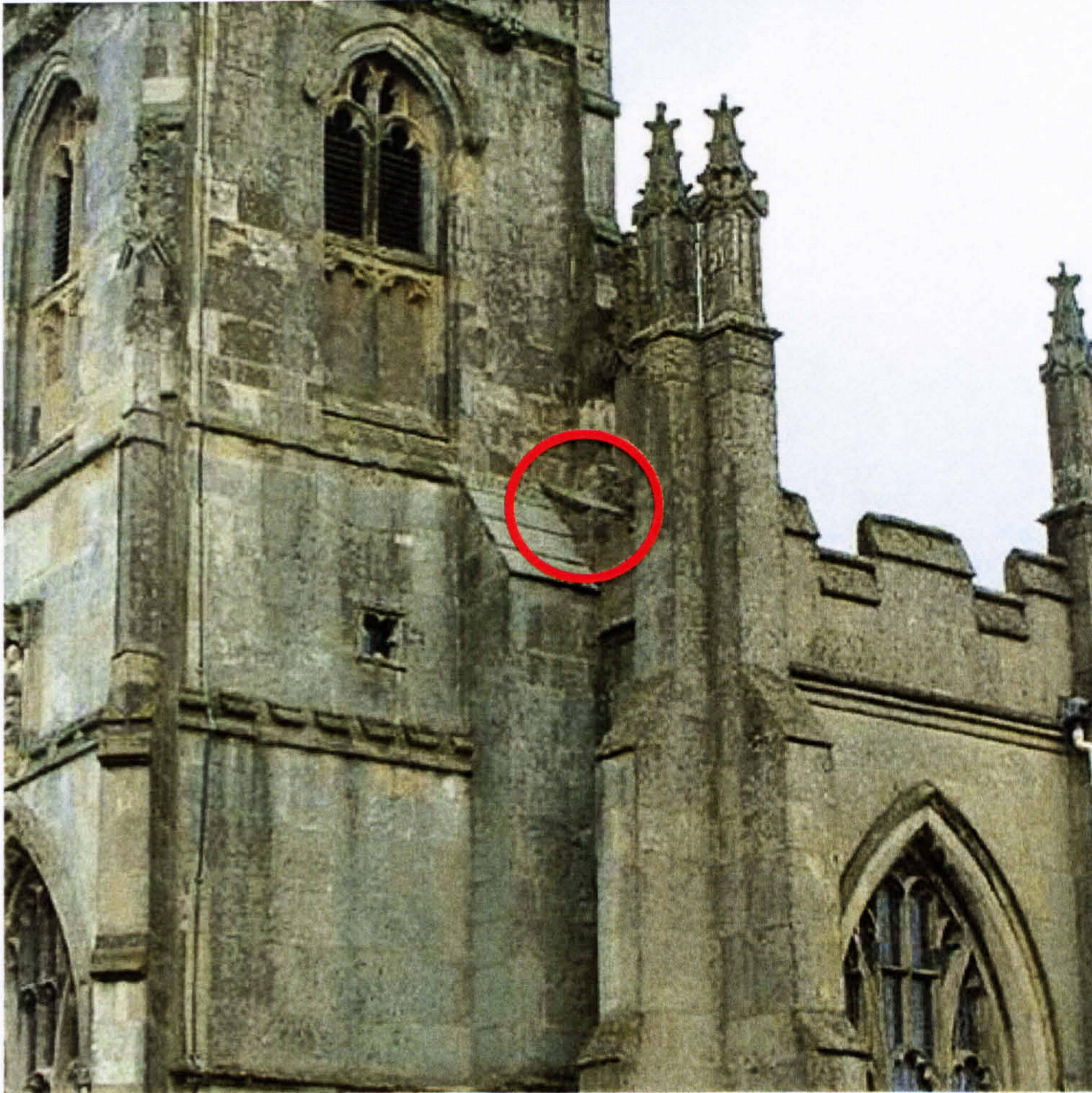
Plate 13 - St. Augustine, Skirlough: Exterior, join of tower and west wall (Possible gable fragment circled)
