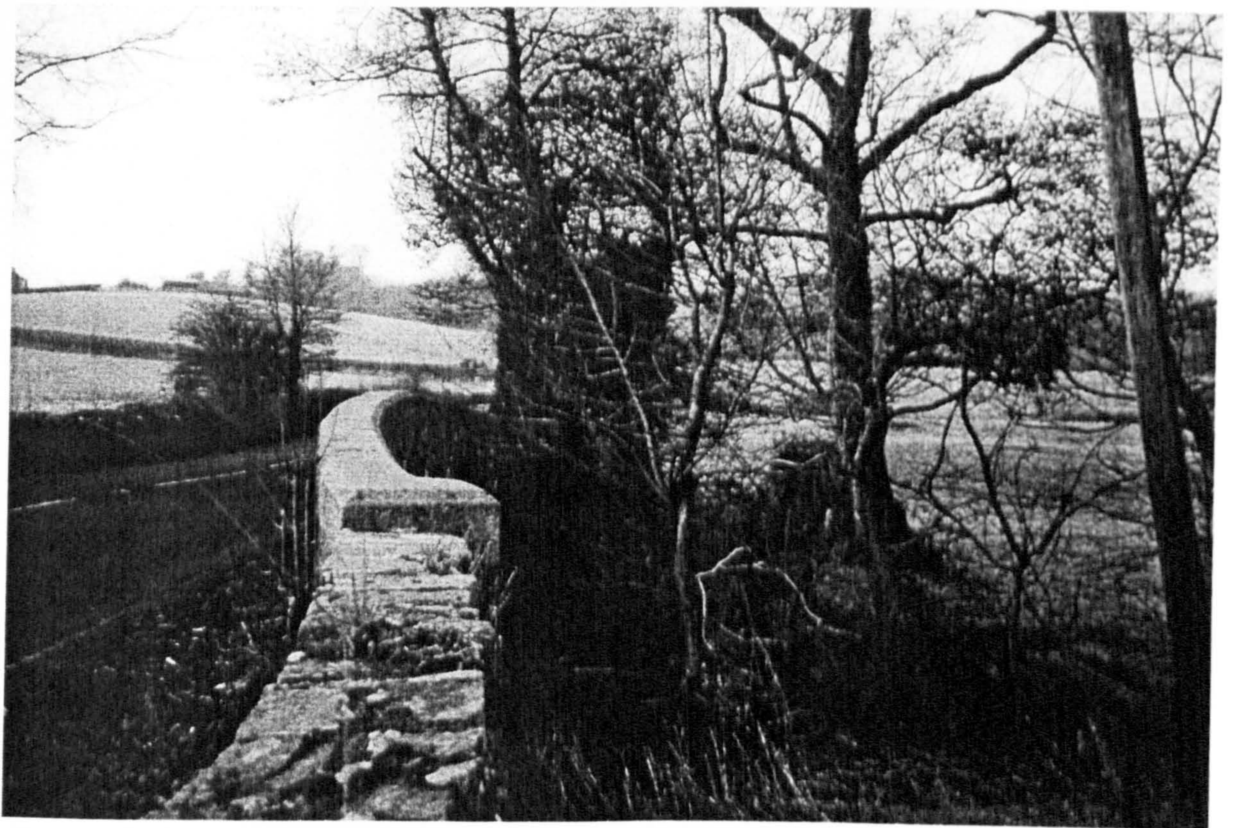
Figure 45: The modern crossing of Creedy Bridge (S 255, S 387, S 890).
