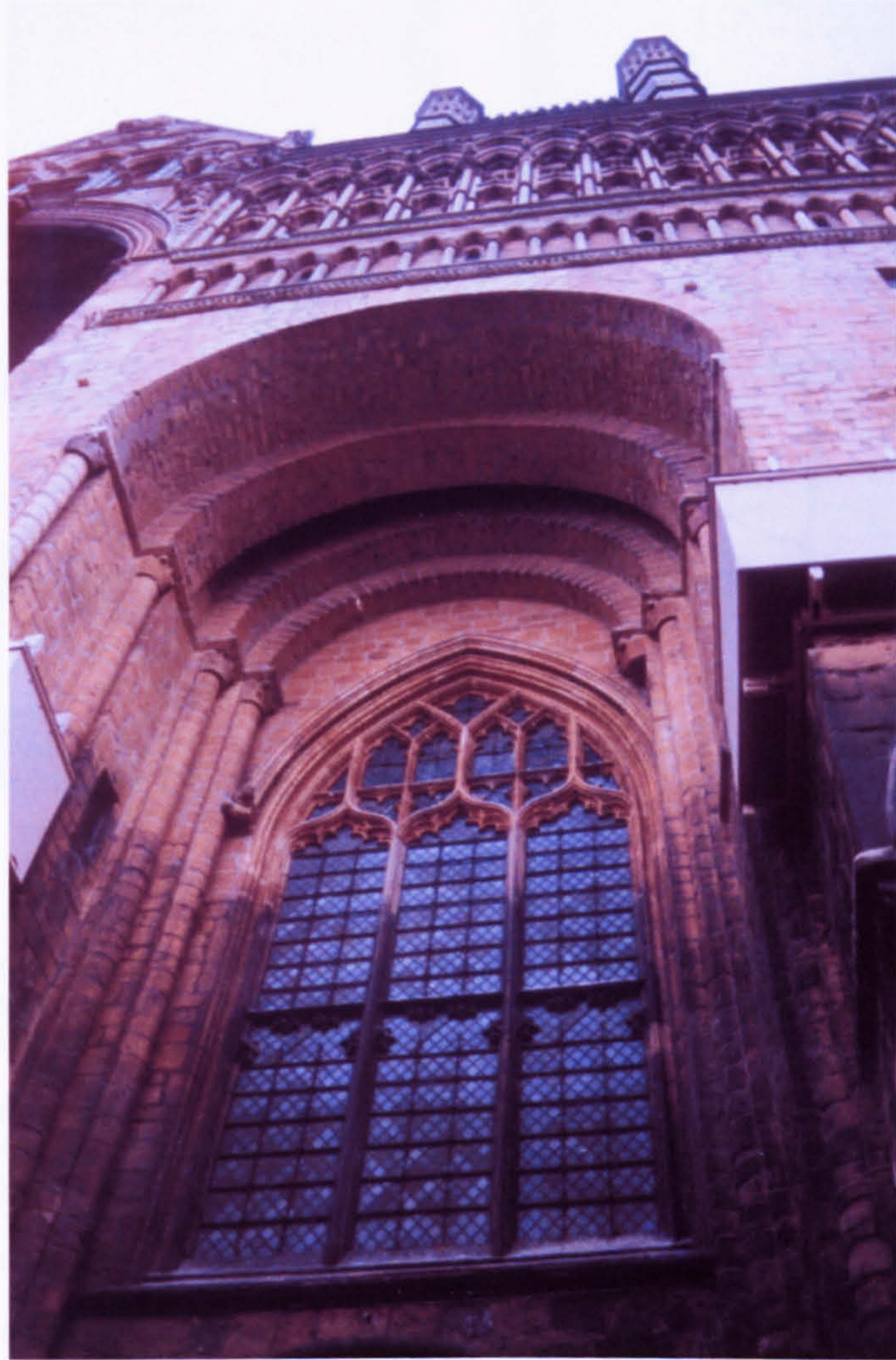
29. Southern bay of the west front, Lincoln Cathedral, showing machicolation slot. 11th century.
