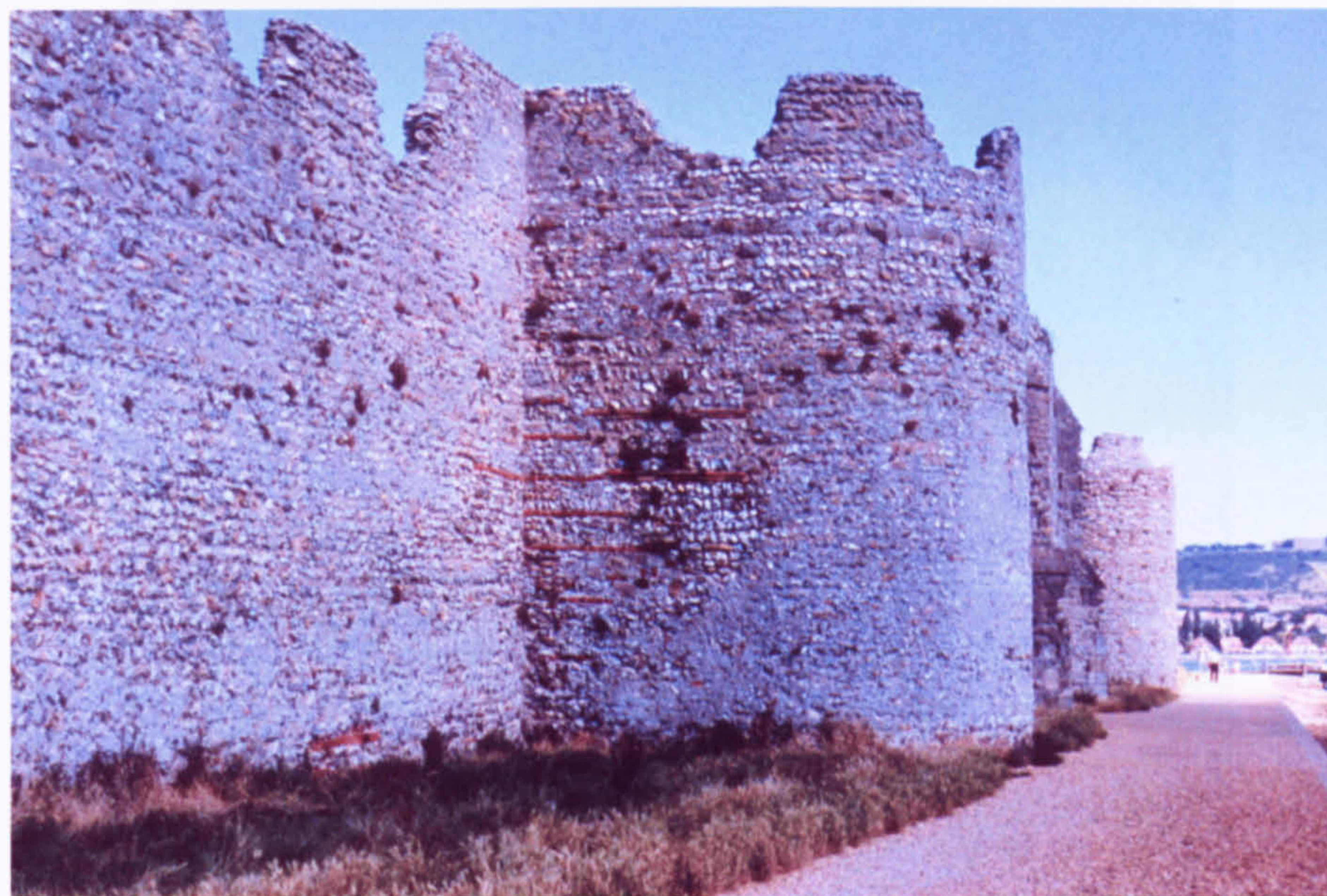
35. Portchester Castle, Roman fort wall, south bastion of the Roman east gateway, showing tile-banded Roman masonry and medieval flint banded repairs, above. Medieval work ?14th century, Roman walls of the last quarter of the 3rd century A.D.
