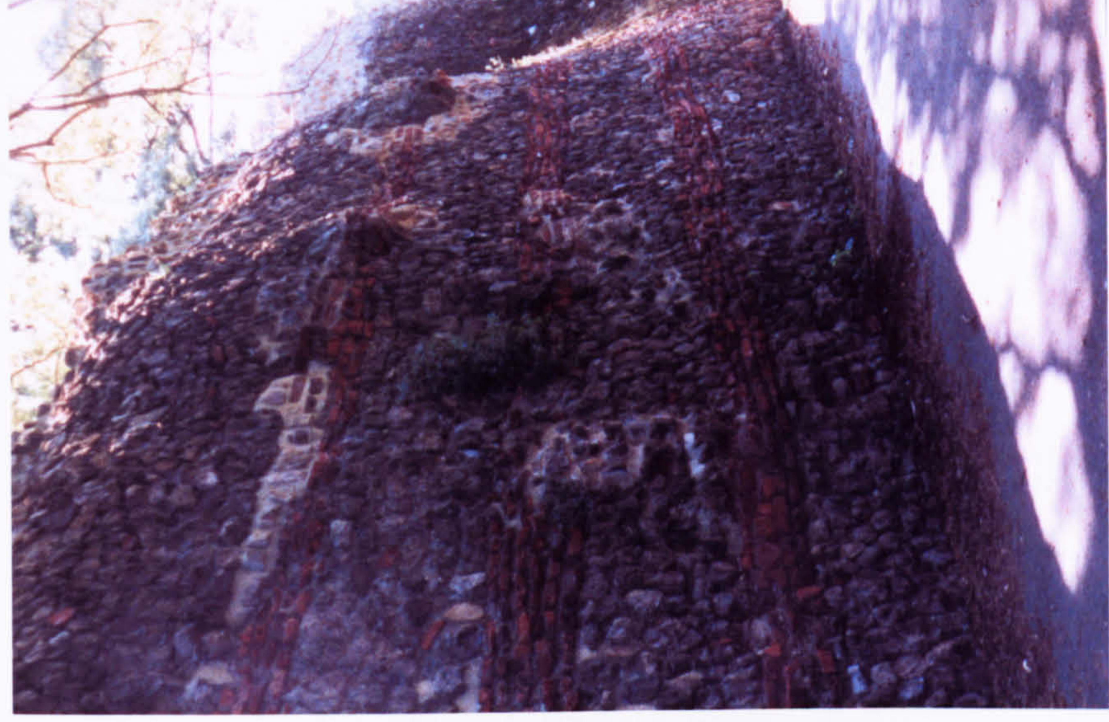
7. Roman wall in Colchester Castle Park, showing banded masonry. C.60 A.D.
