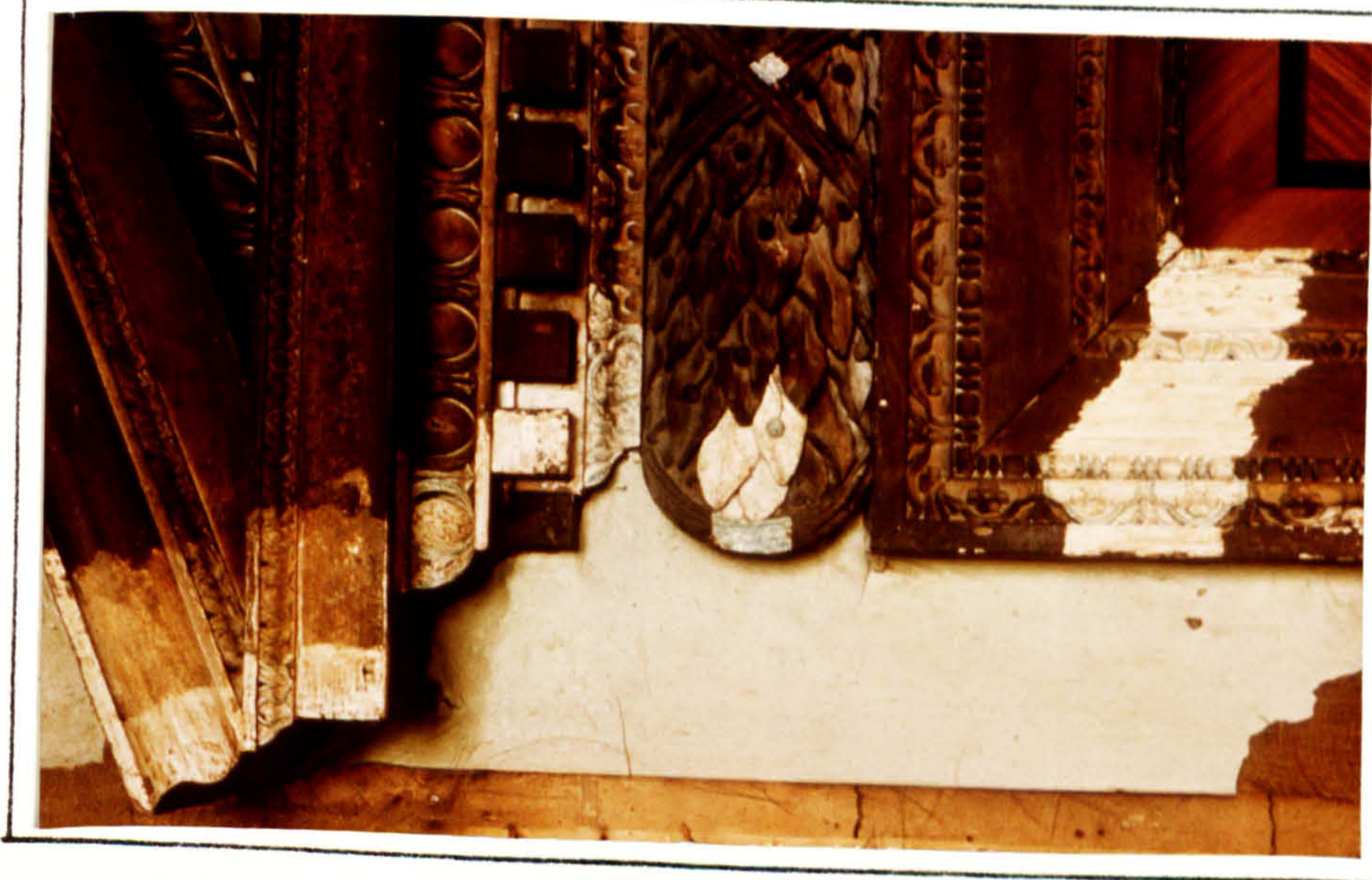
FIG. 130 ORIGINAL BLUE PICKING OUT (C. 1770) PARTLY EXPOSED ON DOORCASE OF SALOON IN THE CASINO - MARINO
