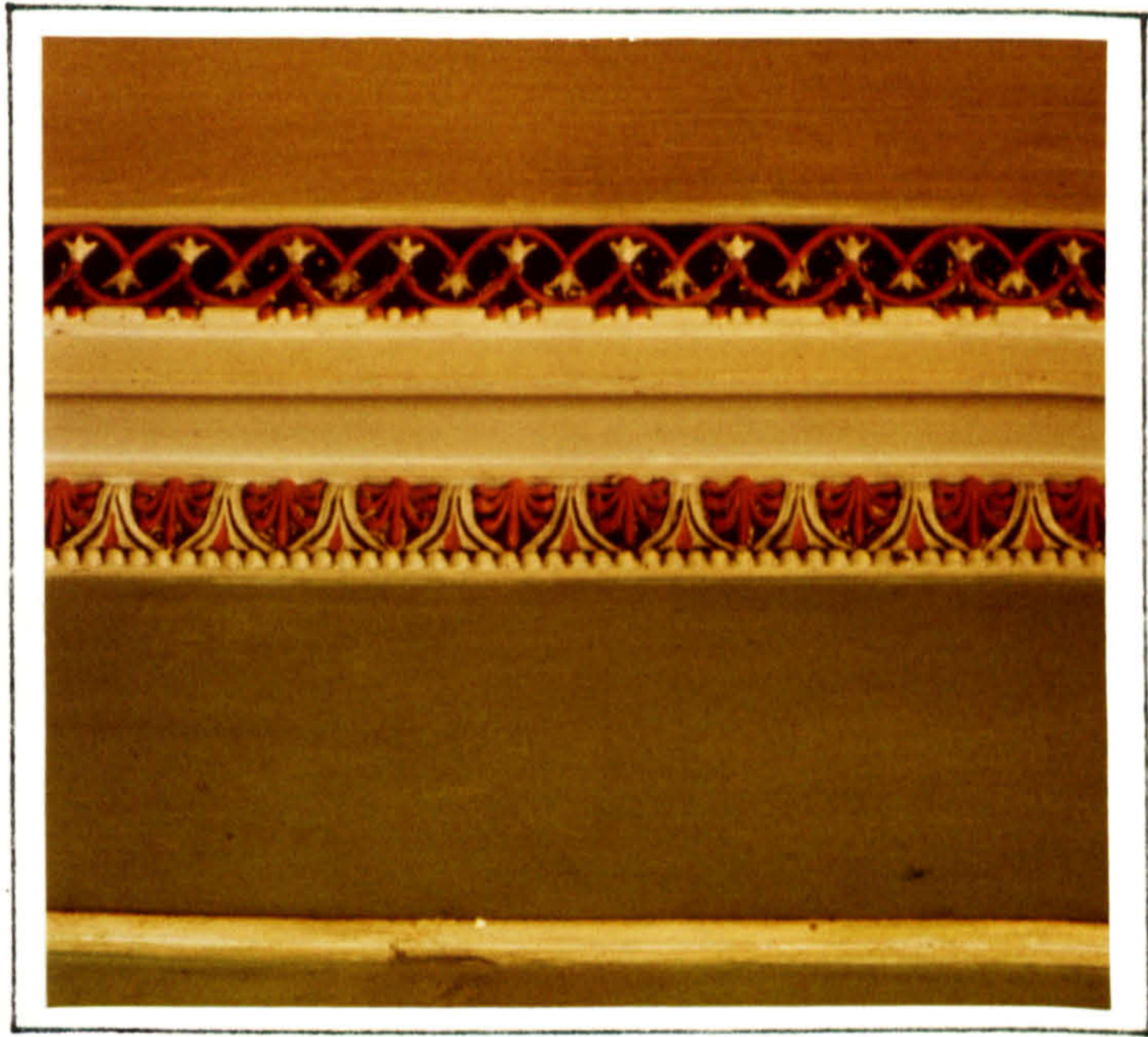
FIG. 132 PICKING-OUT IN 'ETRUSCAN' COLOURS ON THE CORNICE IN THE ETRUSCAN ROOM - HEVENINGHAM HALL
