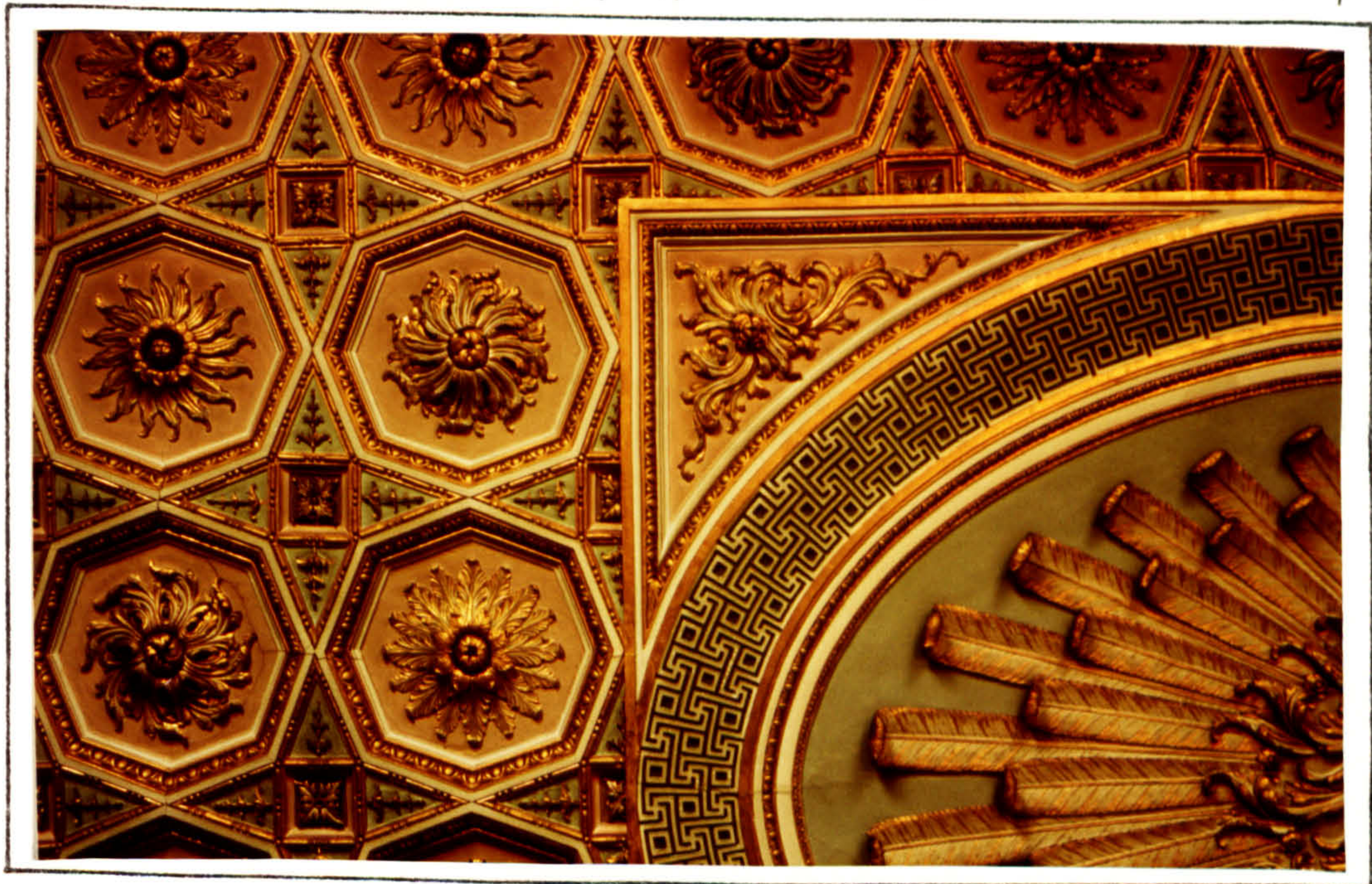
FIG. 142 CEILING OF THE DRAWING ROOM · OSTERLEY PARK
