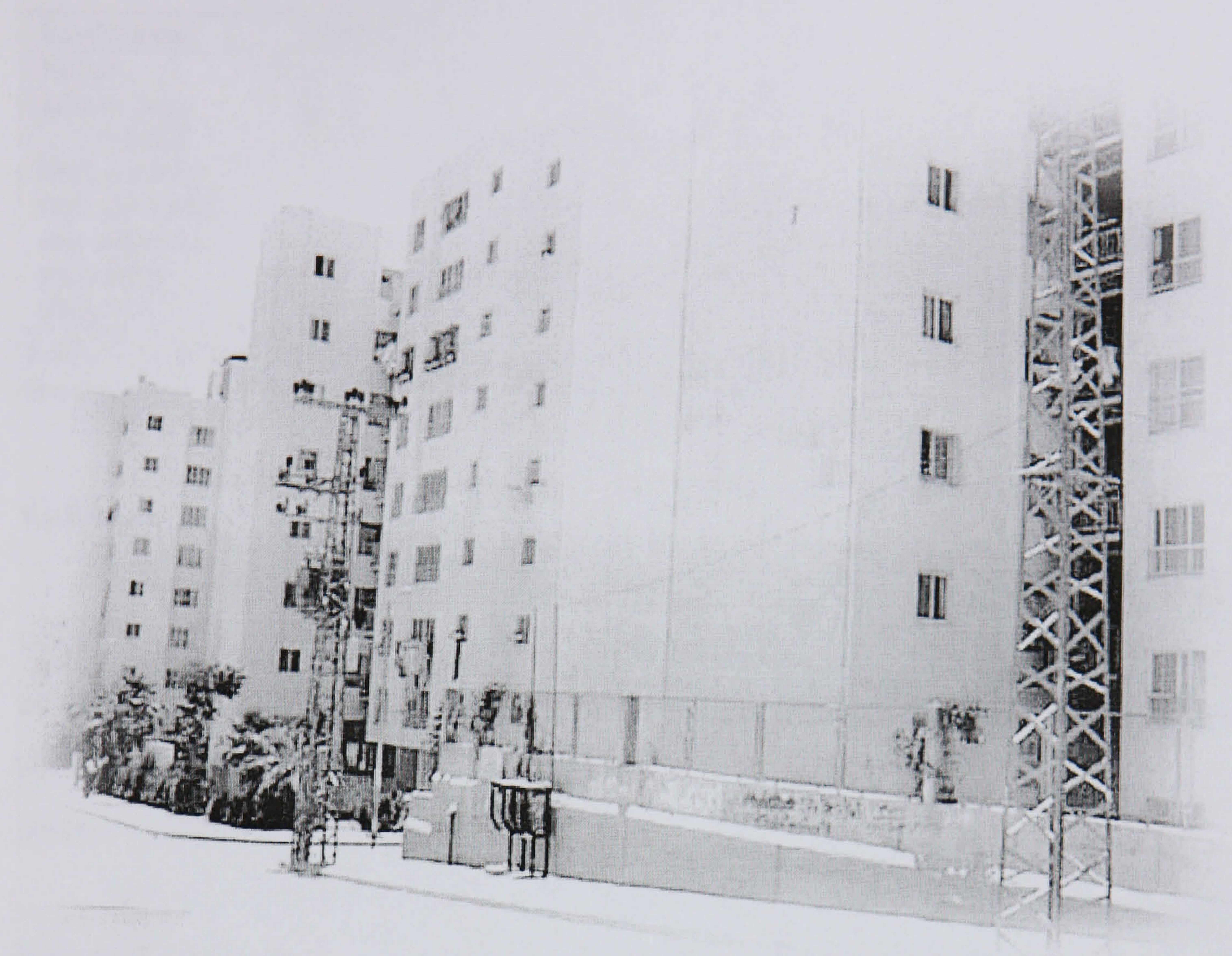
Figure 7.2: A Multi-storey Residential Building, Gaza Strip Source: The Author (May 1996)
