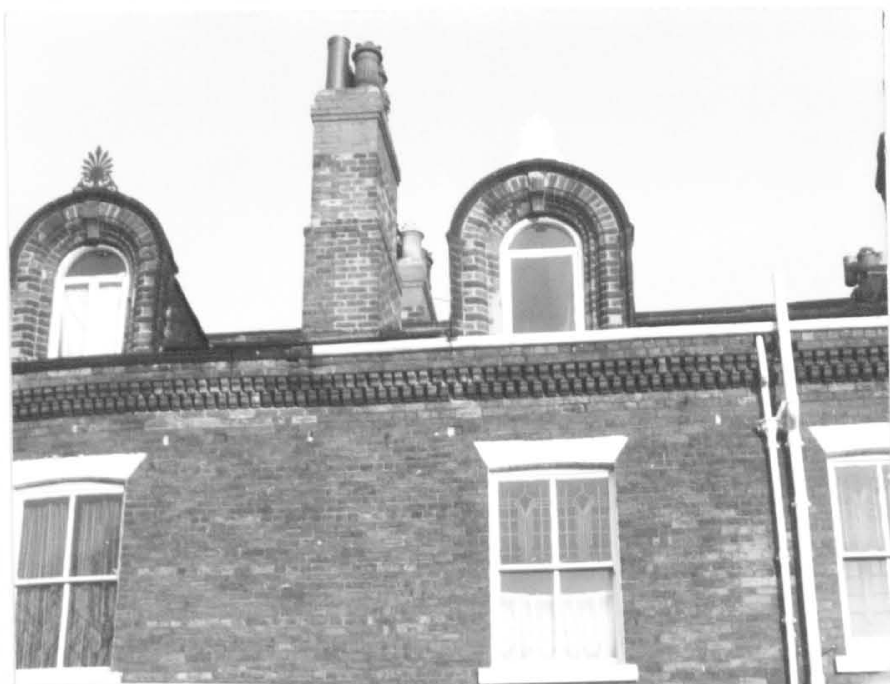
Fig. 166 Eaves detail, Kensington Terrace.
