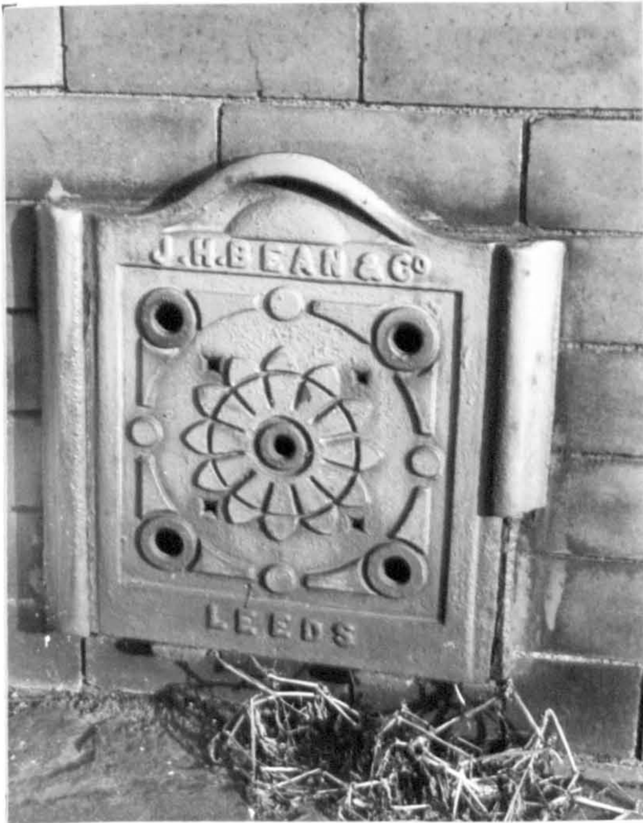
Fig.178 Coal chute cover.
