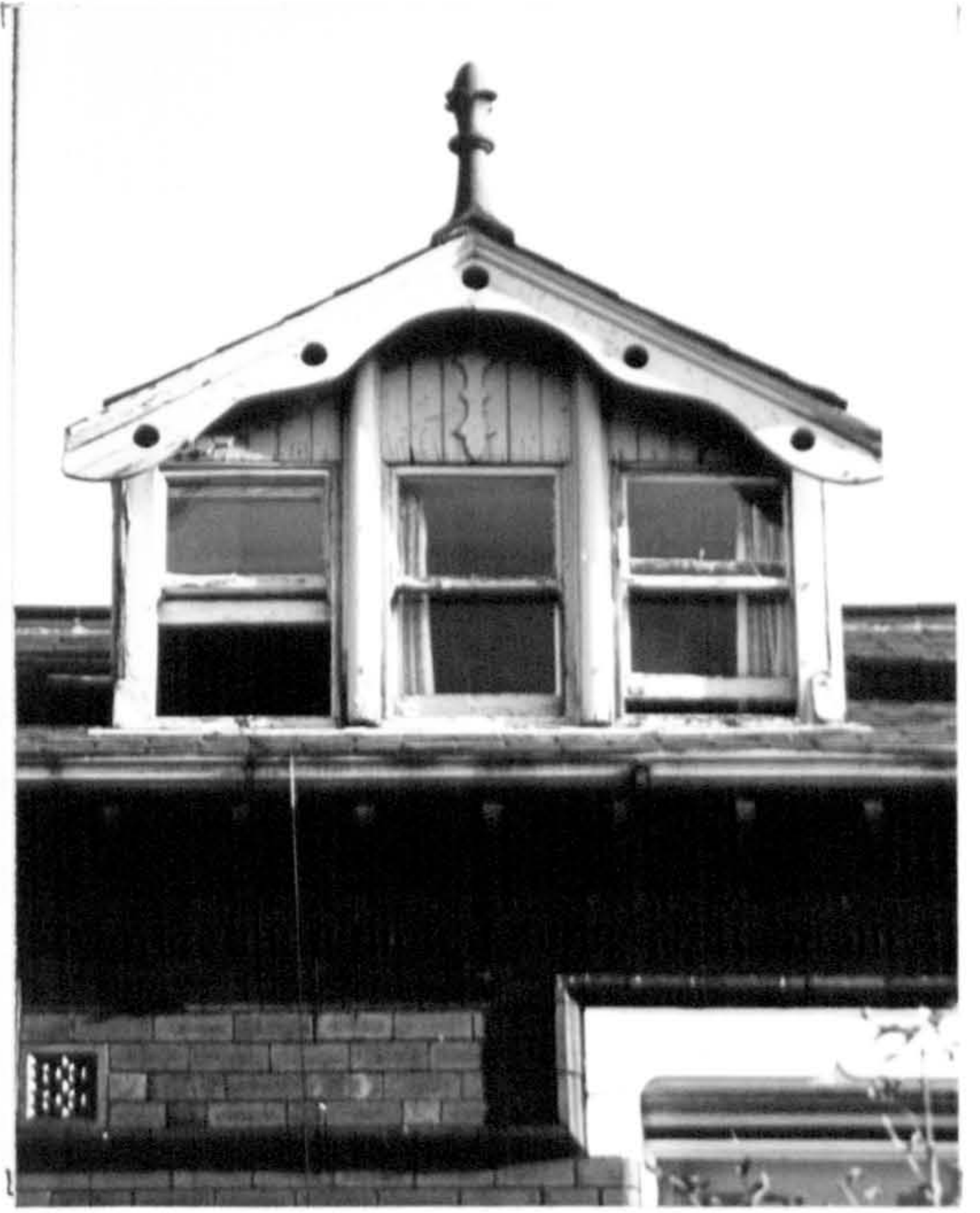
Fig.211 Roof finial on dormer window.
