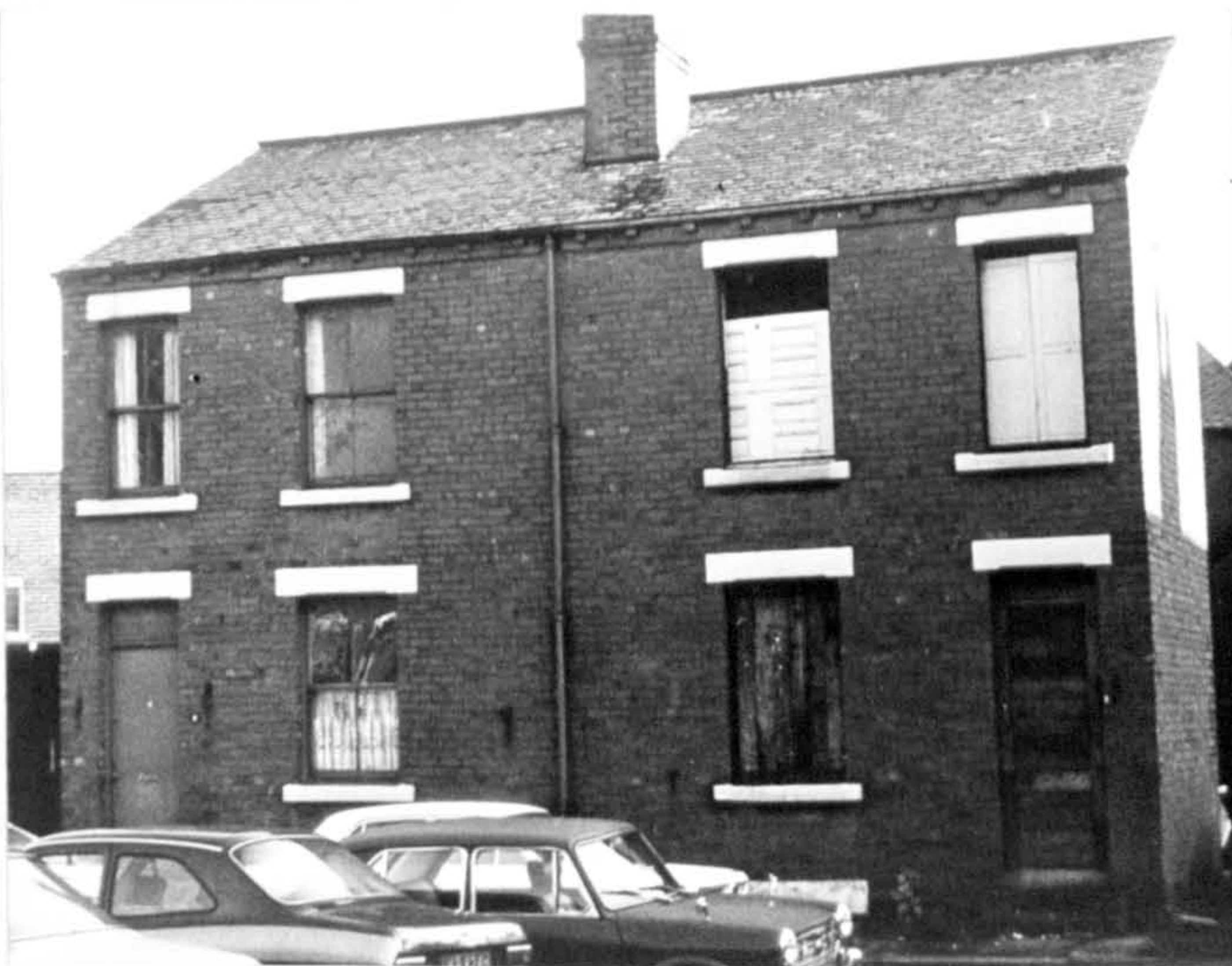
Fig.109 Blind back-to-back houses, Grunberg Grove, taken just prior to demolition.
