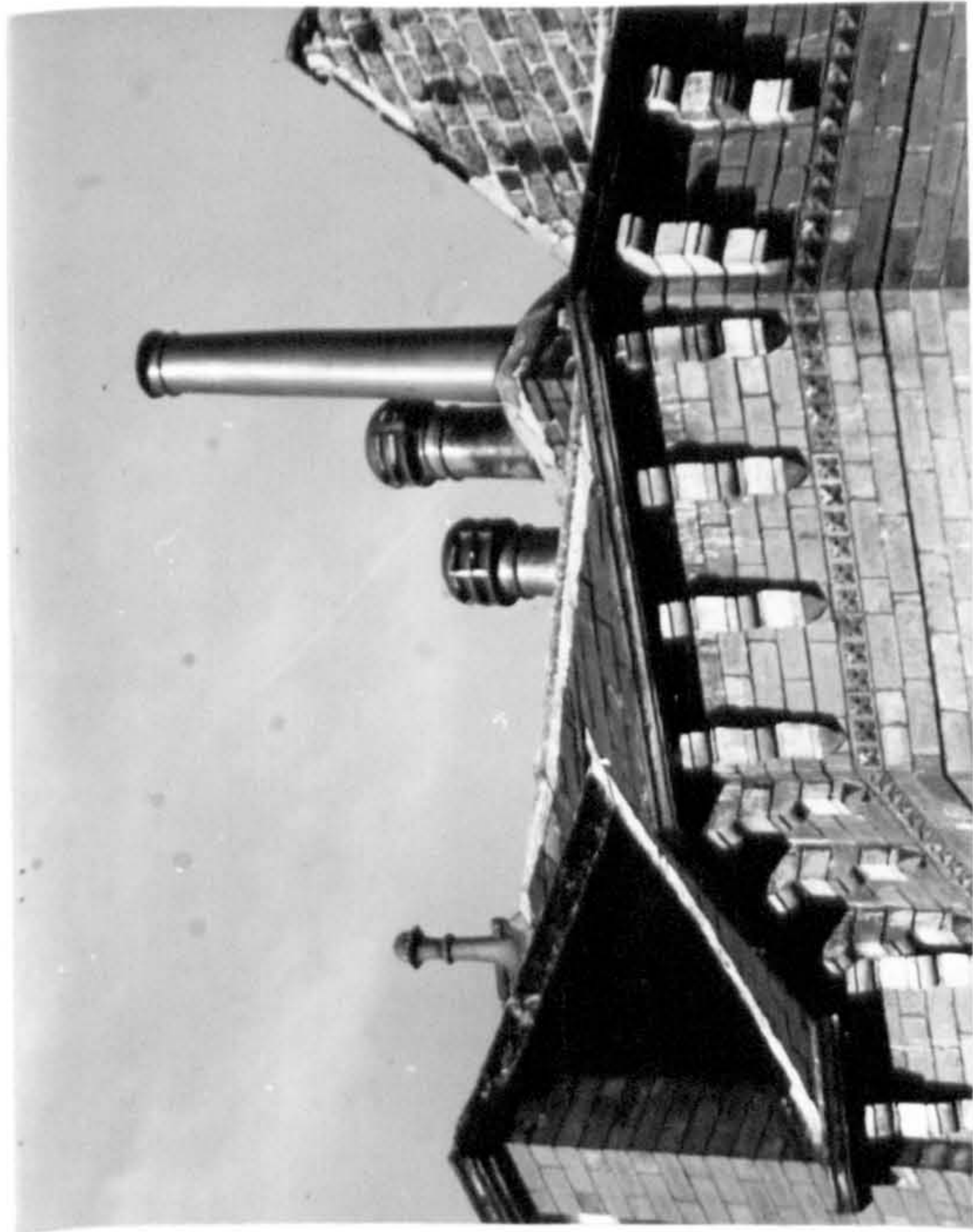
Figs. 206 & 207 Examples of gutter brackets.
