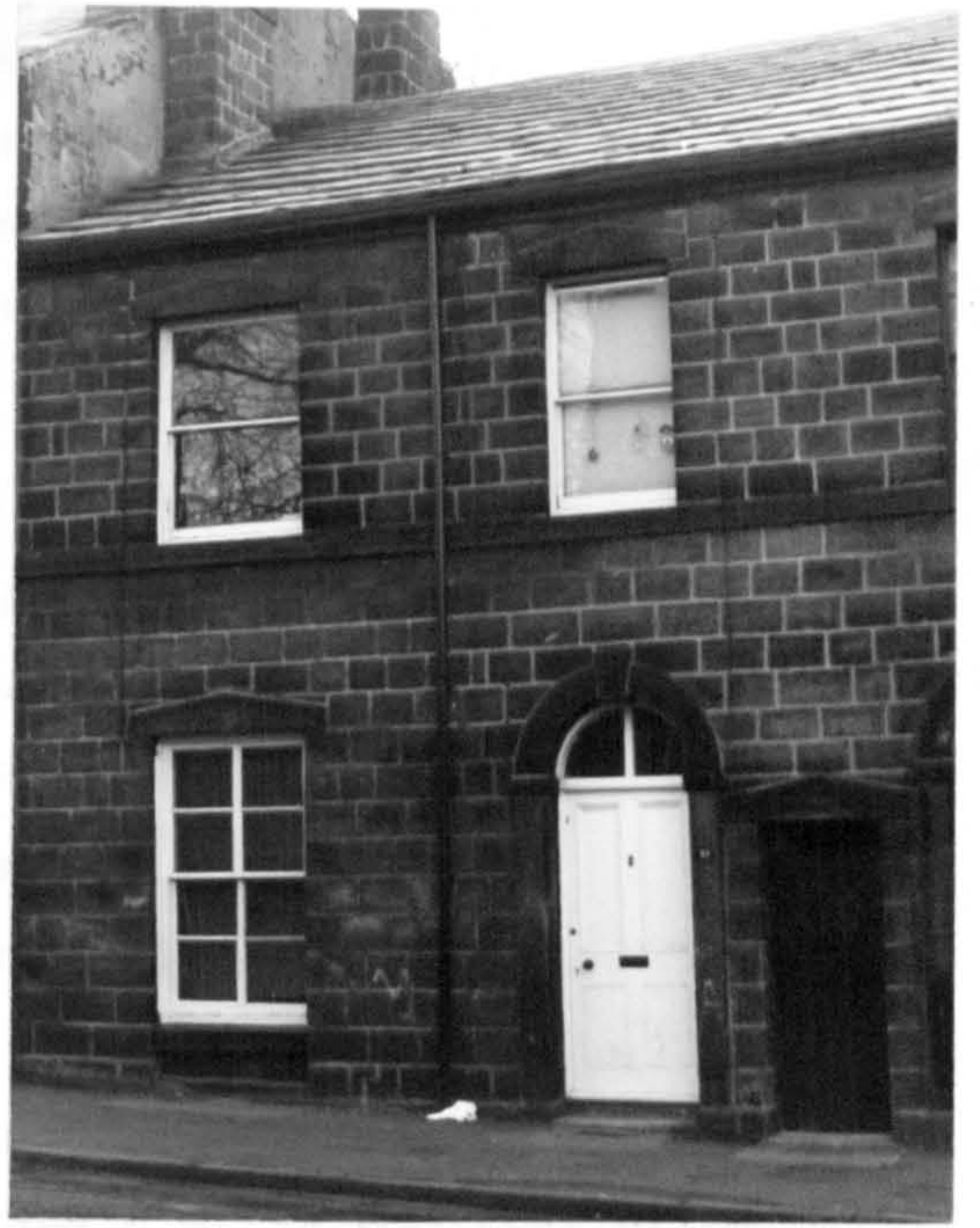
Fig.161 Through terrace, Victoria Road (erected c.1840 - 1860). Note the stone roofing slabs.
