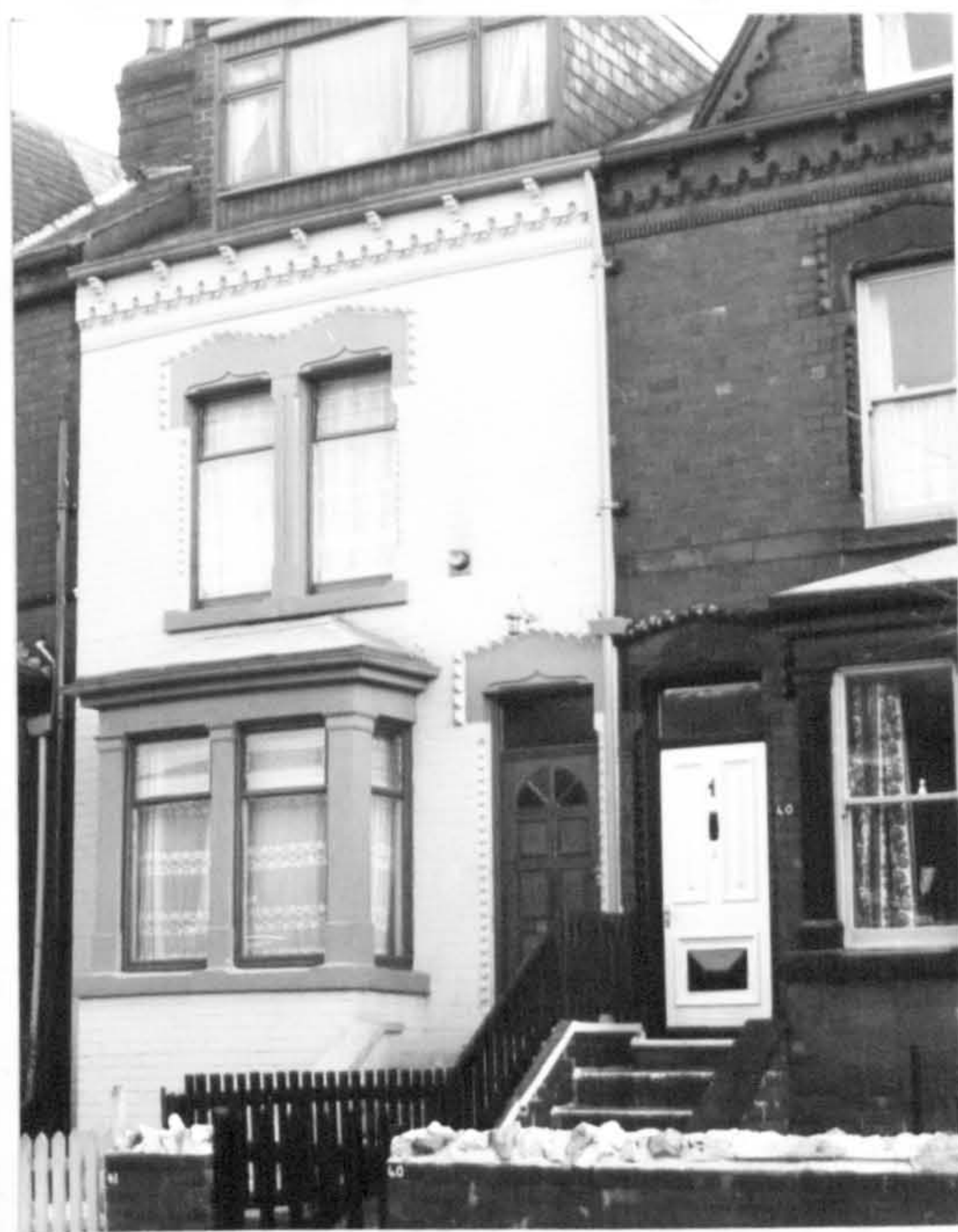
Fig.92 Through houses, Brudenell Mount (Swale & Mitchell 1893) based on an earlier design by J.M. Porter.
