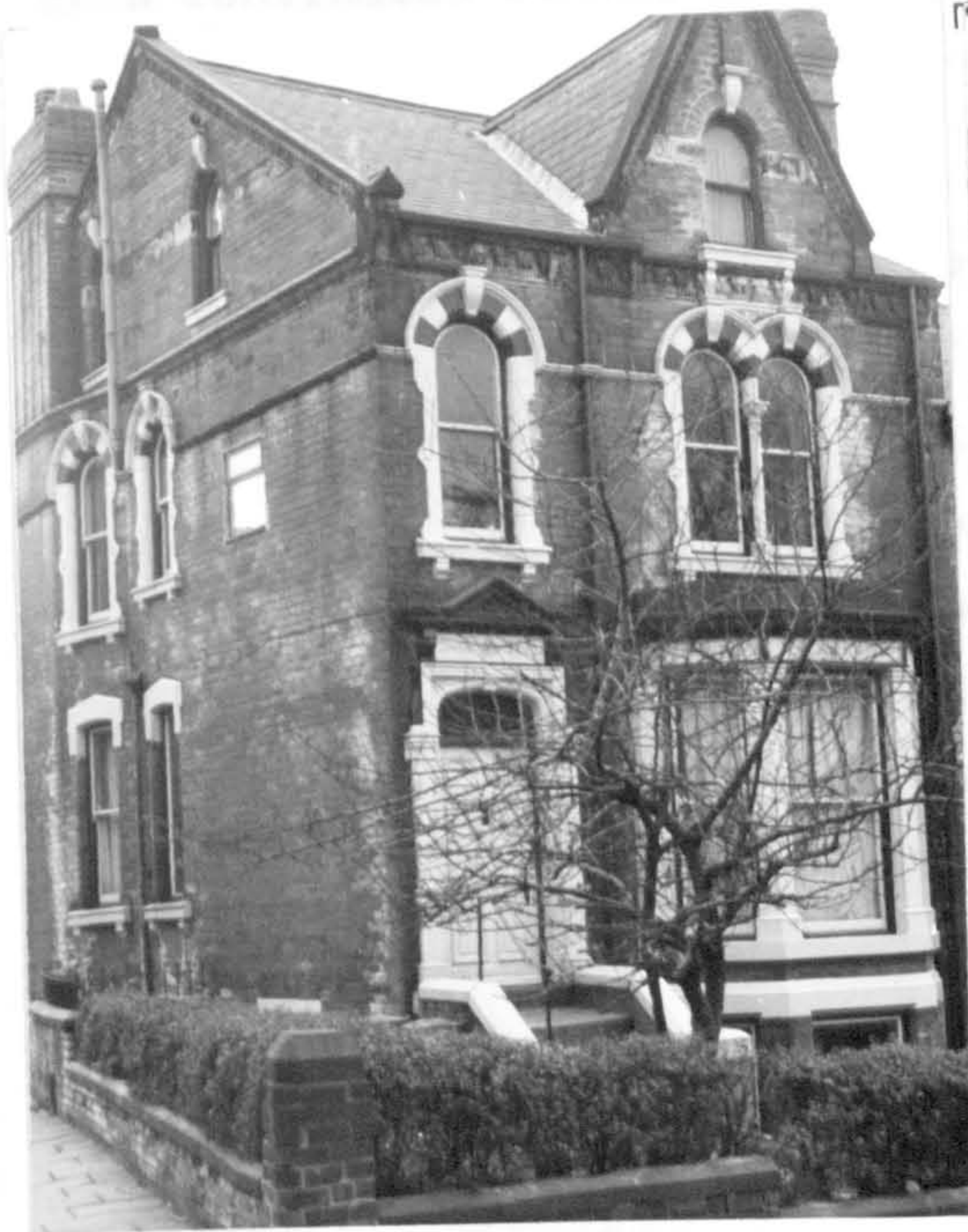
Figs. 204 & 205 Examples of facades incorporating contrasting materials to produce a polychromatic effect.
