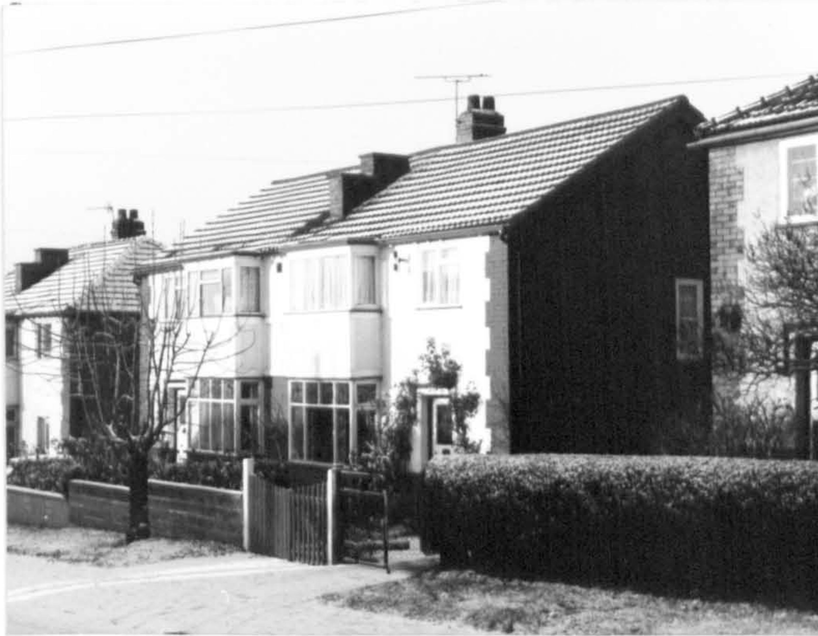
Fig.A64 Inter-war semi-detached houses, Spring Bank Crescent.
