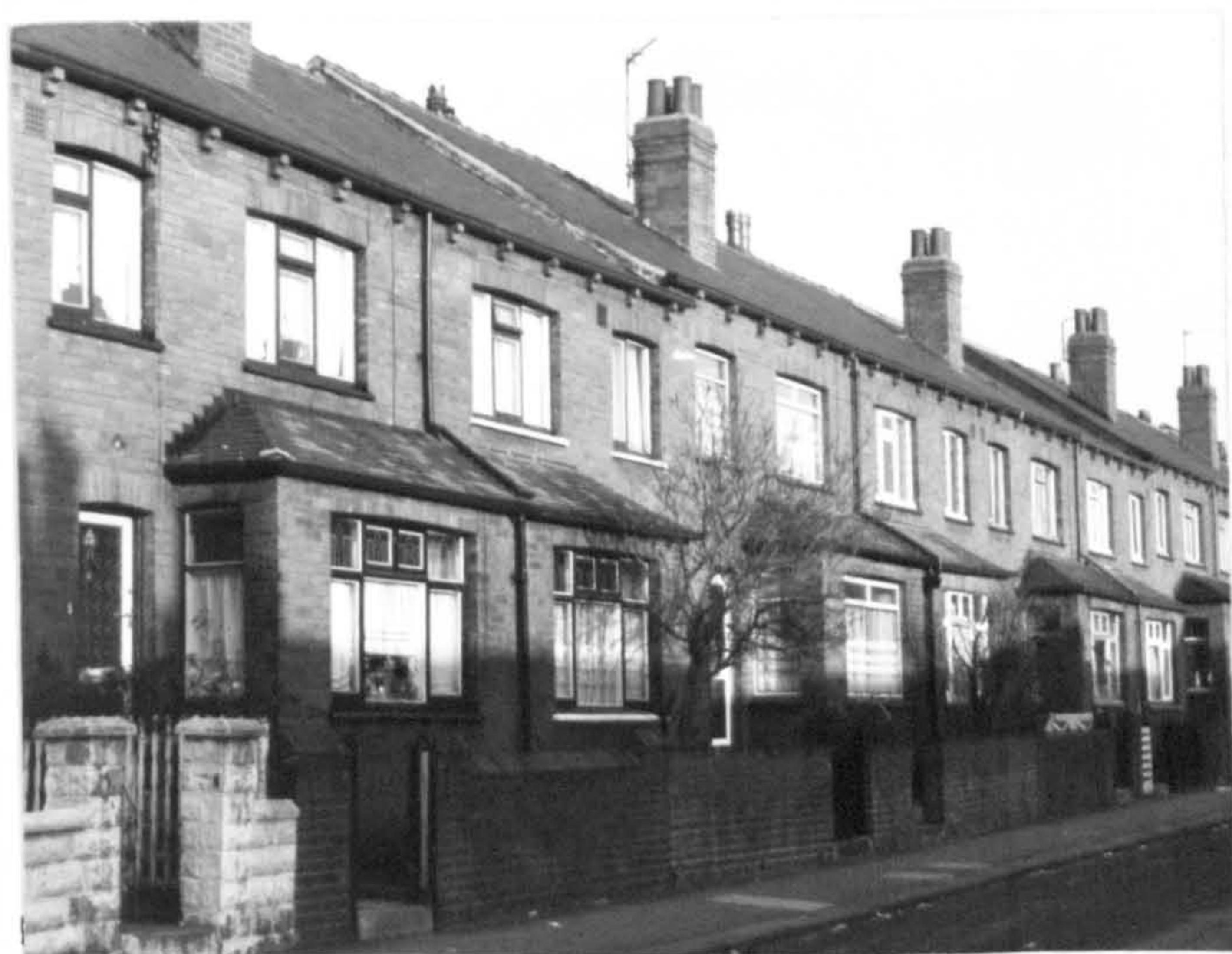
Fig.A62 Through houses built after 1918, Mayville Avenue.
