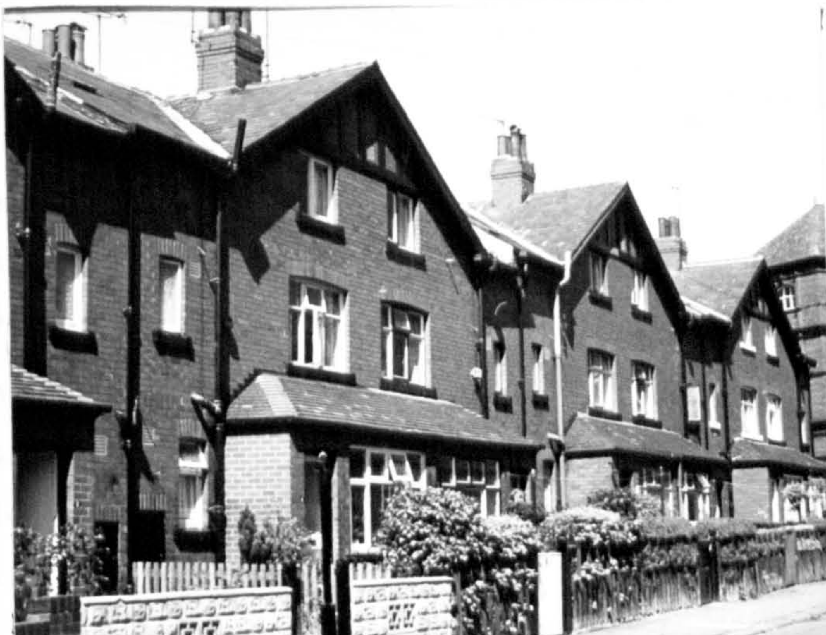
Fig.A63 Back-to-back houses built after 1918, Hessele Road.
