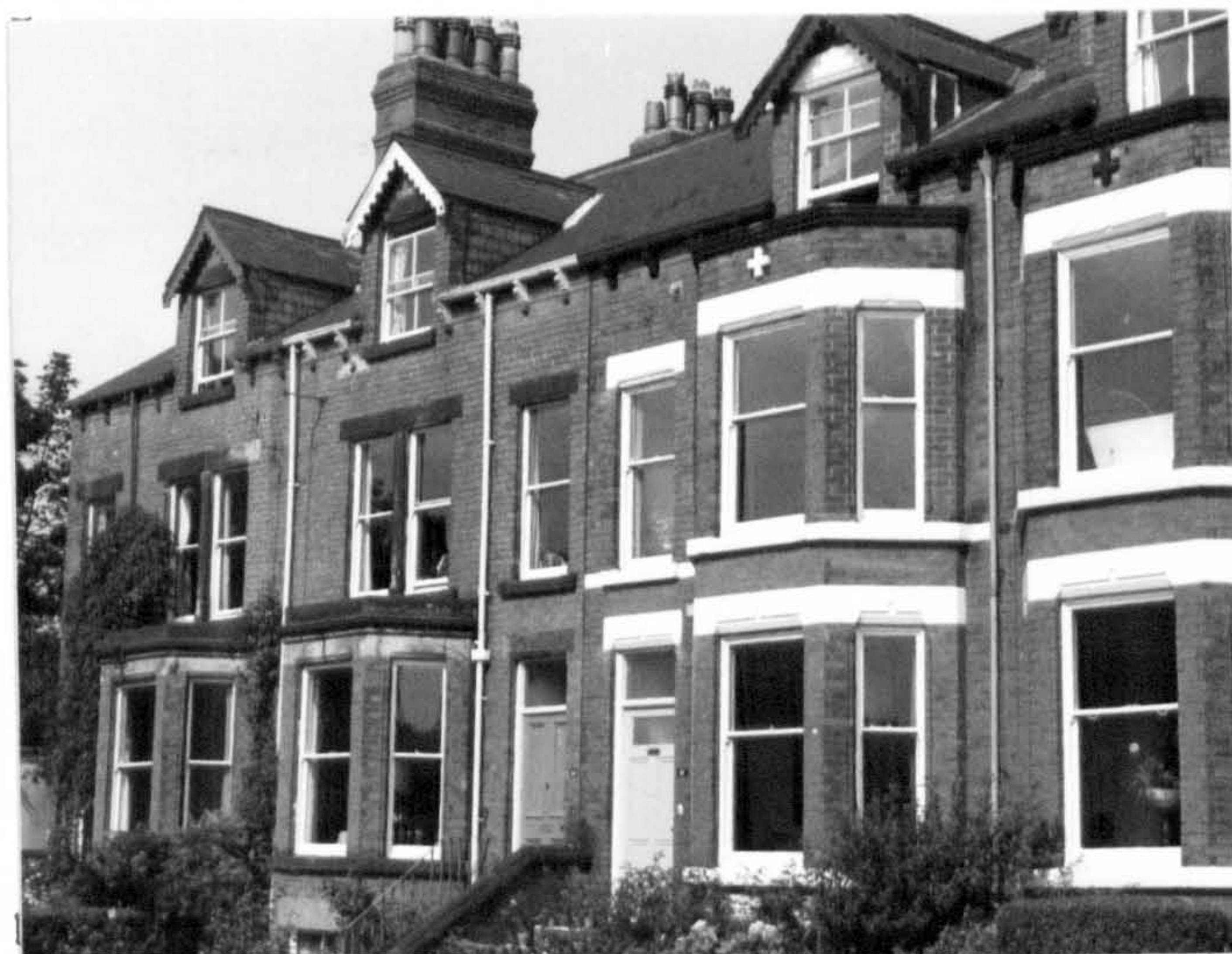
Fig.71 Through houses erected in St. Michael's Road after the introduction of Bye-Laws (G.F. Bowman & E. Wilson 1887 - 1893).
