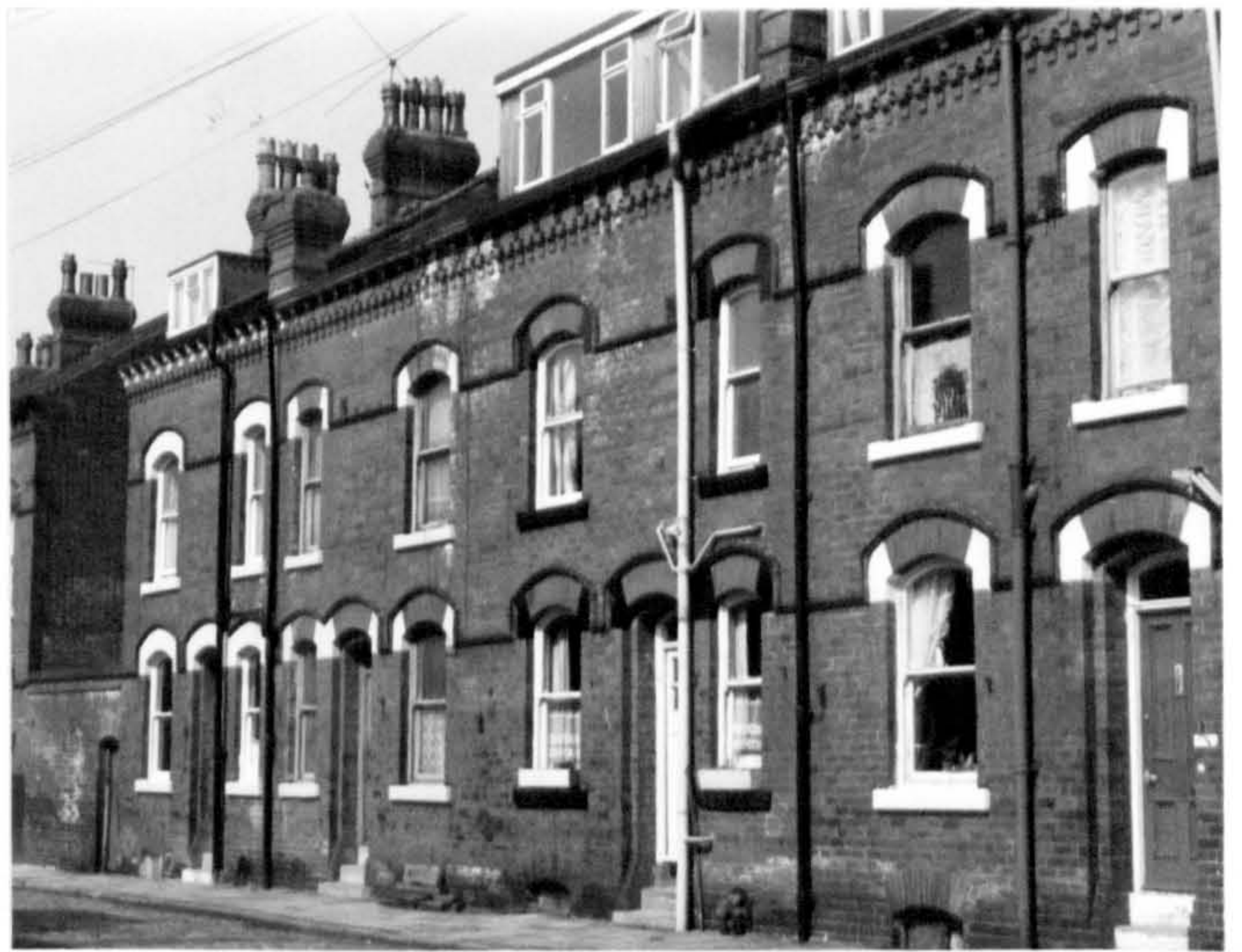
Fig.54 Back-to-back houses, Granby Grove, Headingley village (J. Charles 1886).
