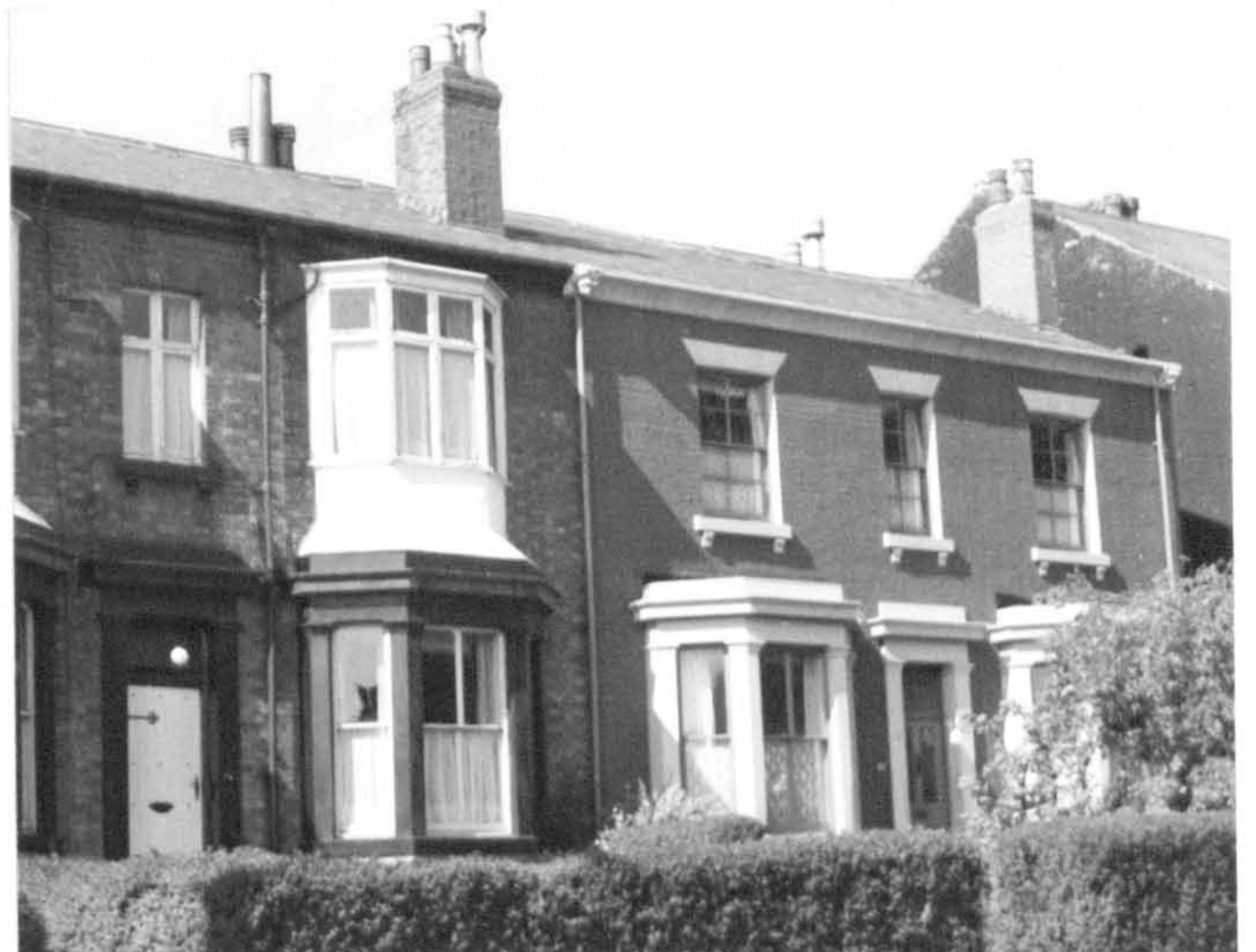
Fig.70 Through houses erected on the Teal Estate prior to the 1870 Bye-Laws.
