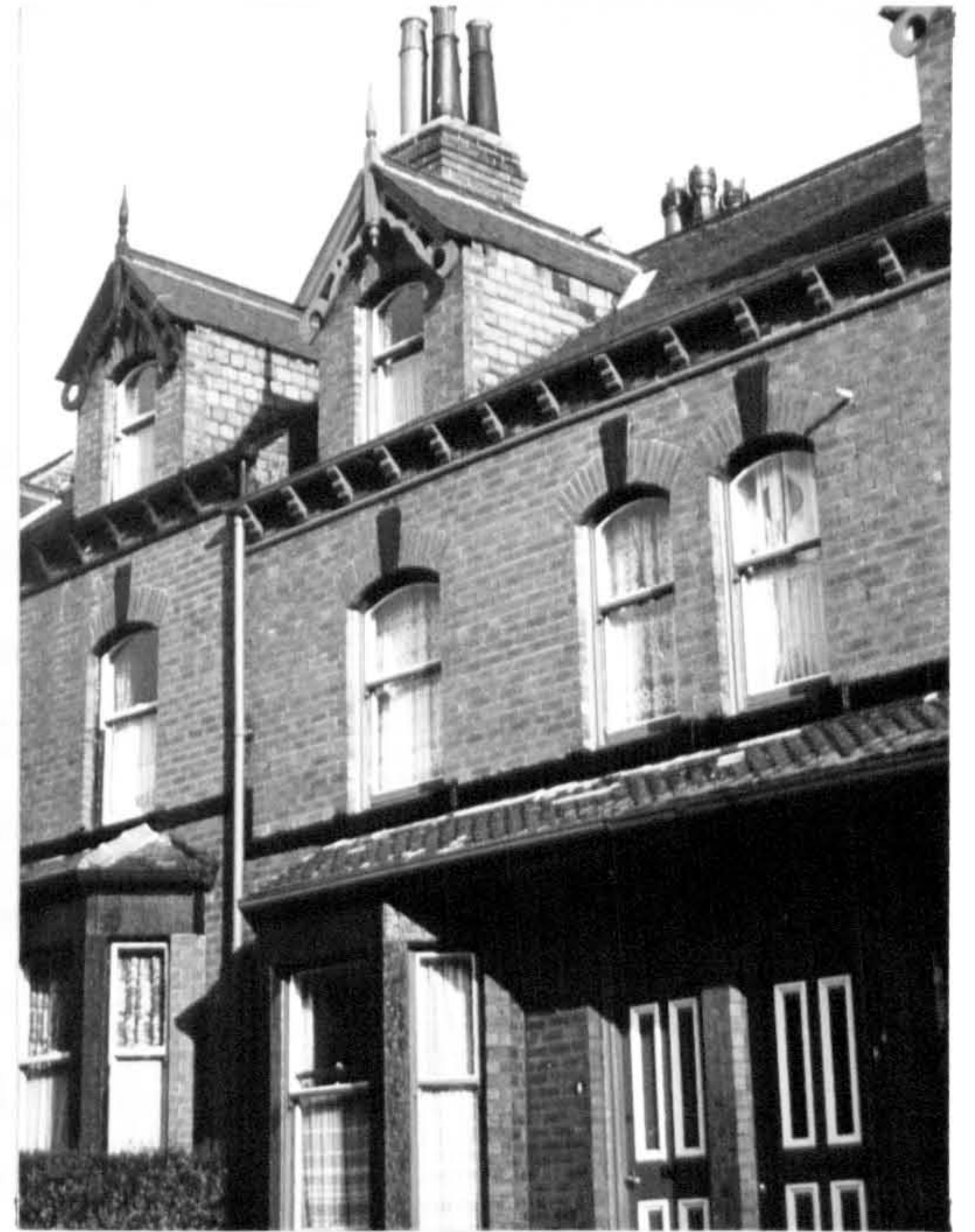
Fig.57 Through houses on the Walmsley Estate, Hessle Place (D. Dodgson 1900).
