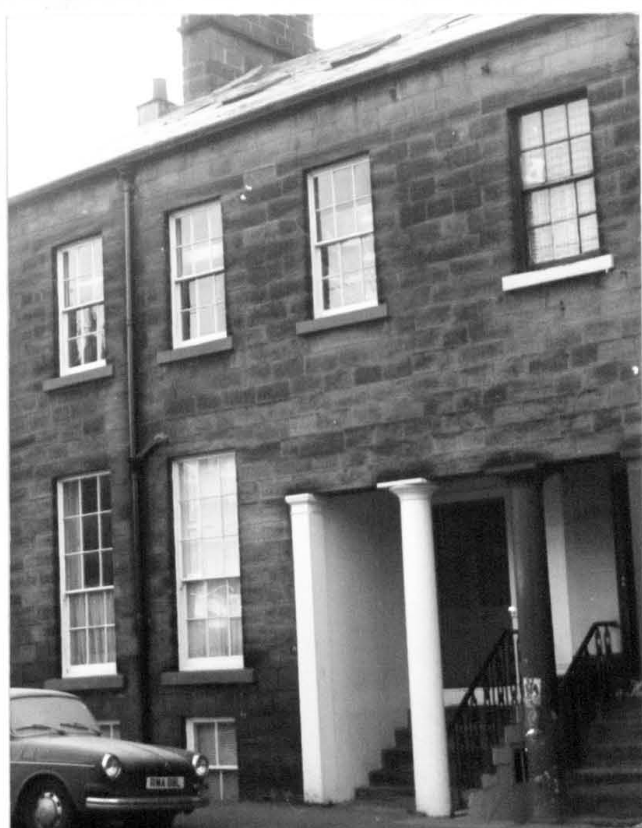
Fig.21 Two houses erected by J. Bulmer in Victoria Road c.1846.
