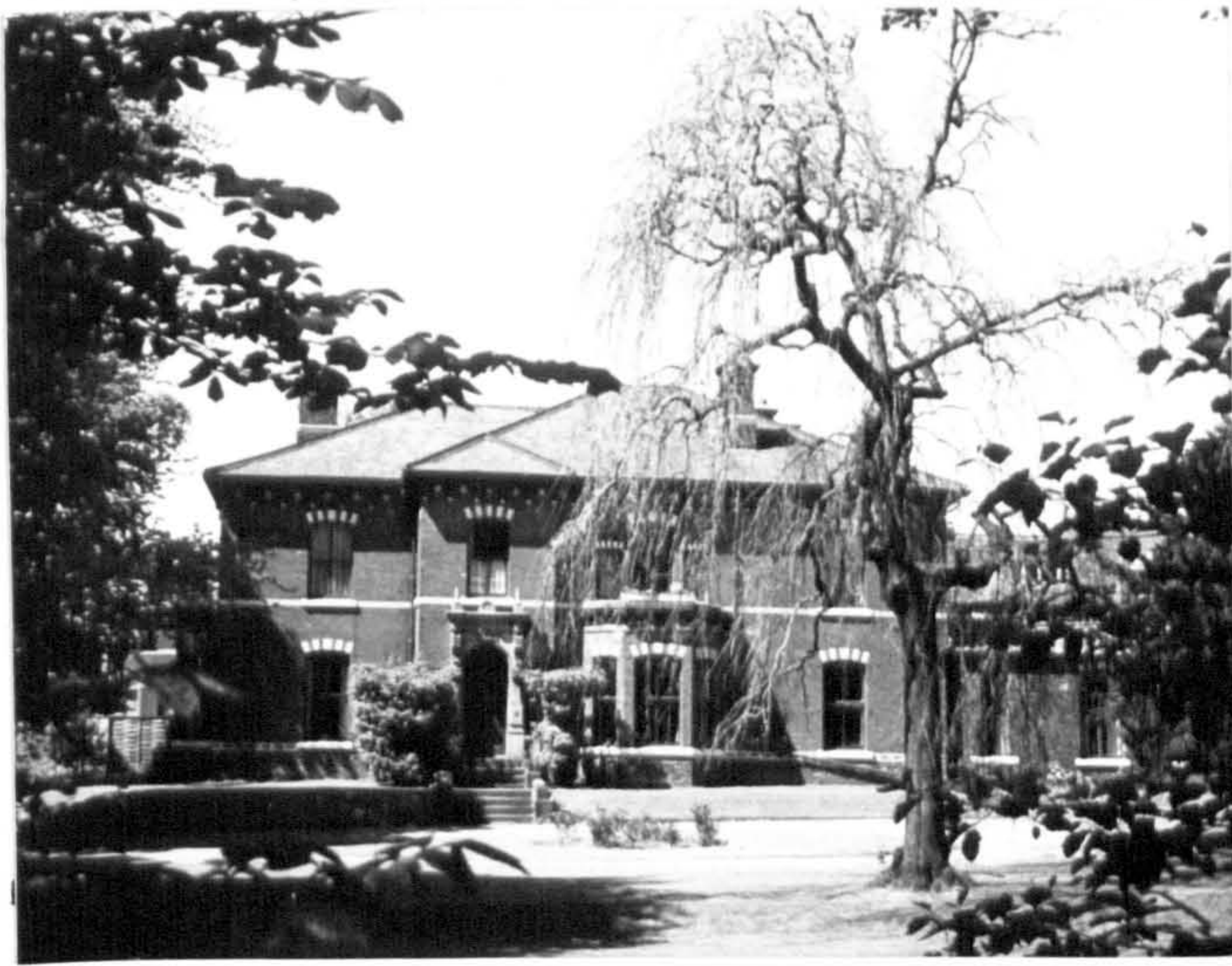
Fig.28 Valley House, Cardigan Road, erected for Jabez Woolley in 1879.
