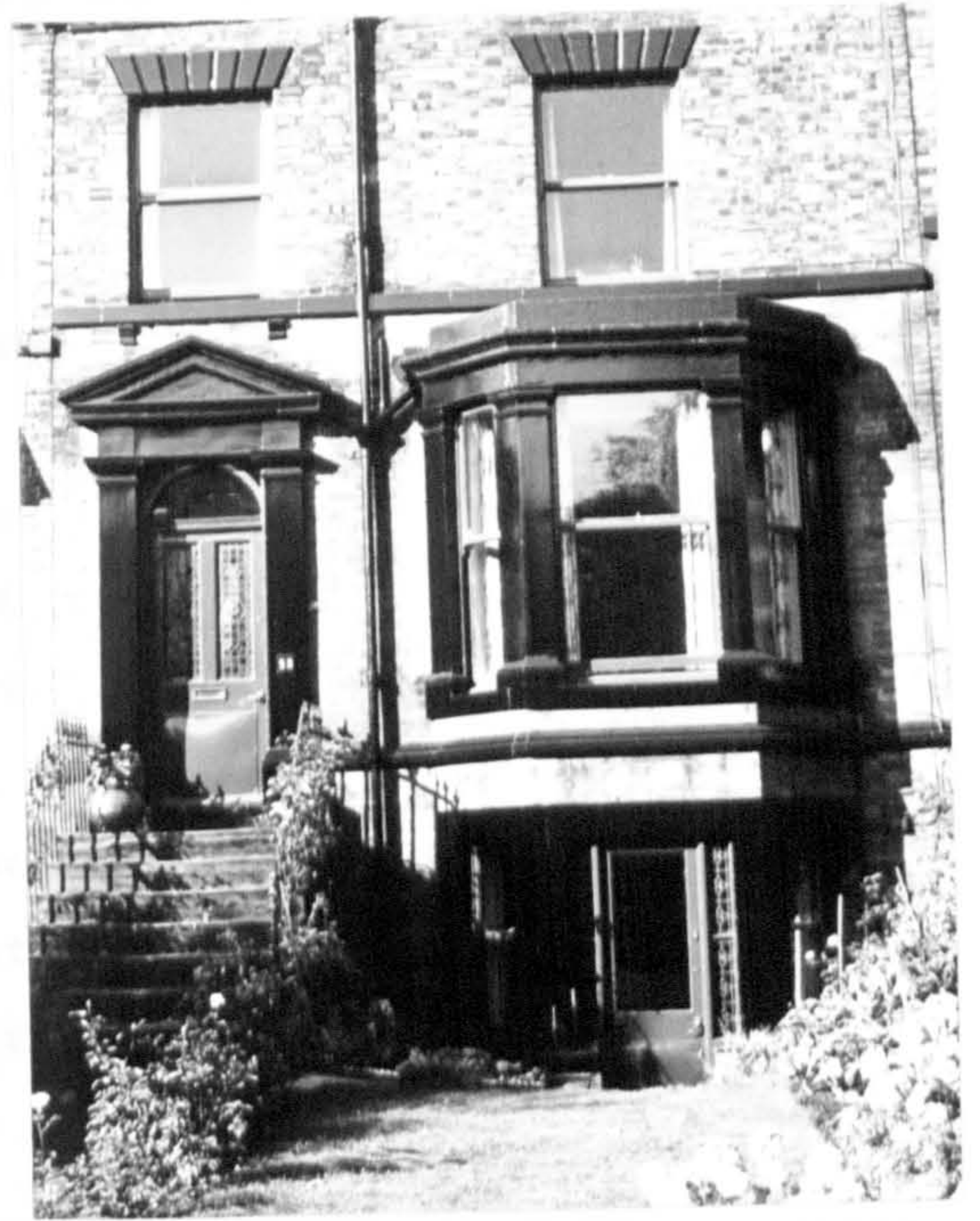
Fig.17 Through house on the Teal Estate, Hyde Park Road, erected c.1862.
