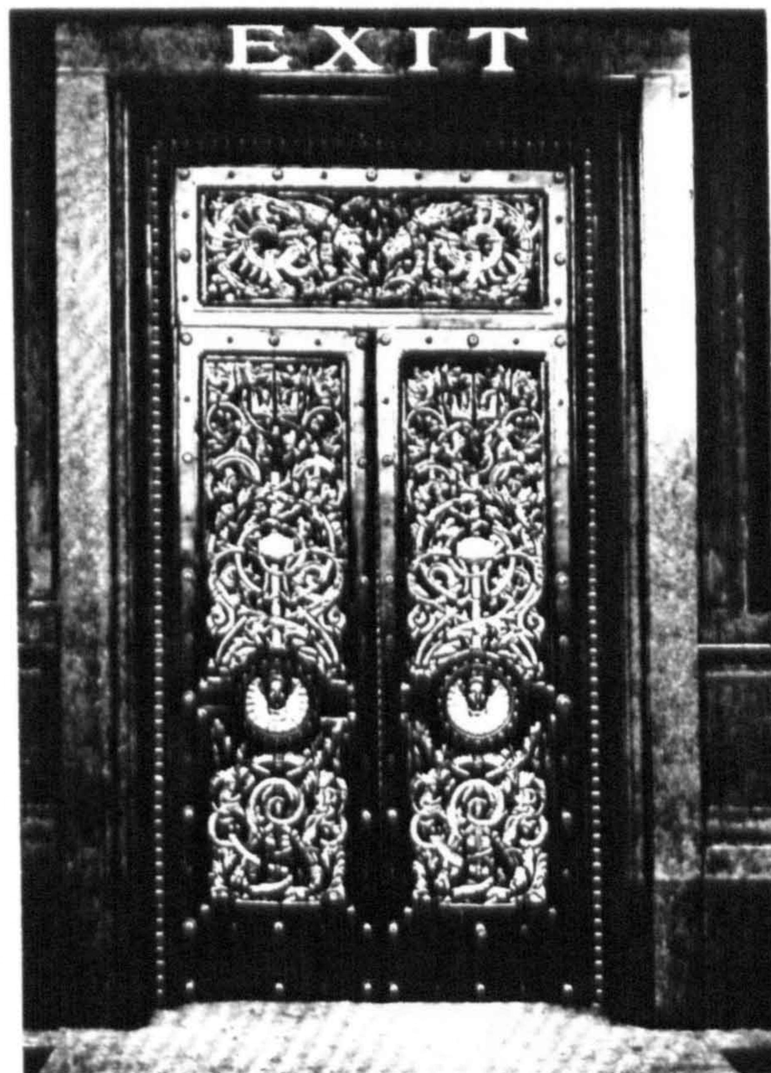
92. One of the doors of St. George's Hall, Liverpool.
