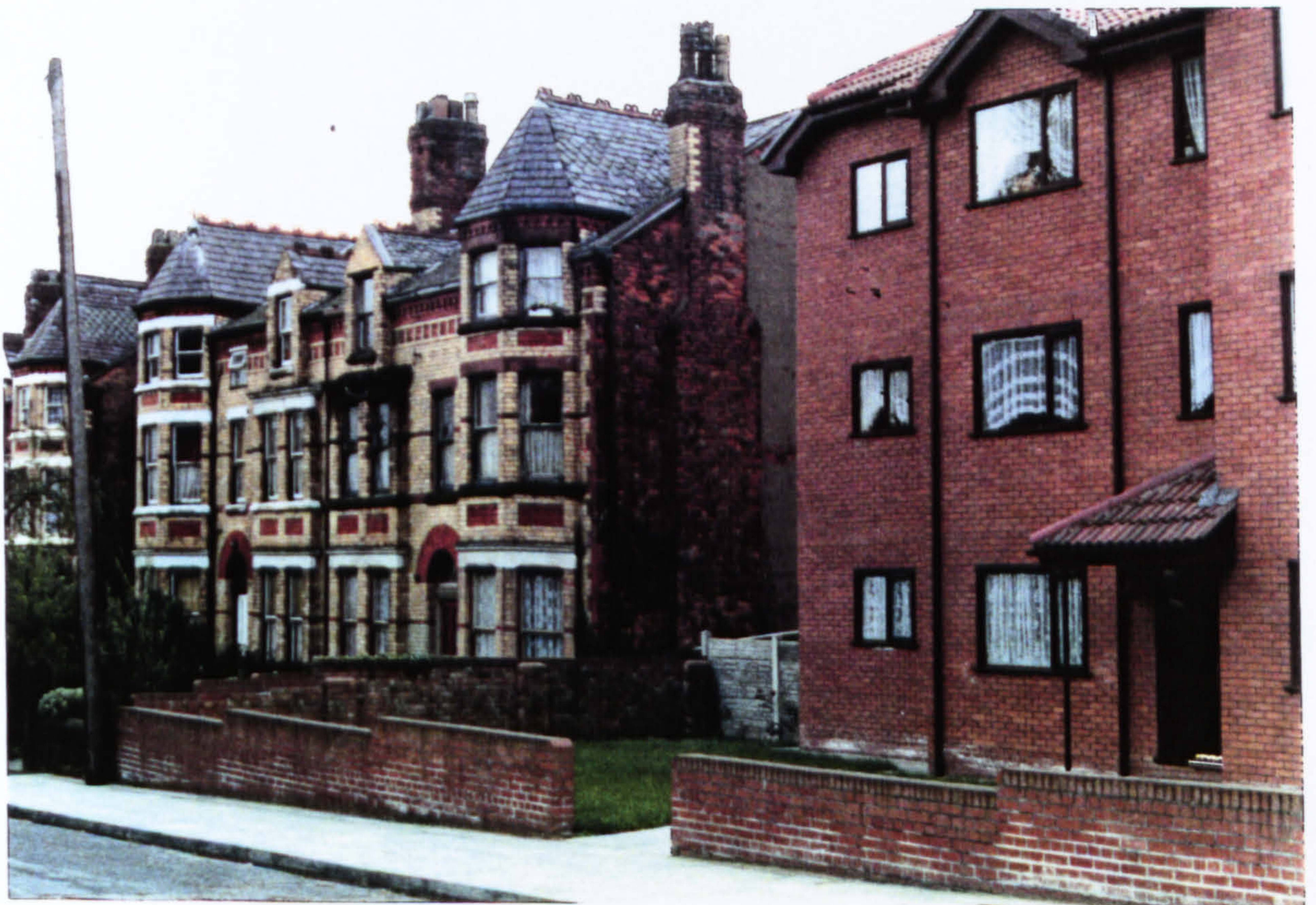
251. The site of 11, Seymour Road, Broad Green, near Liverpool.
