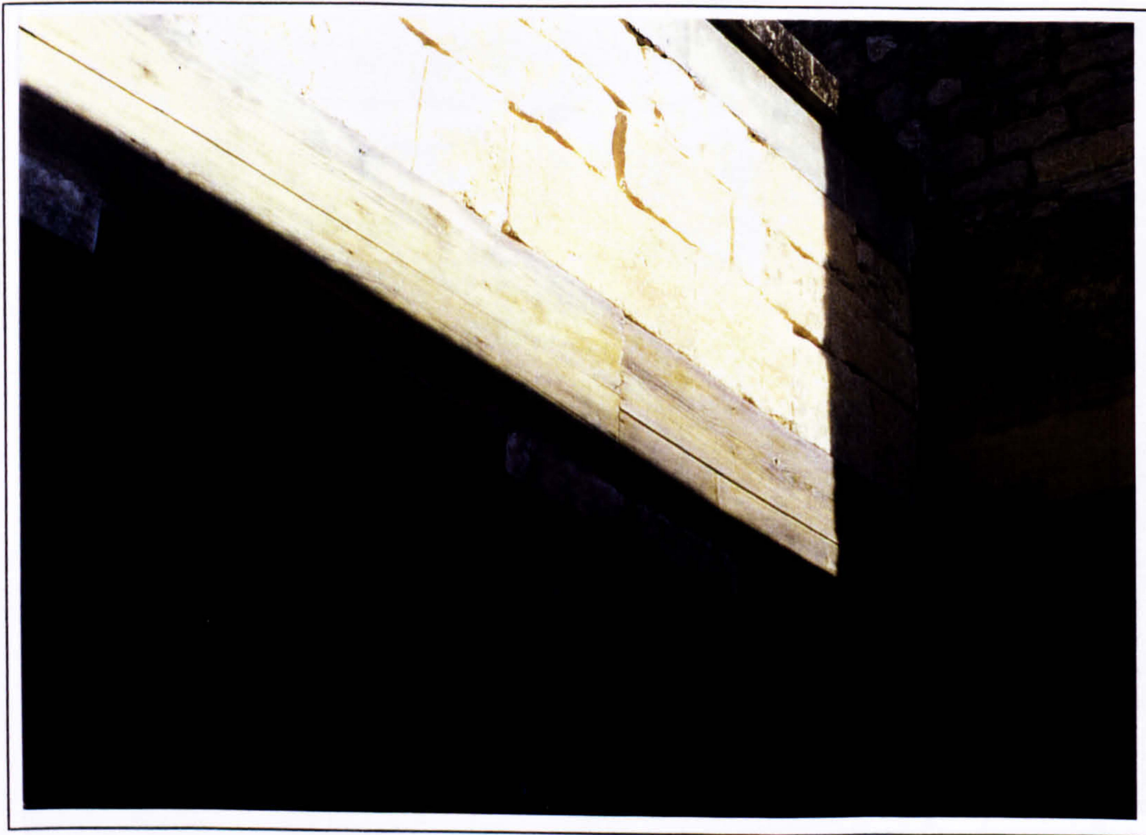
Plate 193 Neglected but still good timber cladding in the light-well of the Queen's Megaron in 1997.
