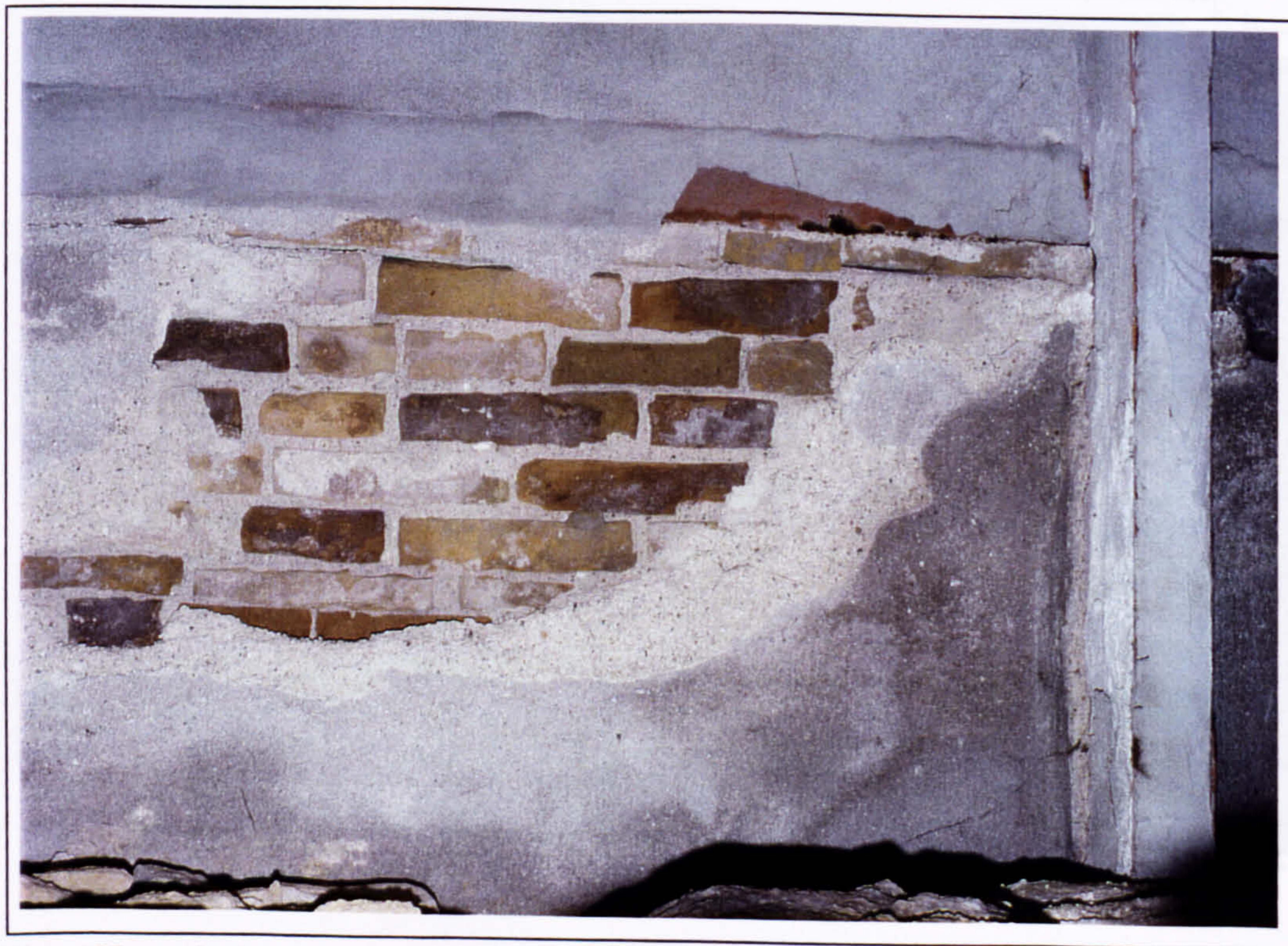
Plate 177 Ceiling of the Corridor of the Painted Pithoi affected by penetrating rain-water.
