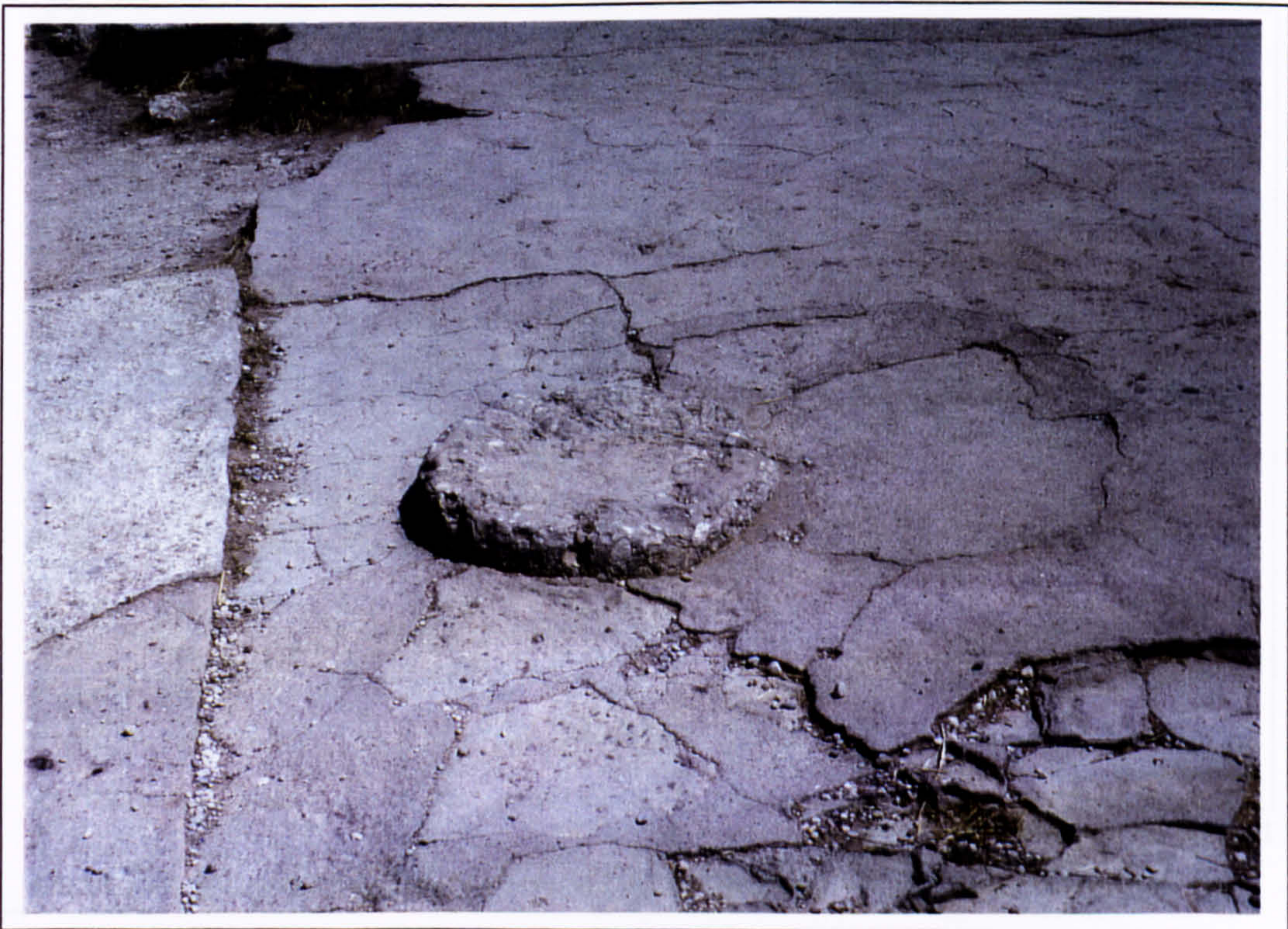
Plate 220 Reconstructed concrete floor and column base at the acropolis of Mycenae.
