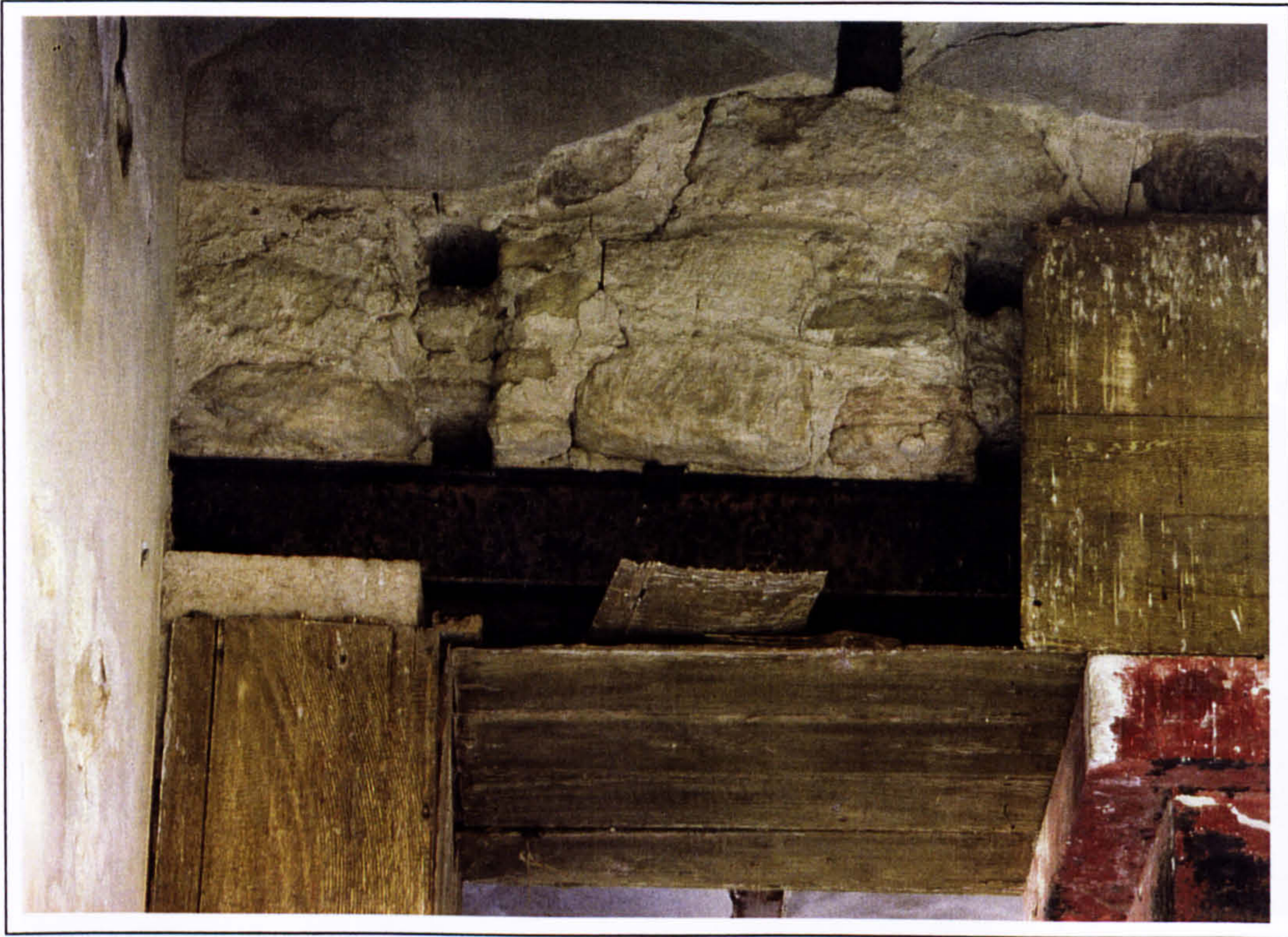
Plate 192 Detail of the lintel construction in the Queen's Megaron in 1997.
