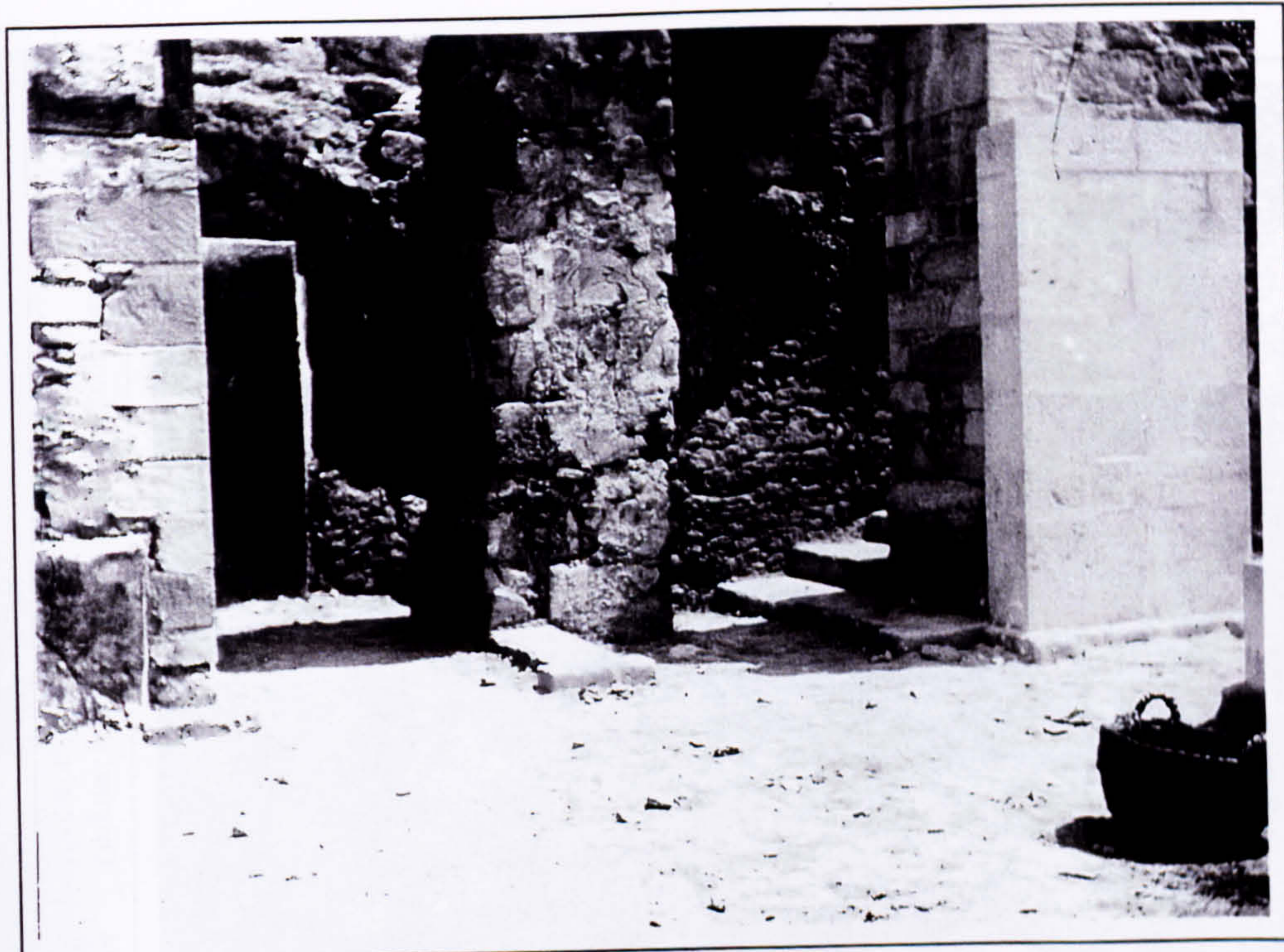
Plate 183 Construction of new door jambs in the Queen's Megaron in 1908.
