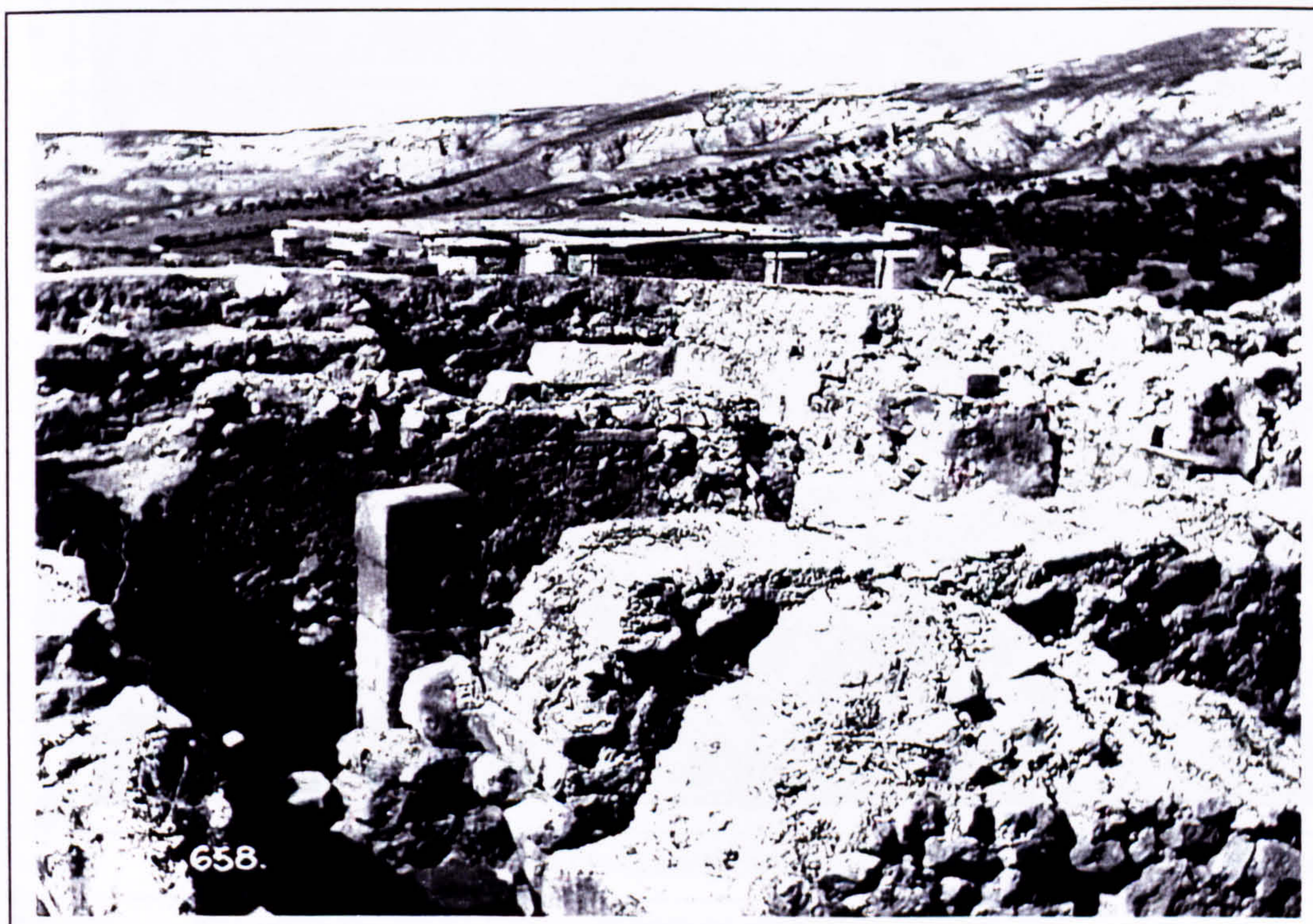
Plate 50 Construction of the flat roof of the Throne Room in 1901. Looking north-east from the south part of the West Wing.
