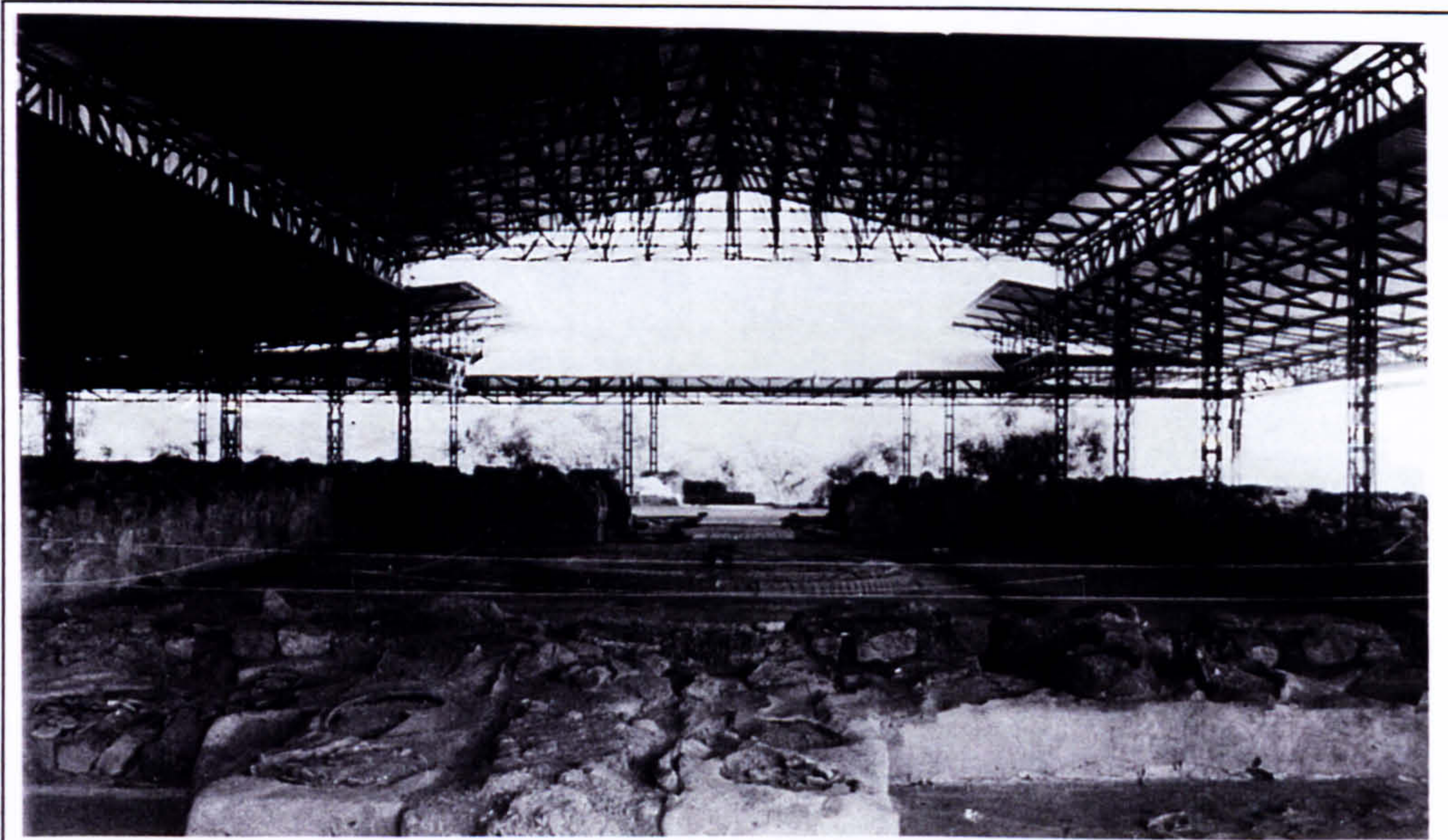
Plate 221 Protection roof above the excavation site of the Palace of Nestor at Pylos.
