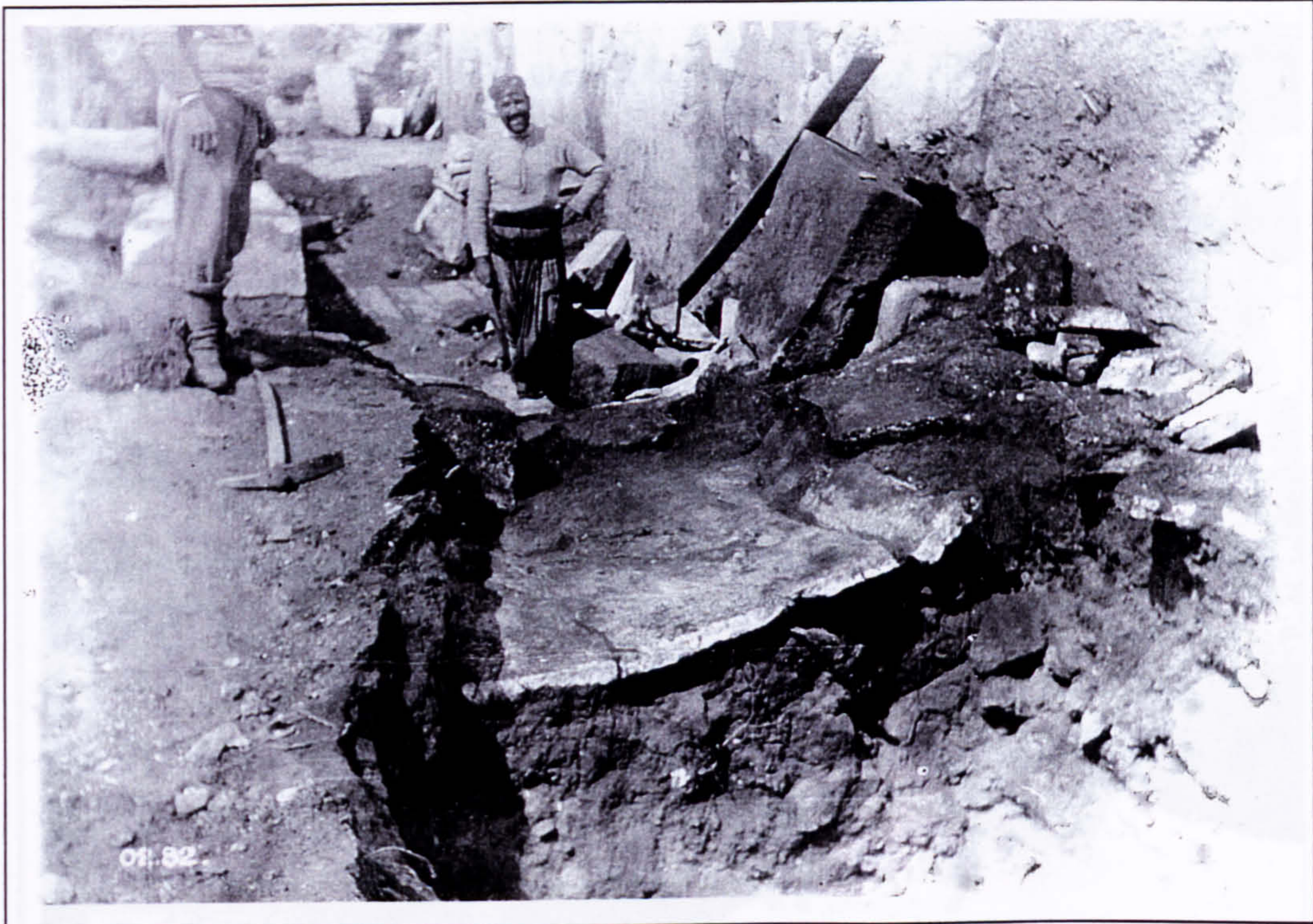
Plate 93 Excavation work at the upper East-West Corridor in 1901 looking west.
