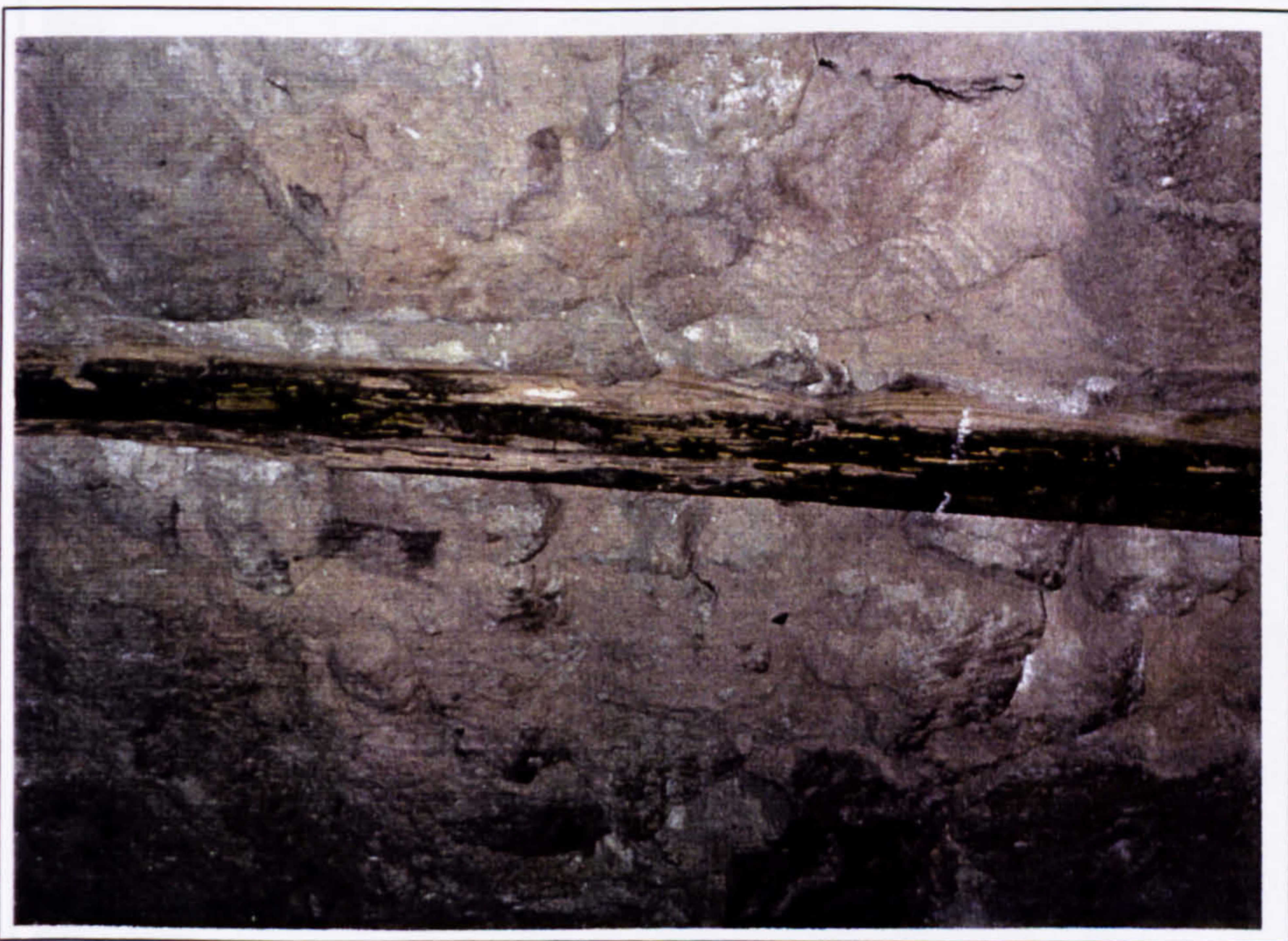
Plate 174 Fir post of Fyfe's 1902 reconstruction work in the Treasury in 1997.
