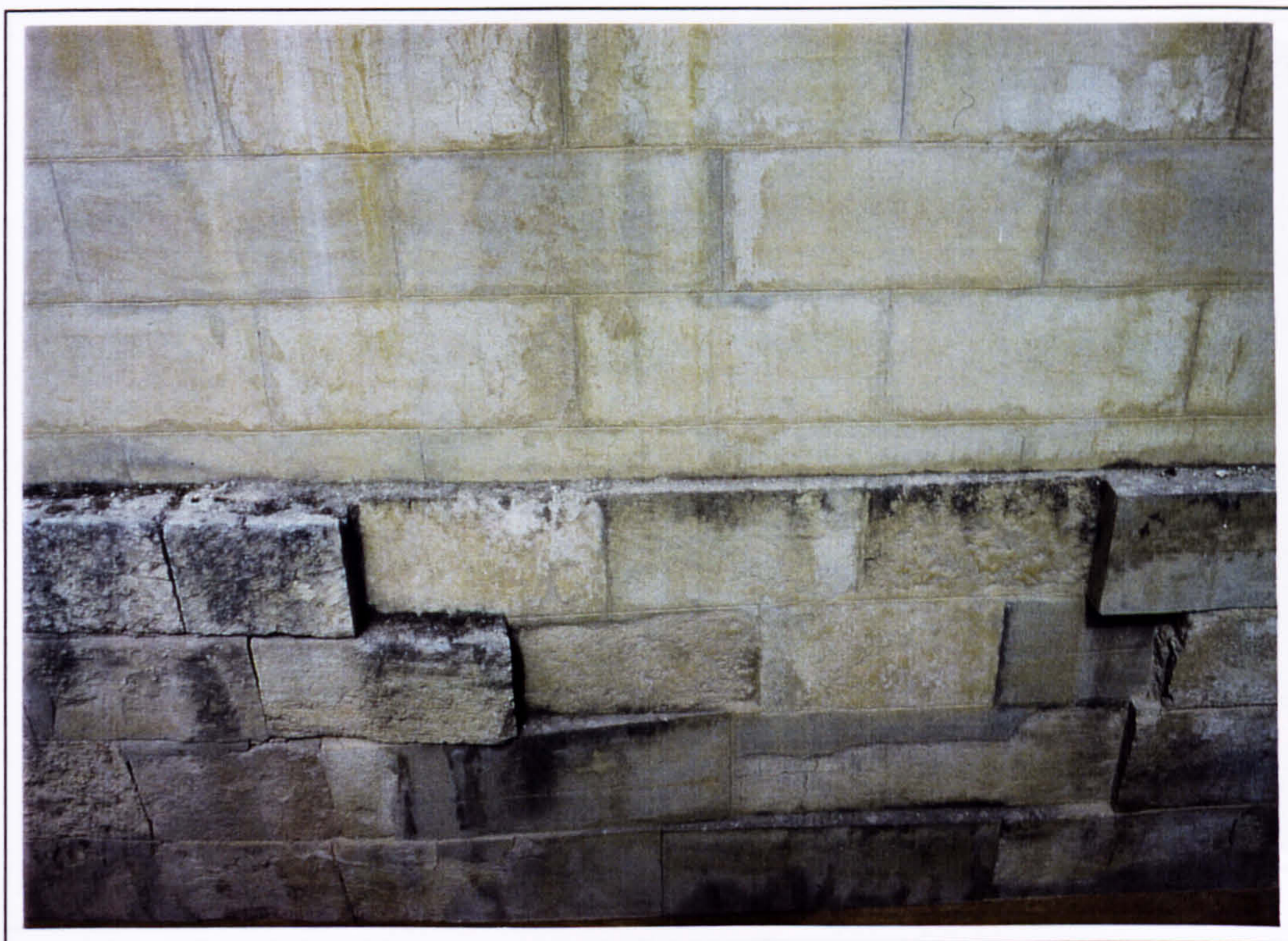
Plate 154 Reconstructed west wall of the light-well of the Hall of the Double Axes in 1997. The lower, projecting stones are the original wall.
