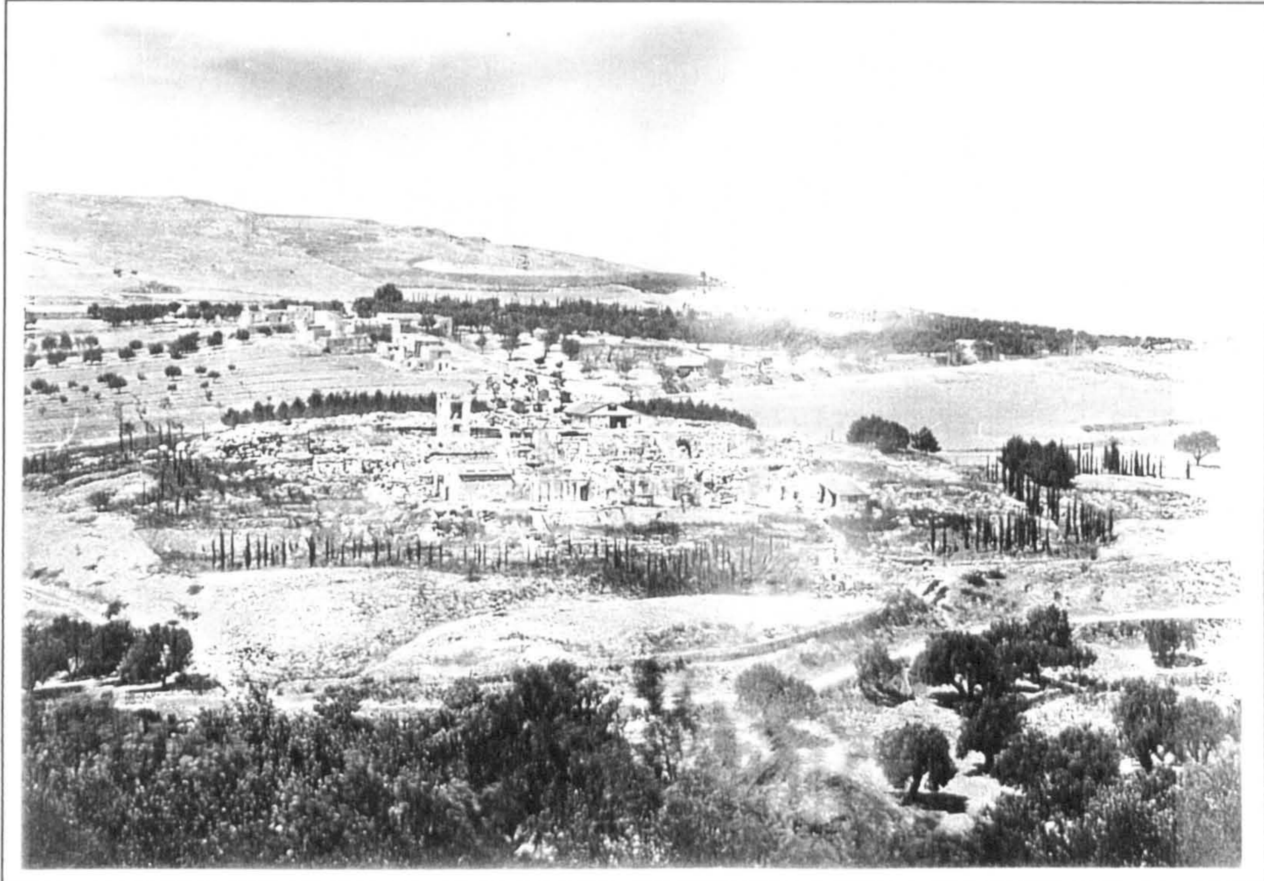
Plate 5 General view of the excavations of the palace, 1922 (?)
