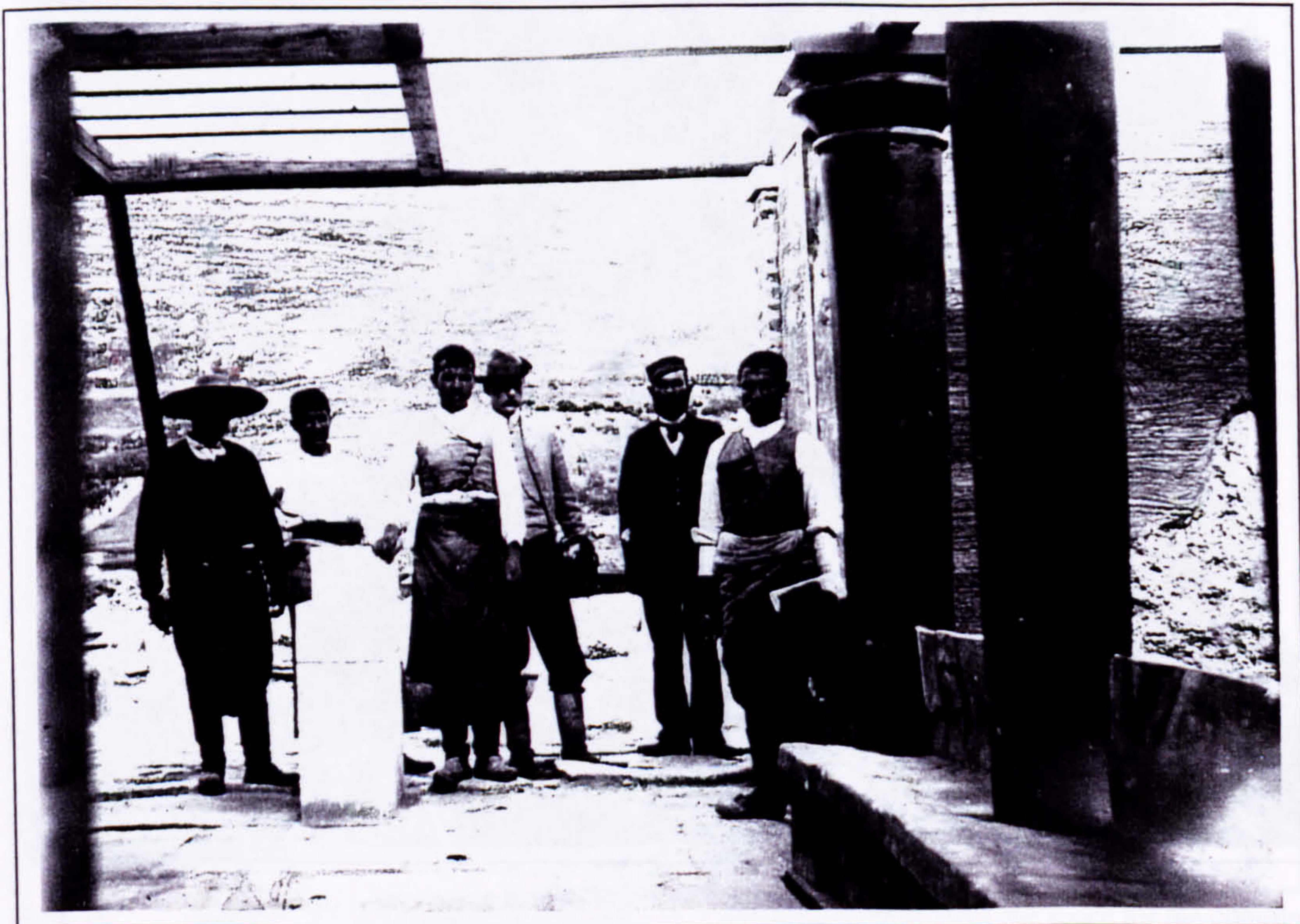
Plate 48 Construction of the flat roof of the Throne Room in 1901. Note the stone pillar.
