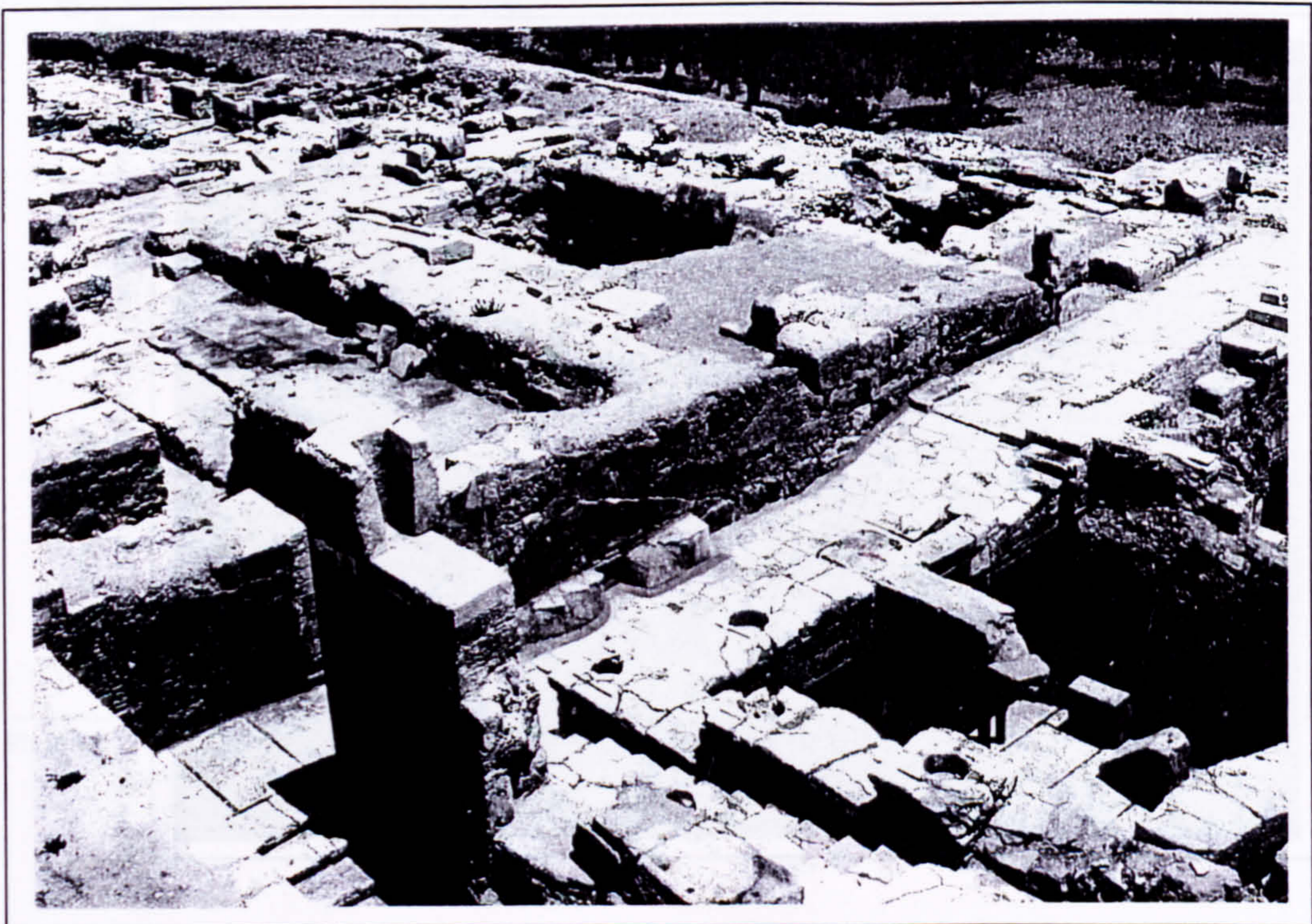
Plate 98 Grand Staircase and Hall of the Colonnades in 1902. Note the basin formed by the reconstructed first floor and the original floor height marked by the slabs sticking to the wall.
