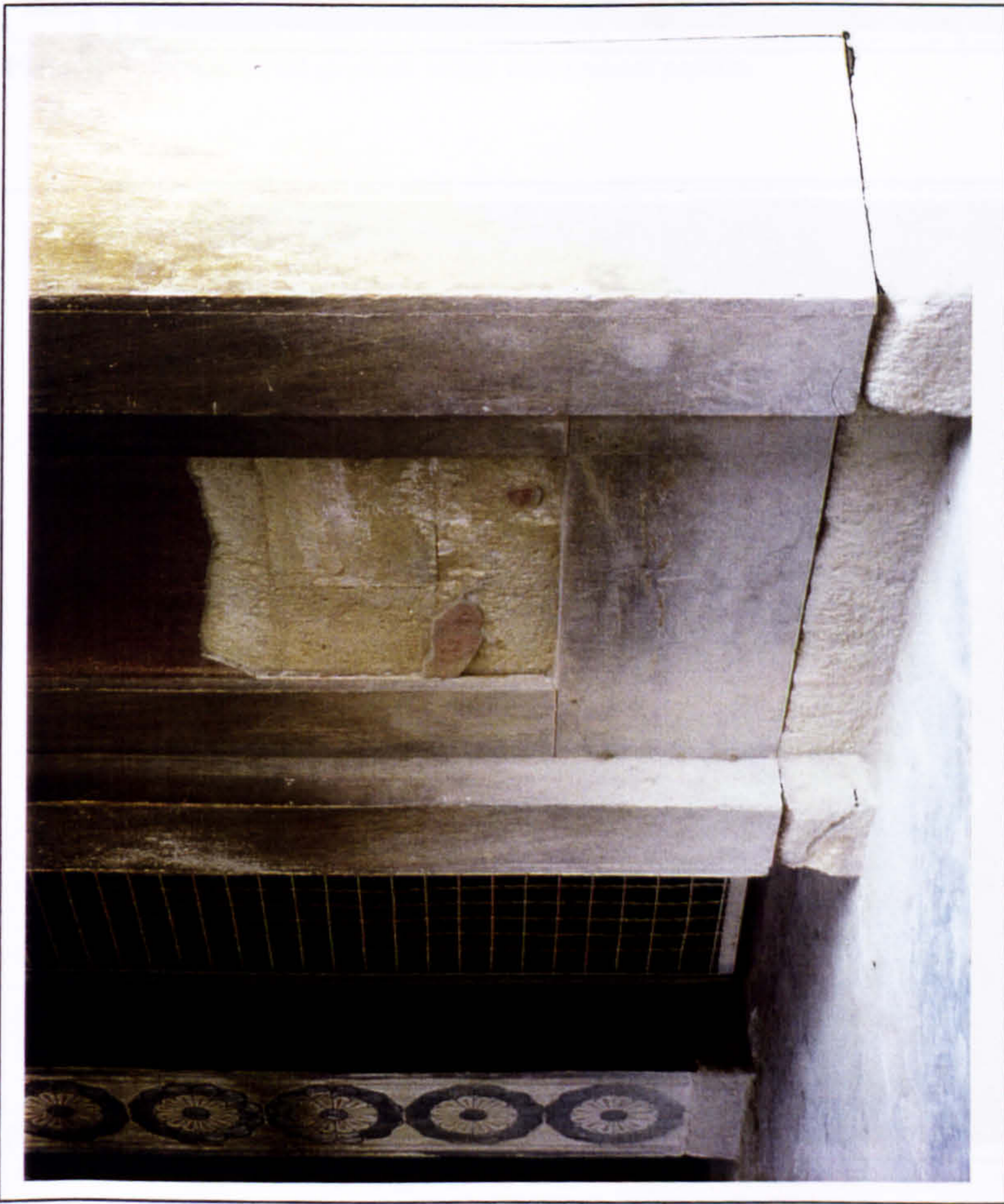
Plate 194 Detail of the door jamb construction in the Queen's Megaron. Compare with plate 183 to see the construction of the masonry pillar behind the boards.
