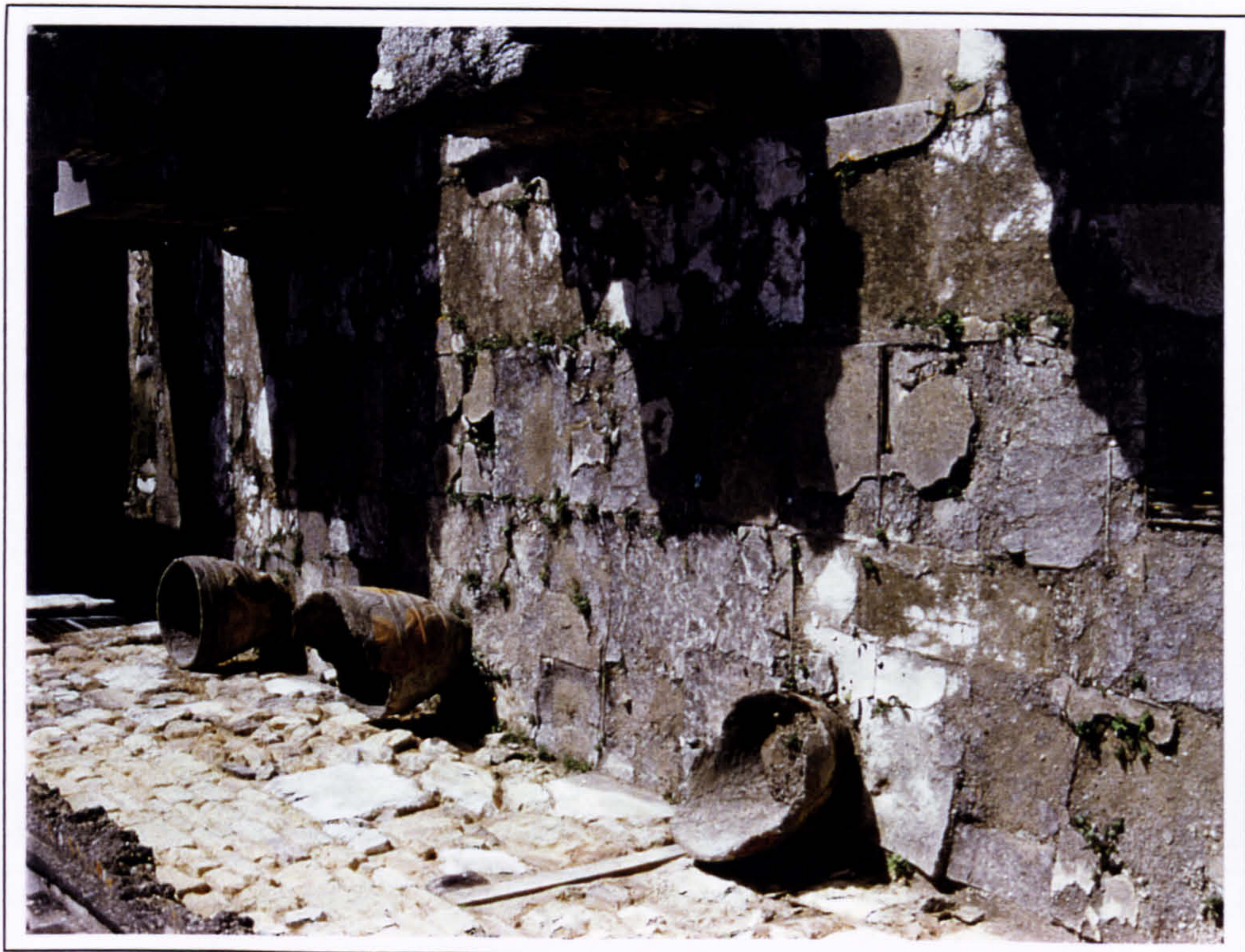
Plate 24 Long Corridor looking south in 1997.
