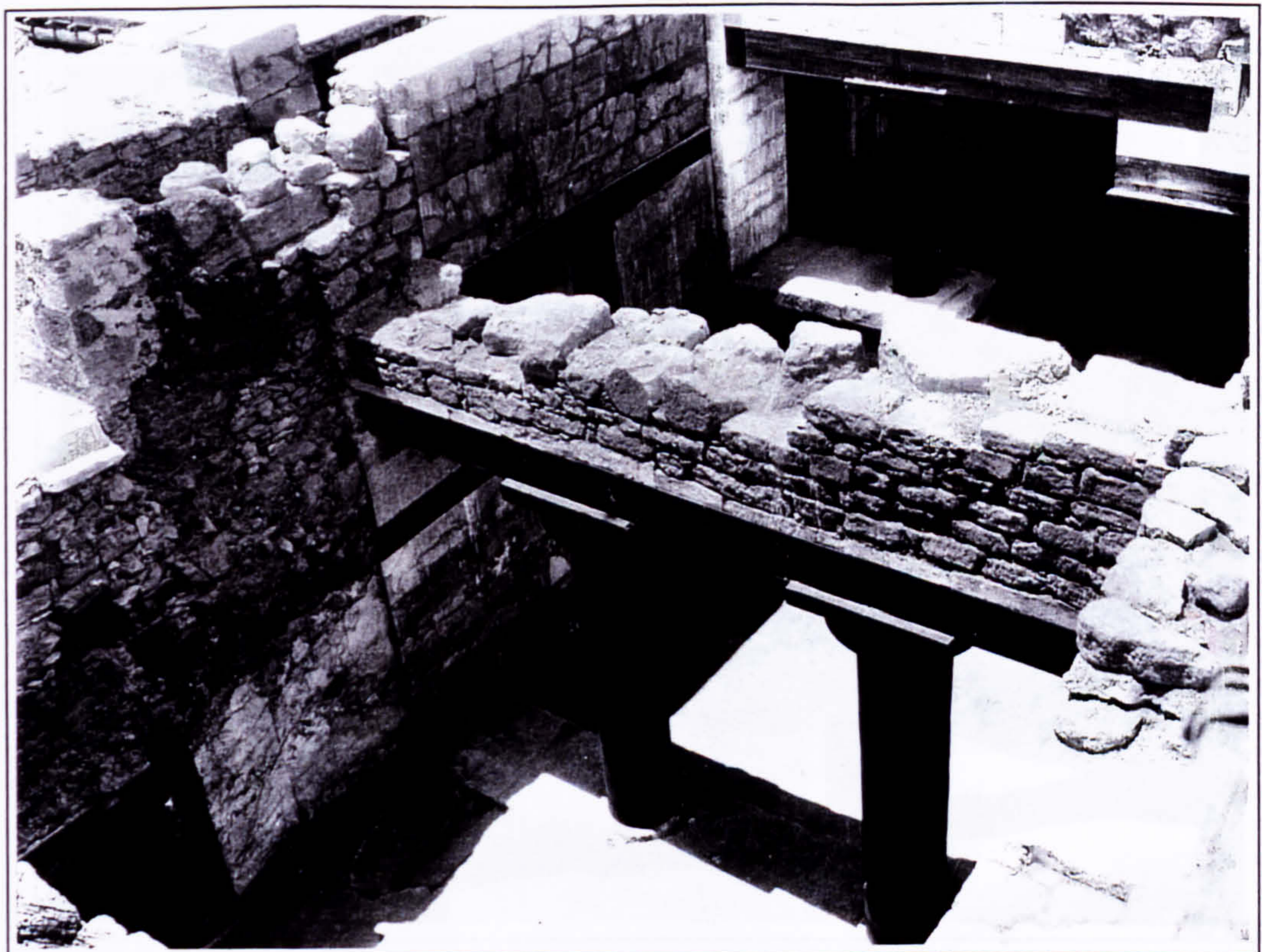
Plate 112 Hall of the Colonnades and Grand Staircase after the reconstruction work of 1905.
