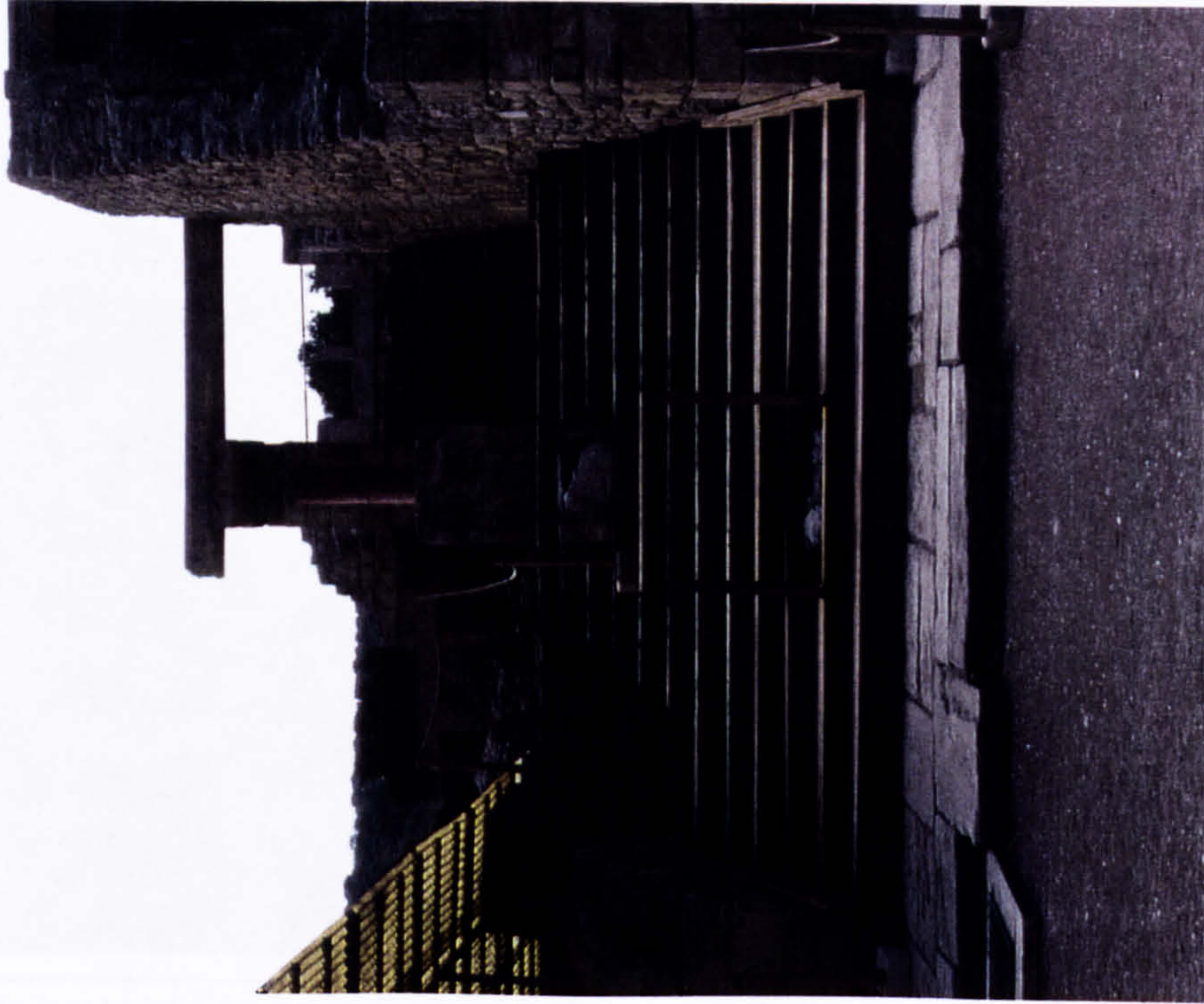
Plate 36 Stepped Portico looking west in 1998. Note subsidence of lower steps of upper flight of steps.
