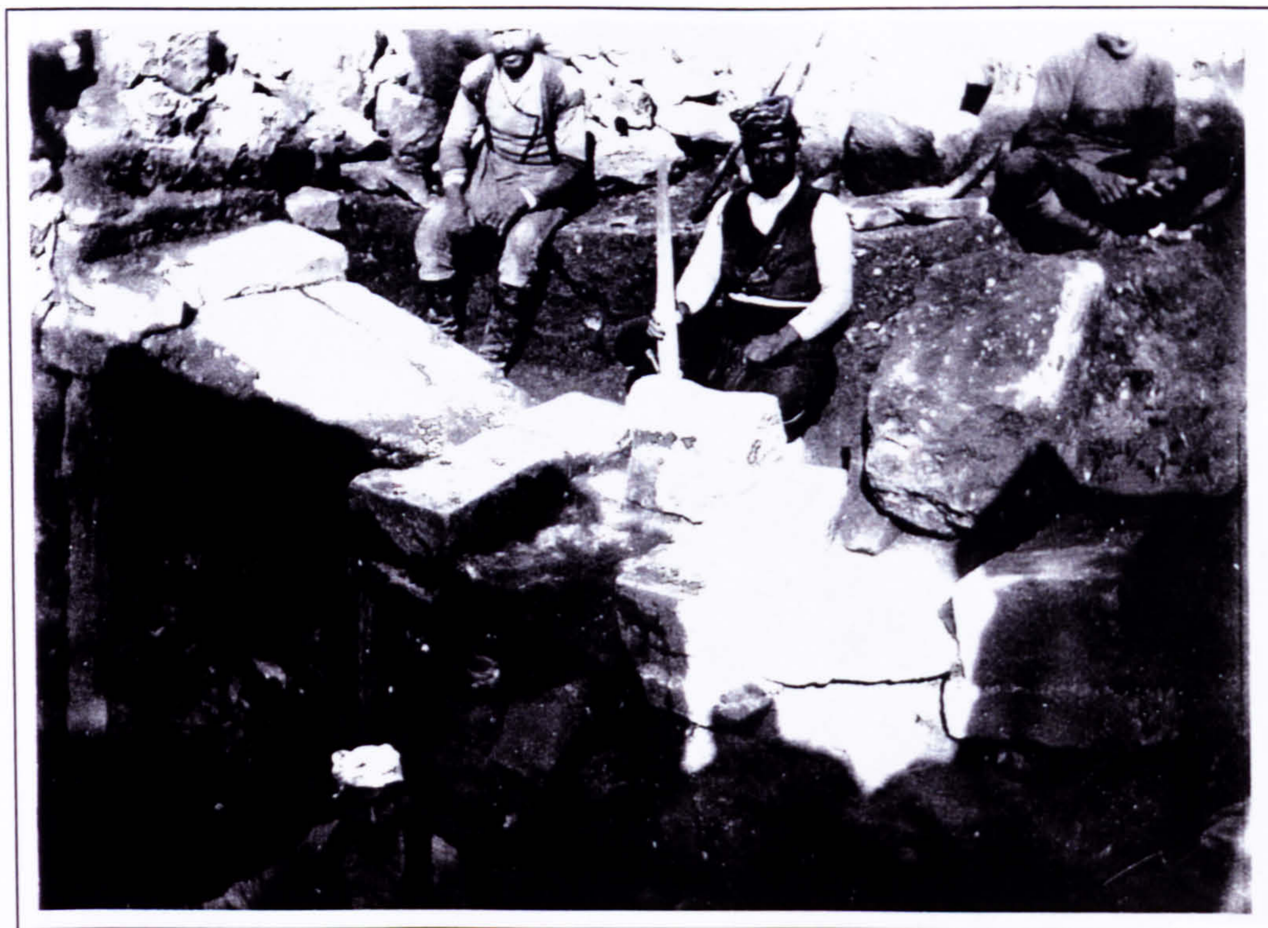
Plate 133 Excavation work in the Hall of the Double Axes in 1901. Note the poles in position to support the door jambs and sills of the first floor level.
