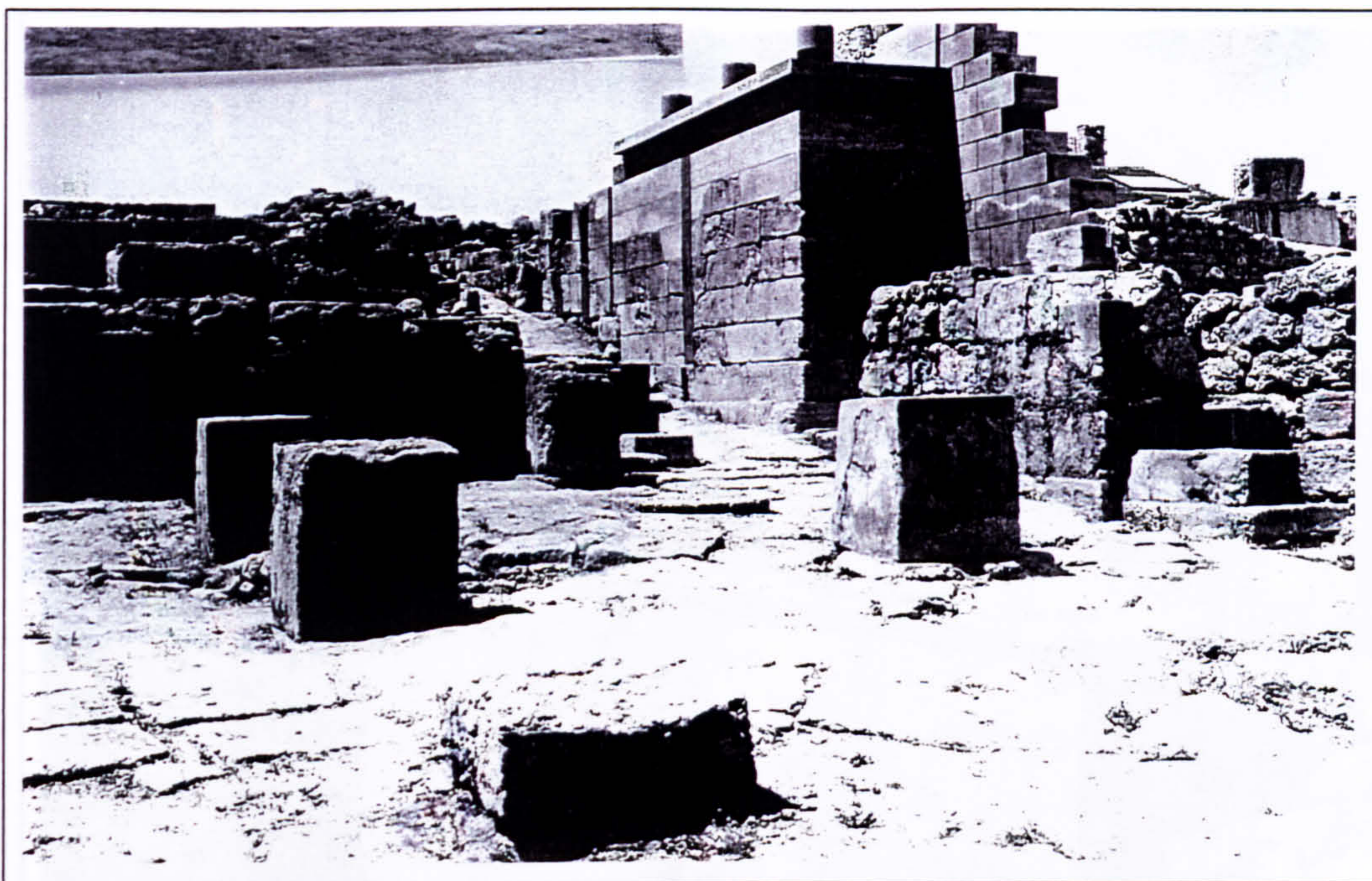
Plate 81 North Entrance Passage after the first restoration in 1929.
