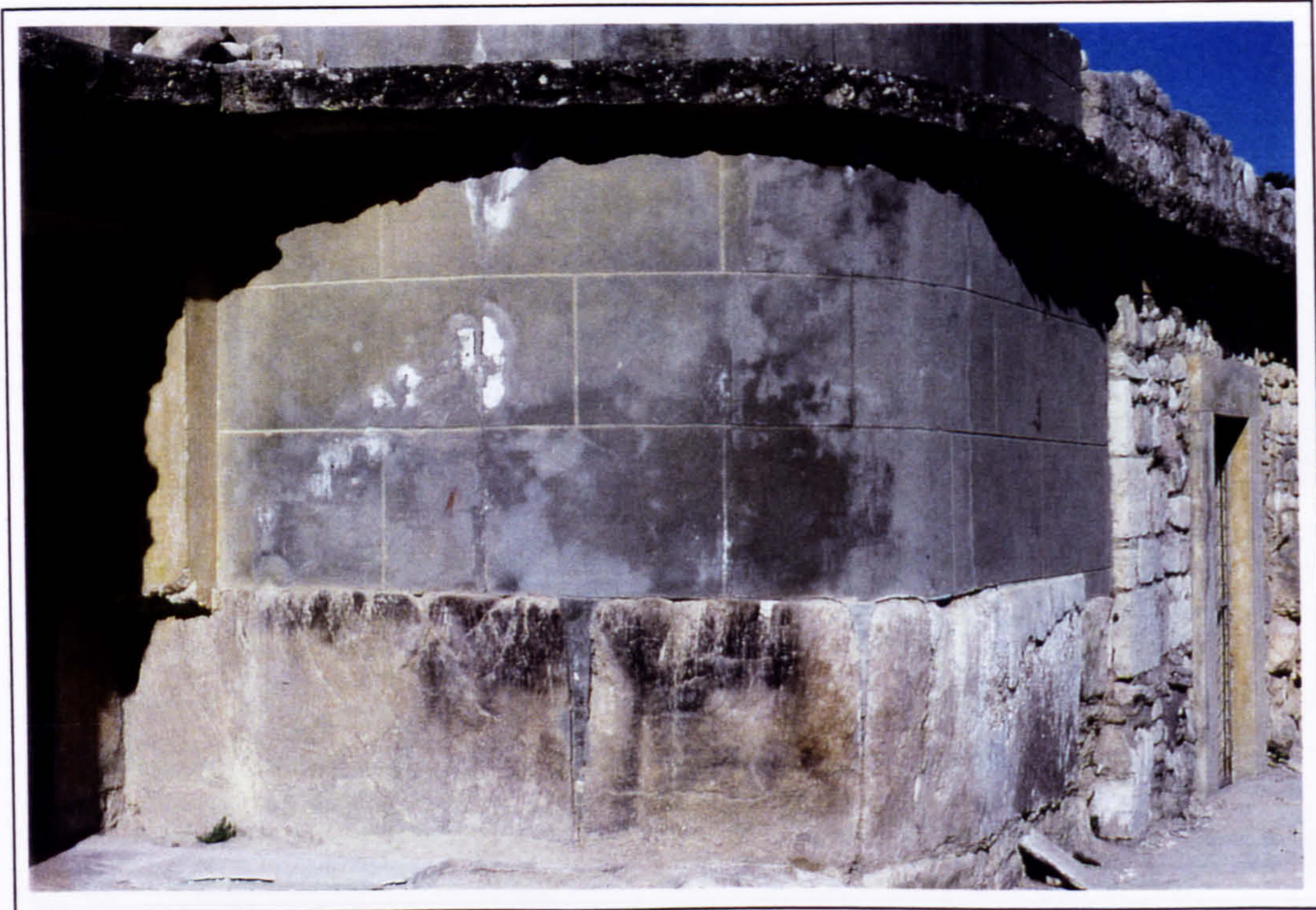
Plate 67 Round corner of the Throne Room in 1997. Note rugged edge indicating continuation of the reconstructed concrete ceiling.
