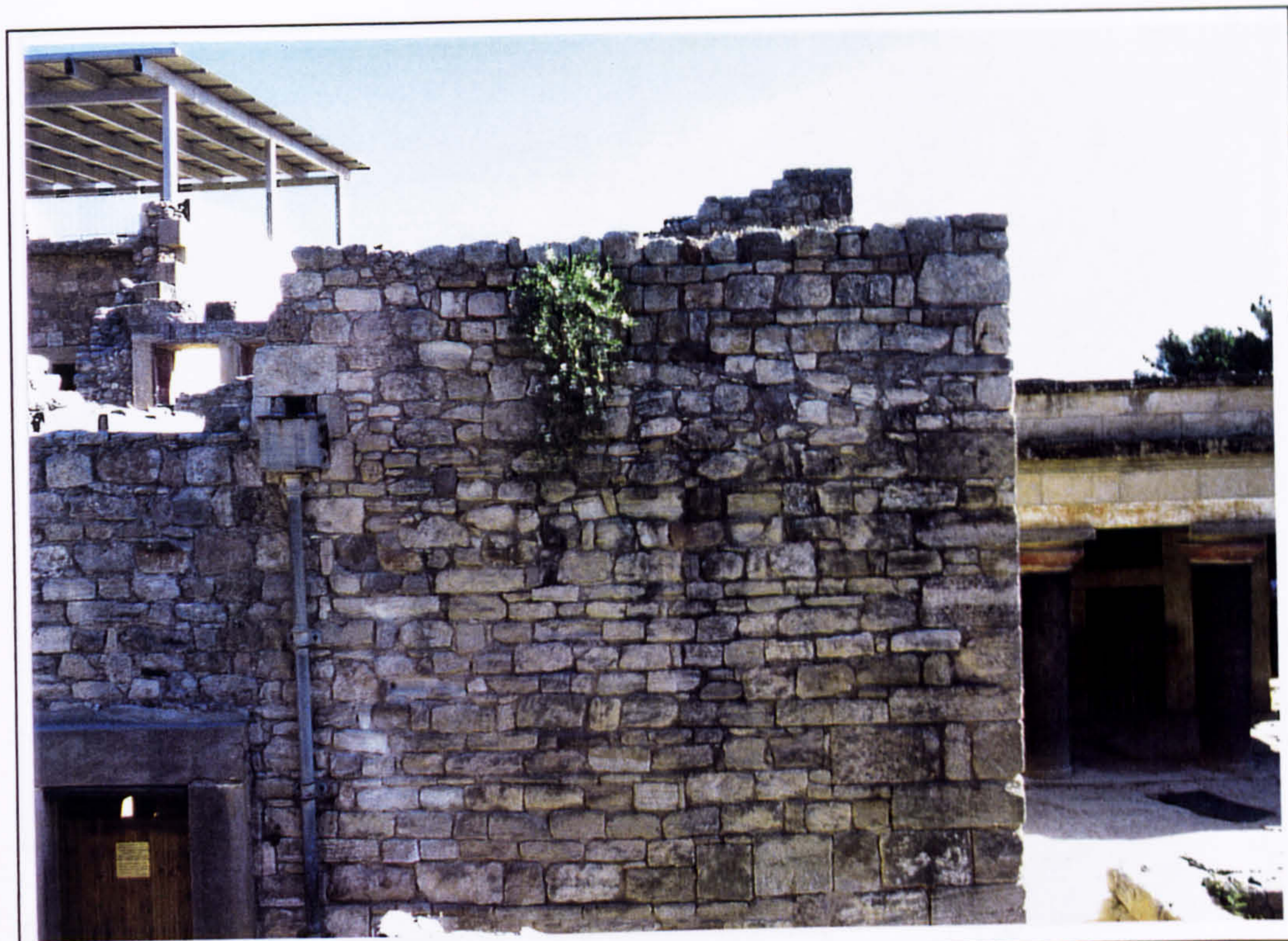
Plate 190 Queen's Megaron south wall of the light-well showing incline of former pitched roof.
