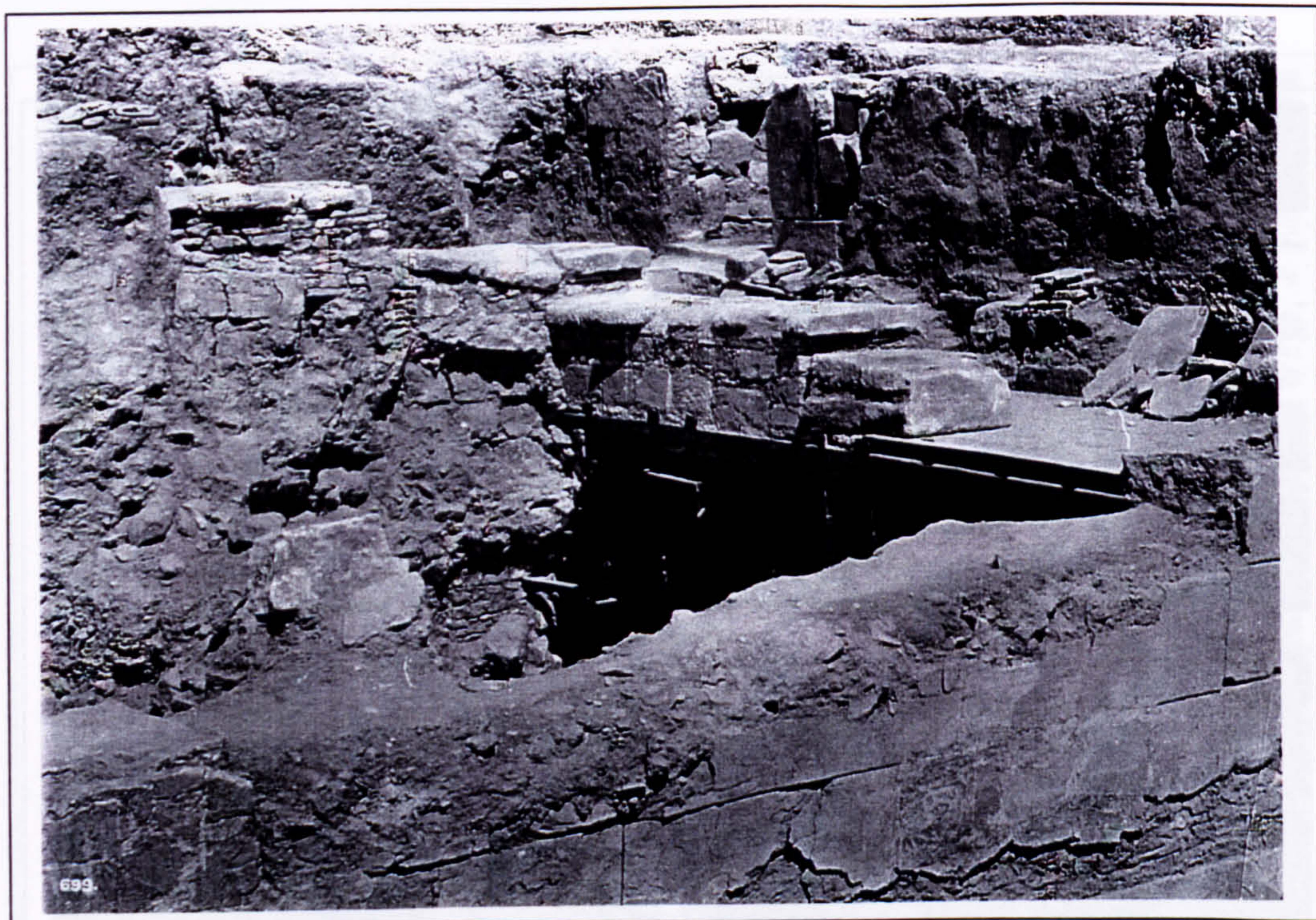
Plate 94 The second support work of the northern portico of the Hall of the Colonnades in 1901. Note the timber floor, the stacked gypsum floor slabs (right) and the original floor height marked by the slabs in original position between the end of the balustrade and the stacked slabs.
