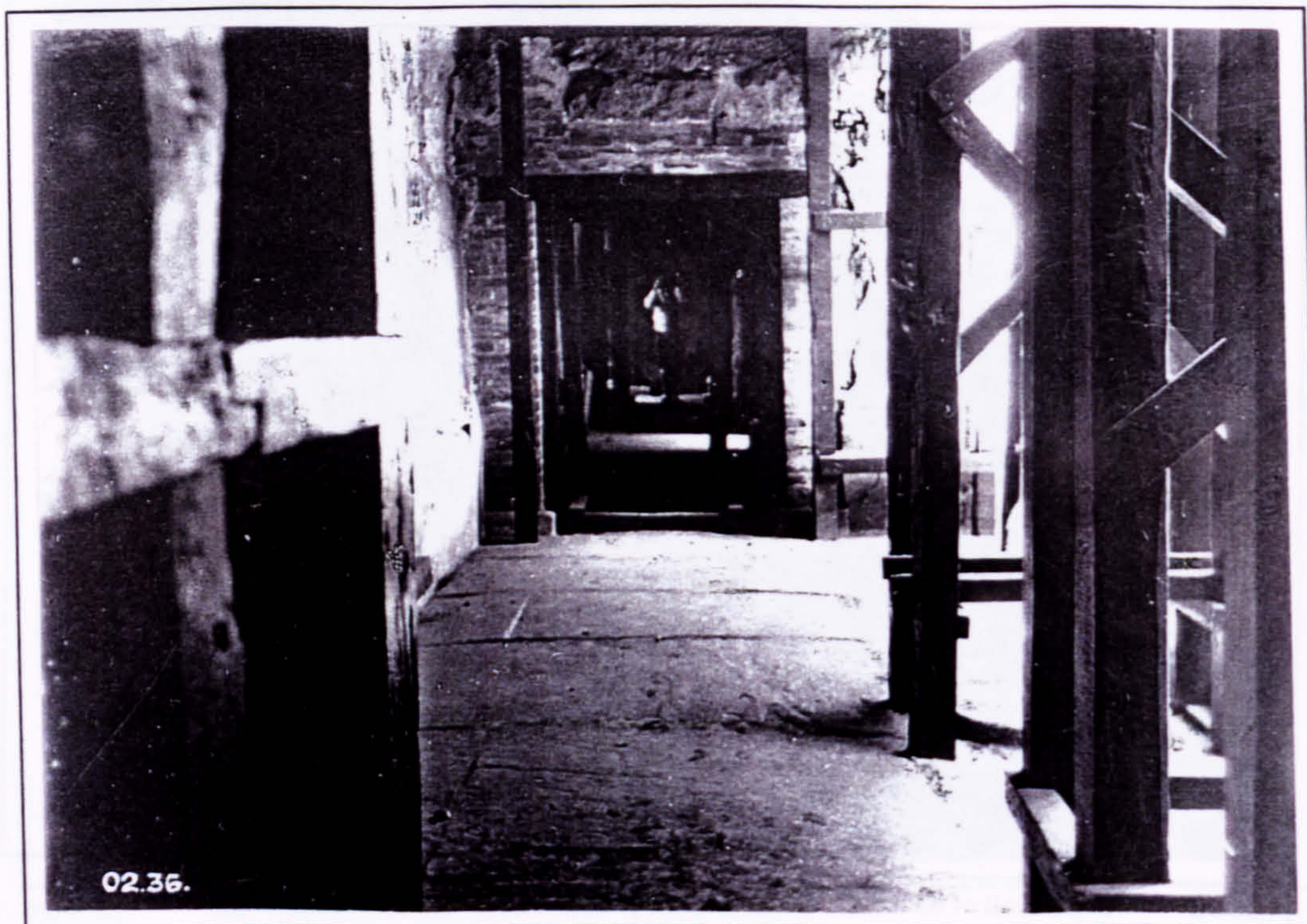
Plate 92 Second set of support-frames in the northern portico of the Hall of the Colonnades in 1902.
