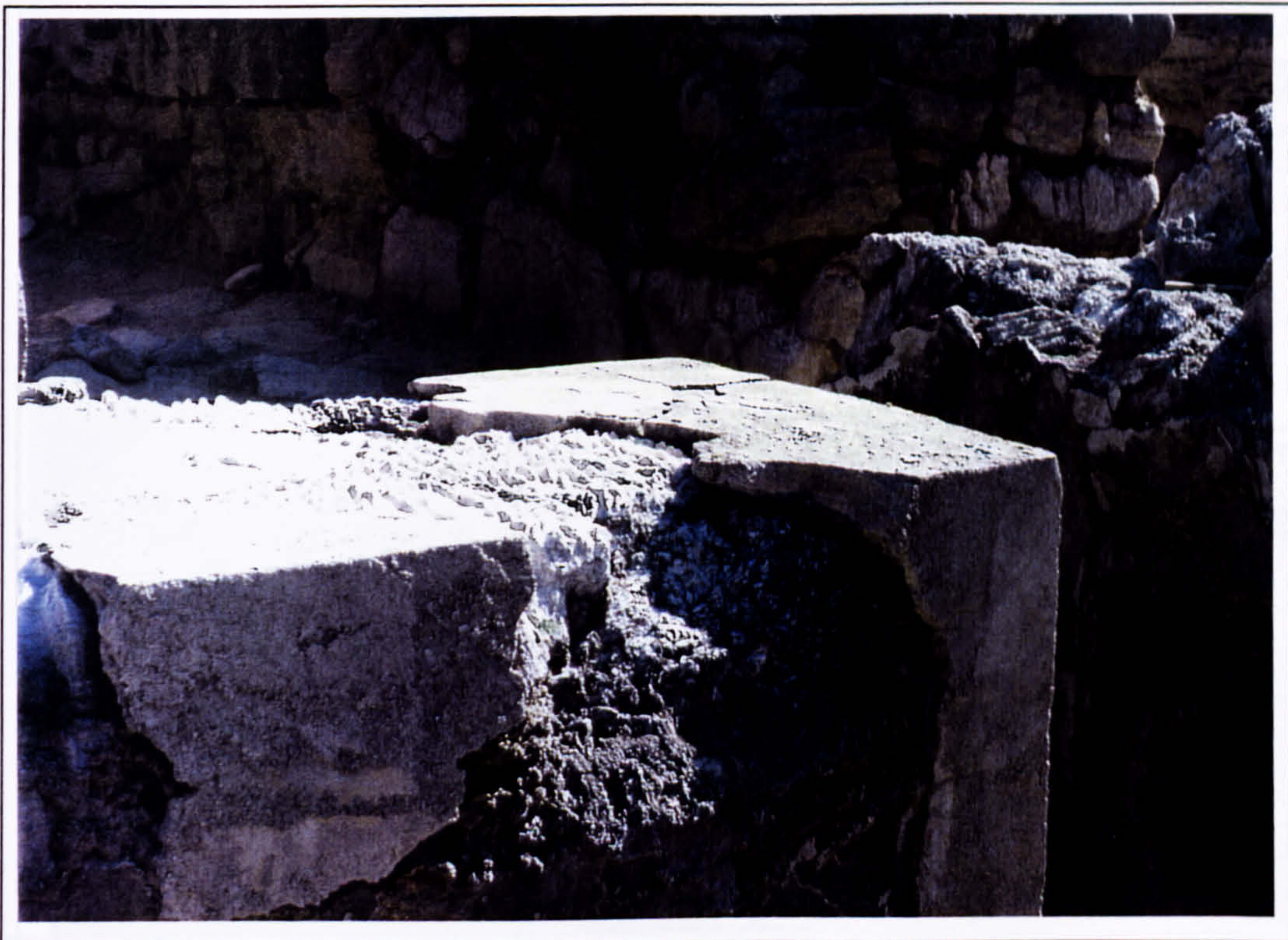
Plate 198 Decayed gypsum block with cement repairs.
