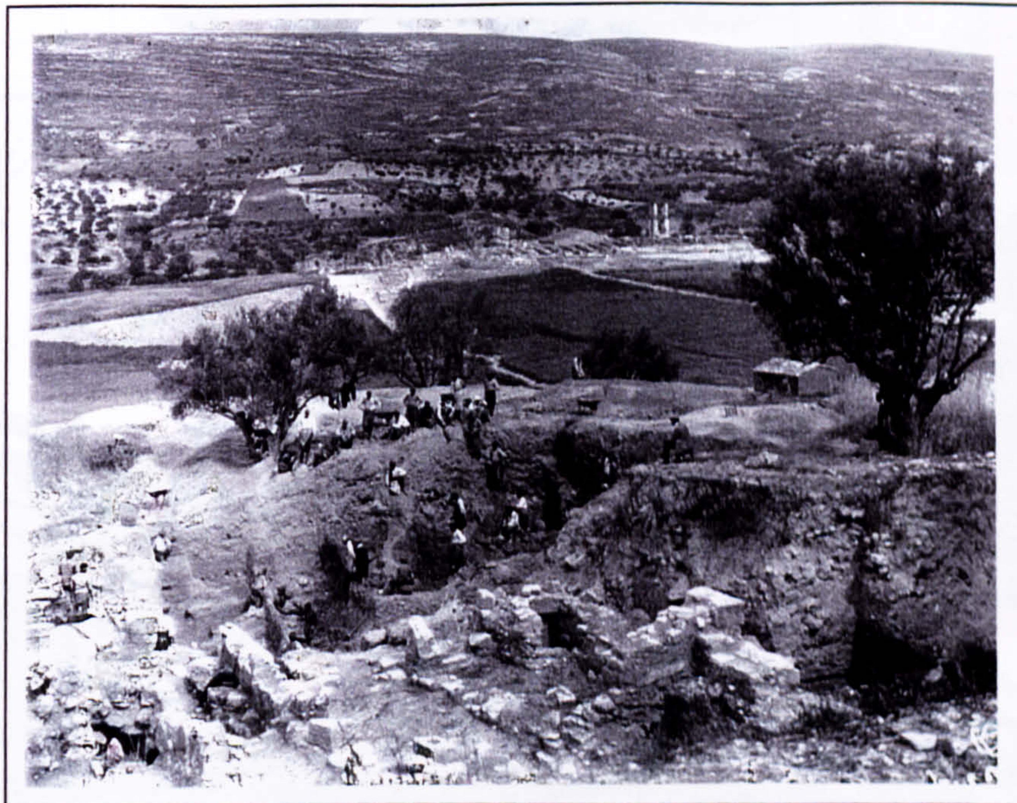
Plate 211 Excavation work in the water system in progress at the Little Palace.
