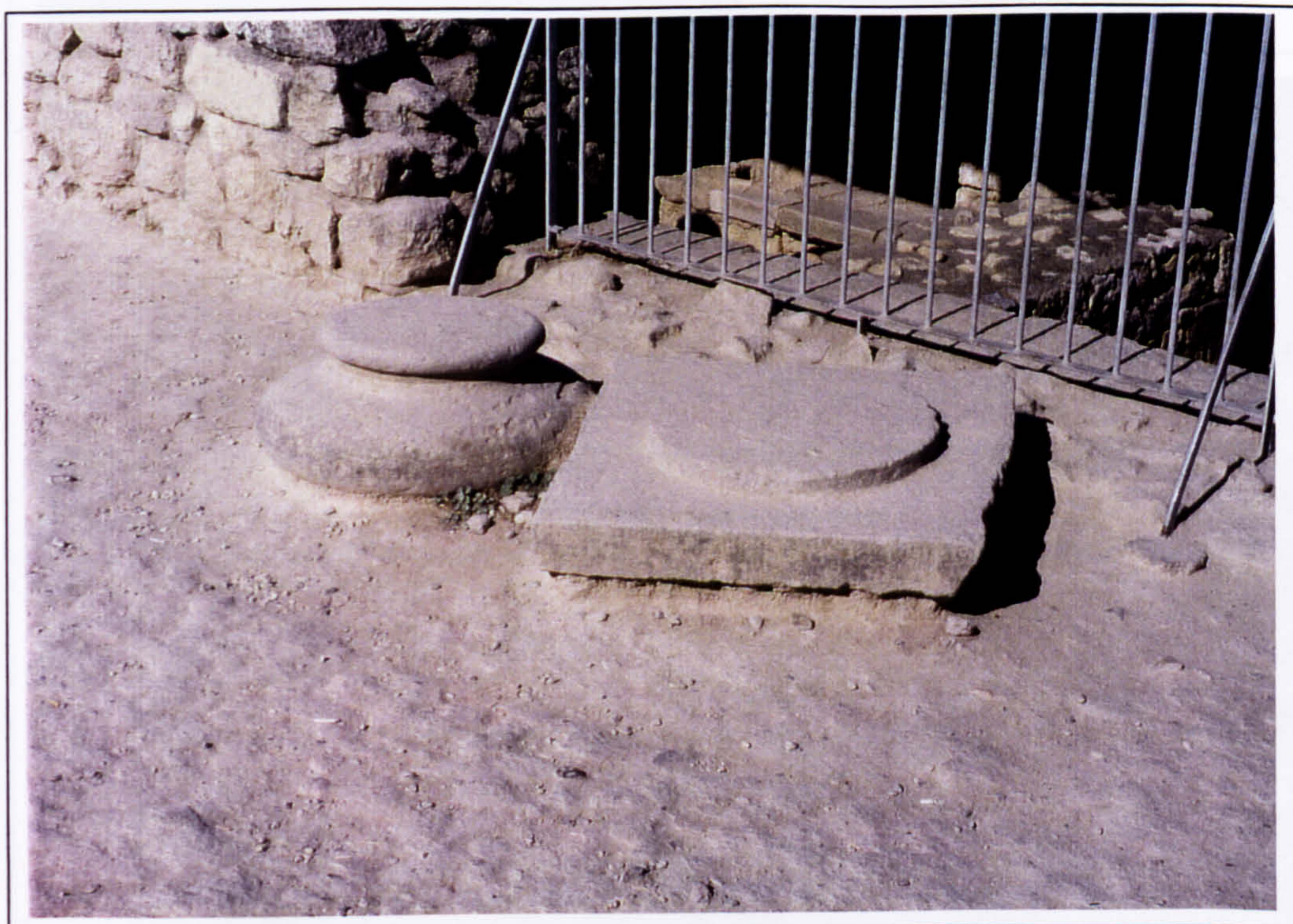
Plate 124 Capital and abacus of the column of the third landing. Removed by Nikolaos Platon after World War II in order to fit the steel pole and corrugated plastic shelter.
