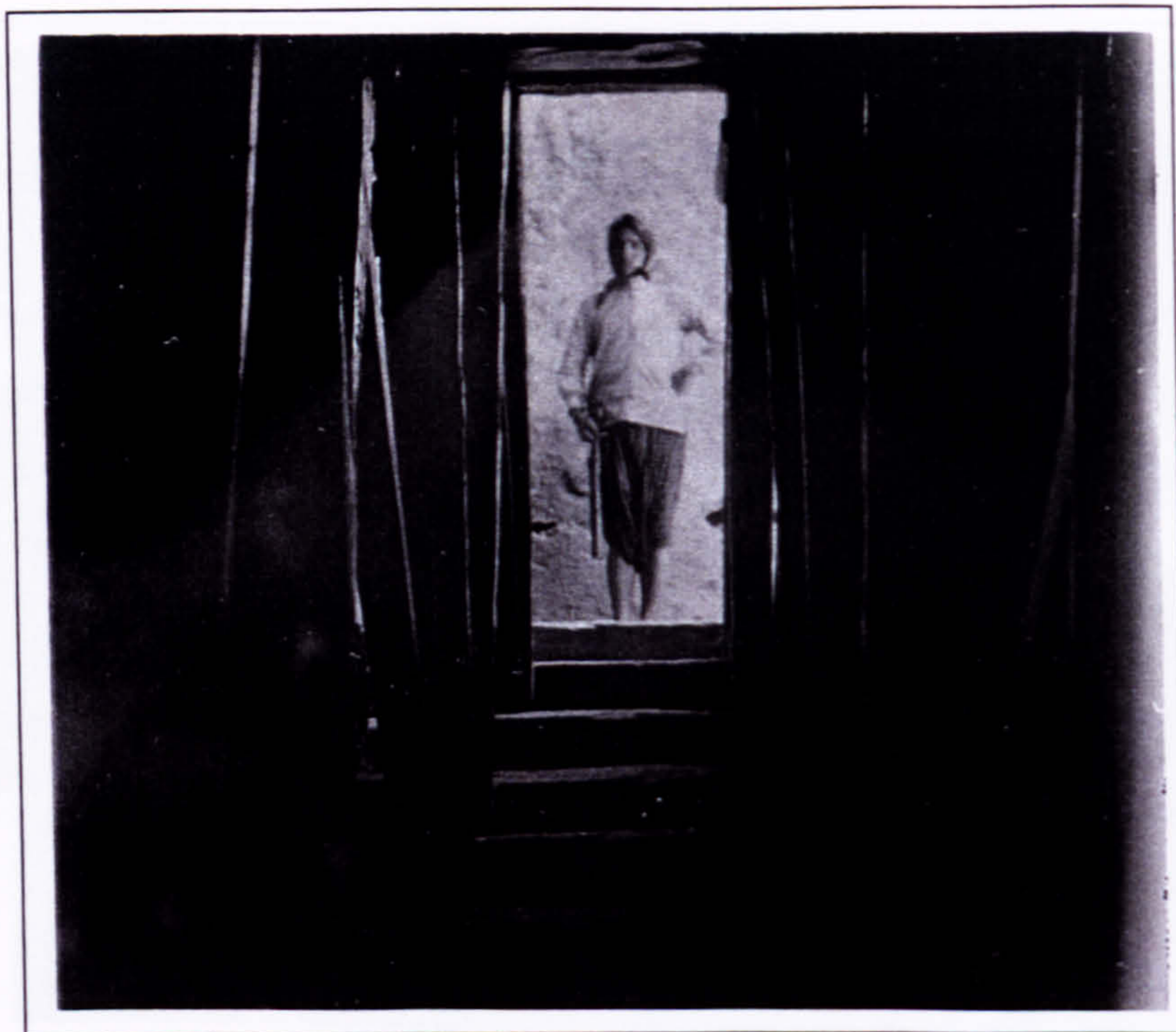
Plate 91 Support-frames in the tunnel under the third flight of the Grand Staircase in 1901.
