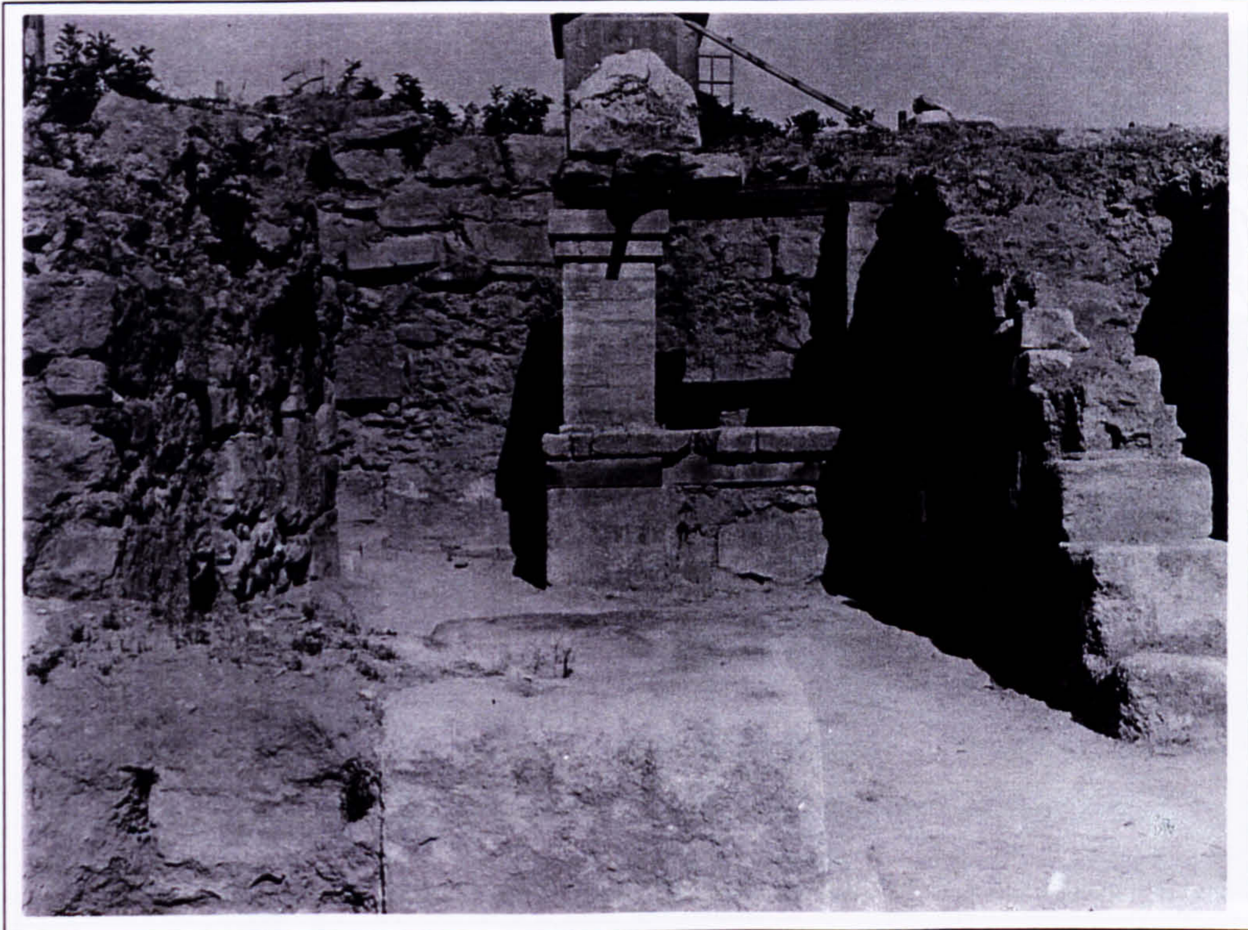
Plate 131 Lobby of the Wooden Posts after reconstruction in 1902.
