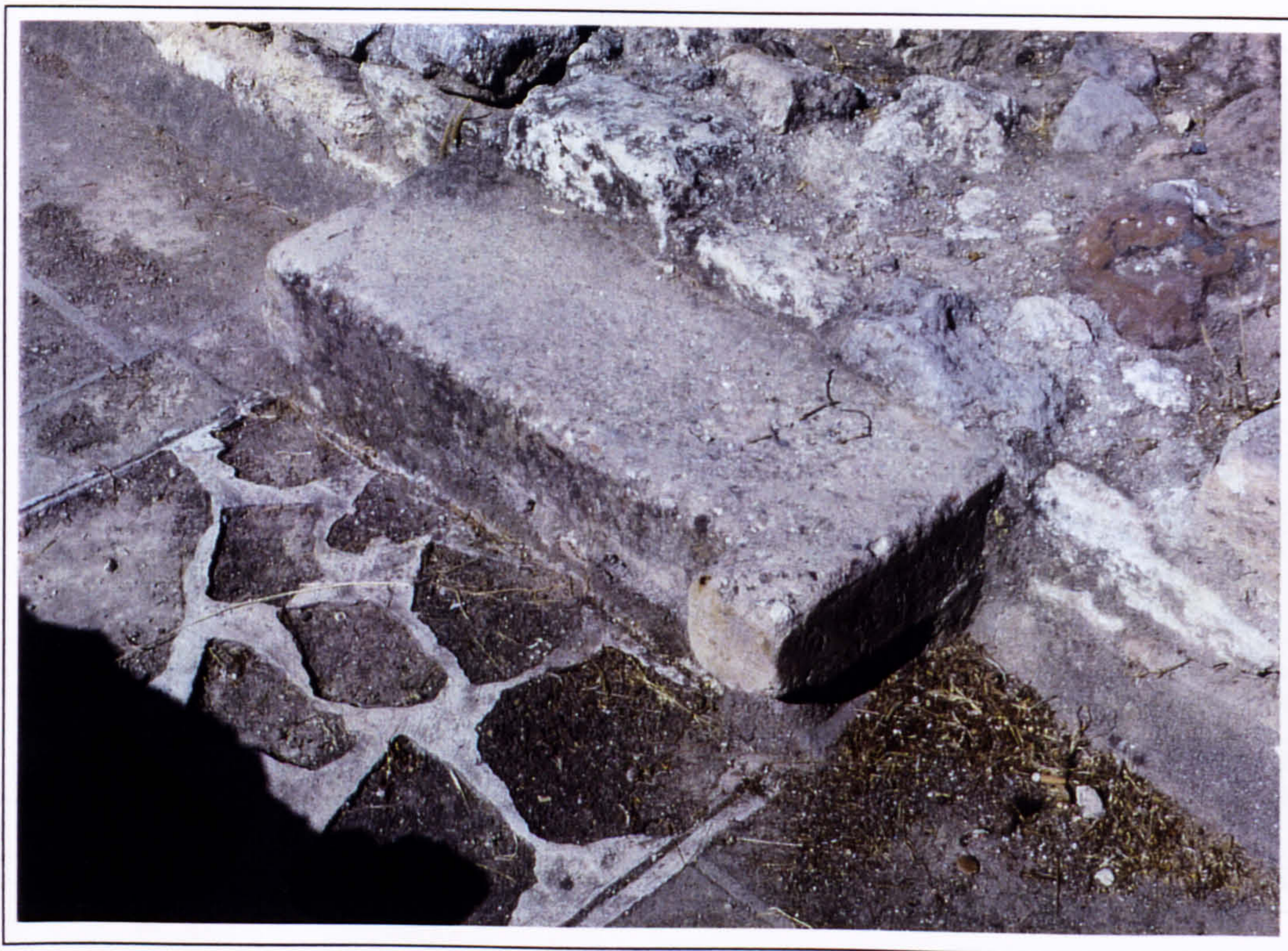
Plate 176 Cast concrete door jamb of Doll's reconstruction work of the Domestic Quarter.
