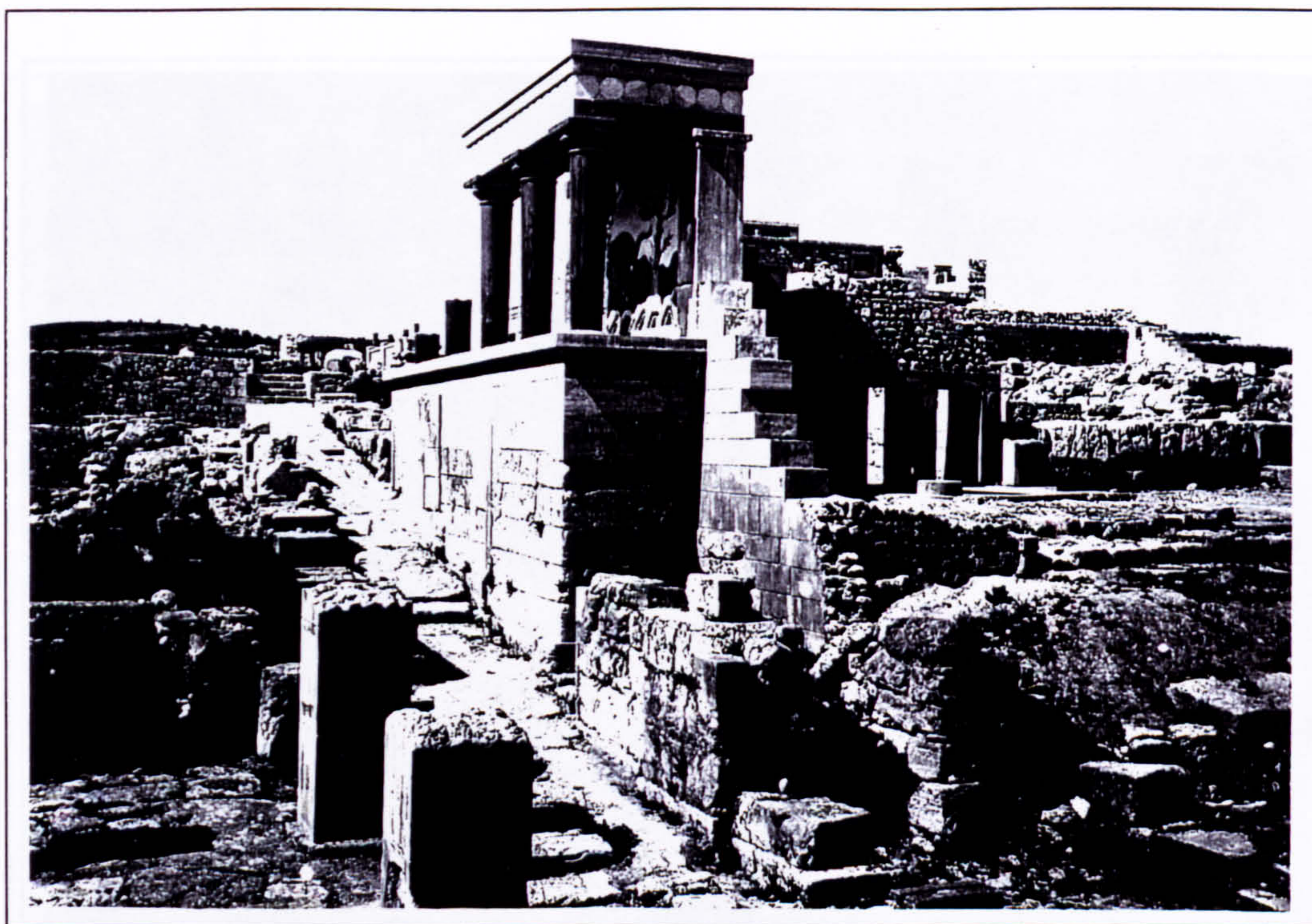
Plate 82 North Entrance Passage after its second restoration in 1930.
