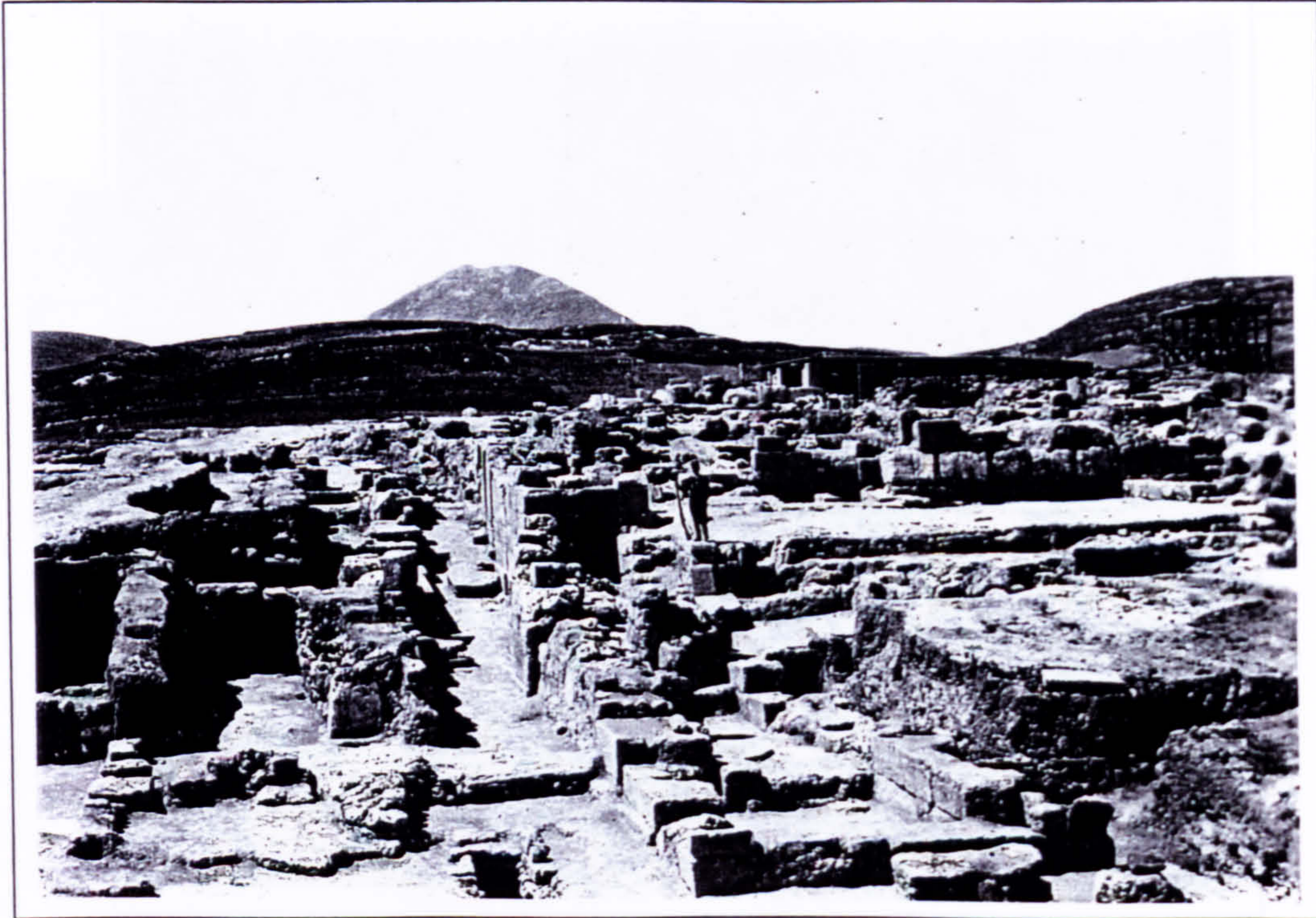
Plate 79 North Entrance Passage after its excavation in 1901 looking south. Note the flat roof of the Throne Room and the first observation tower in the background.
