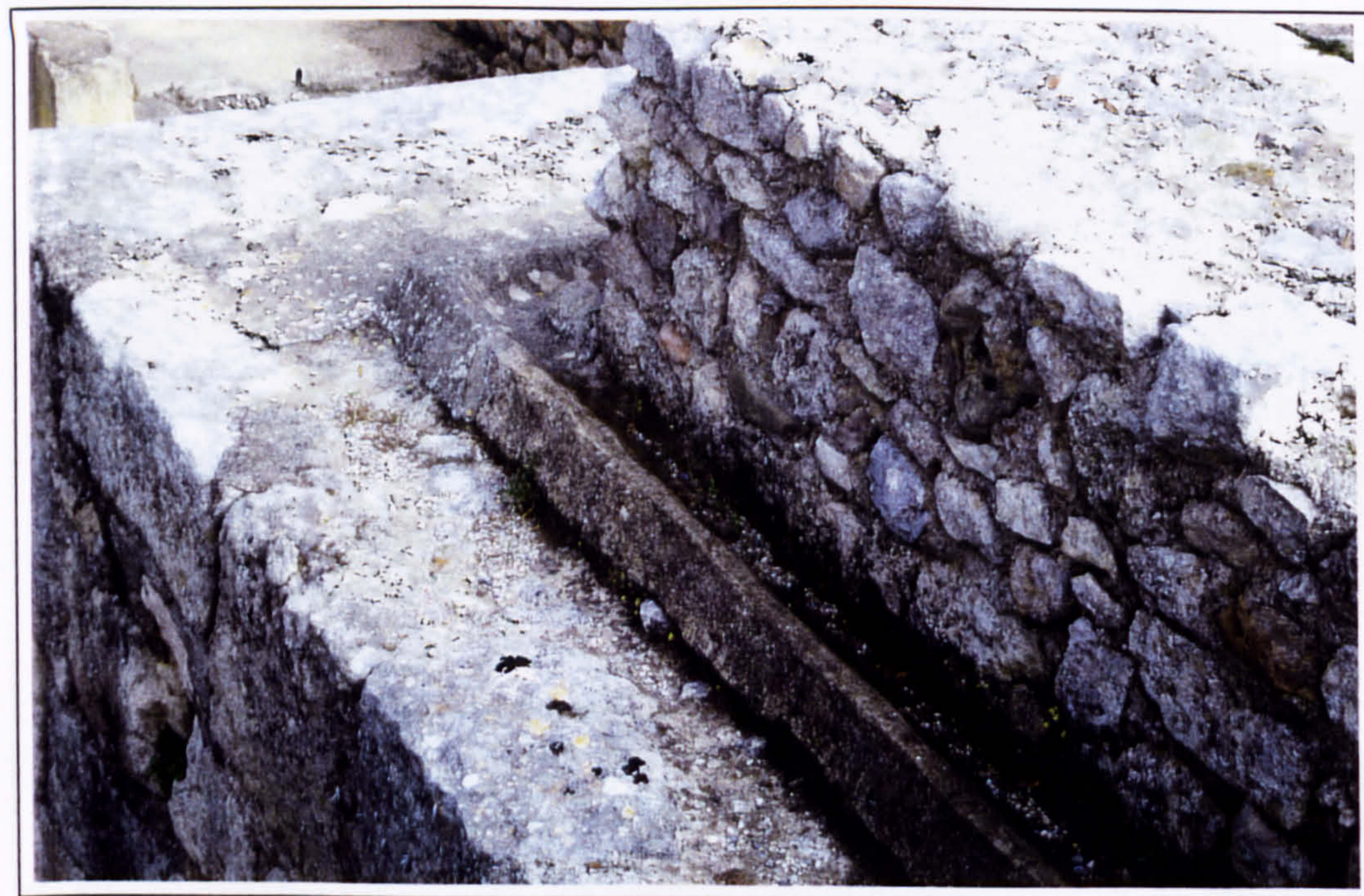
Plate 28 Concrete drain canal at the West Wing. 1997.
