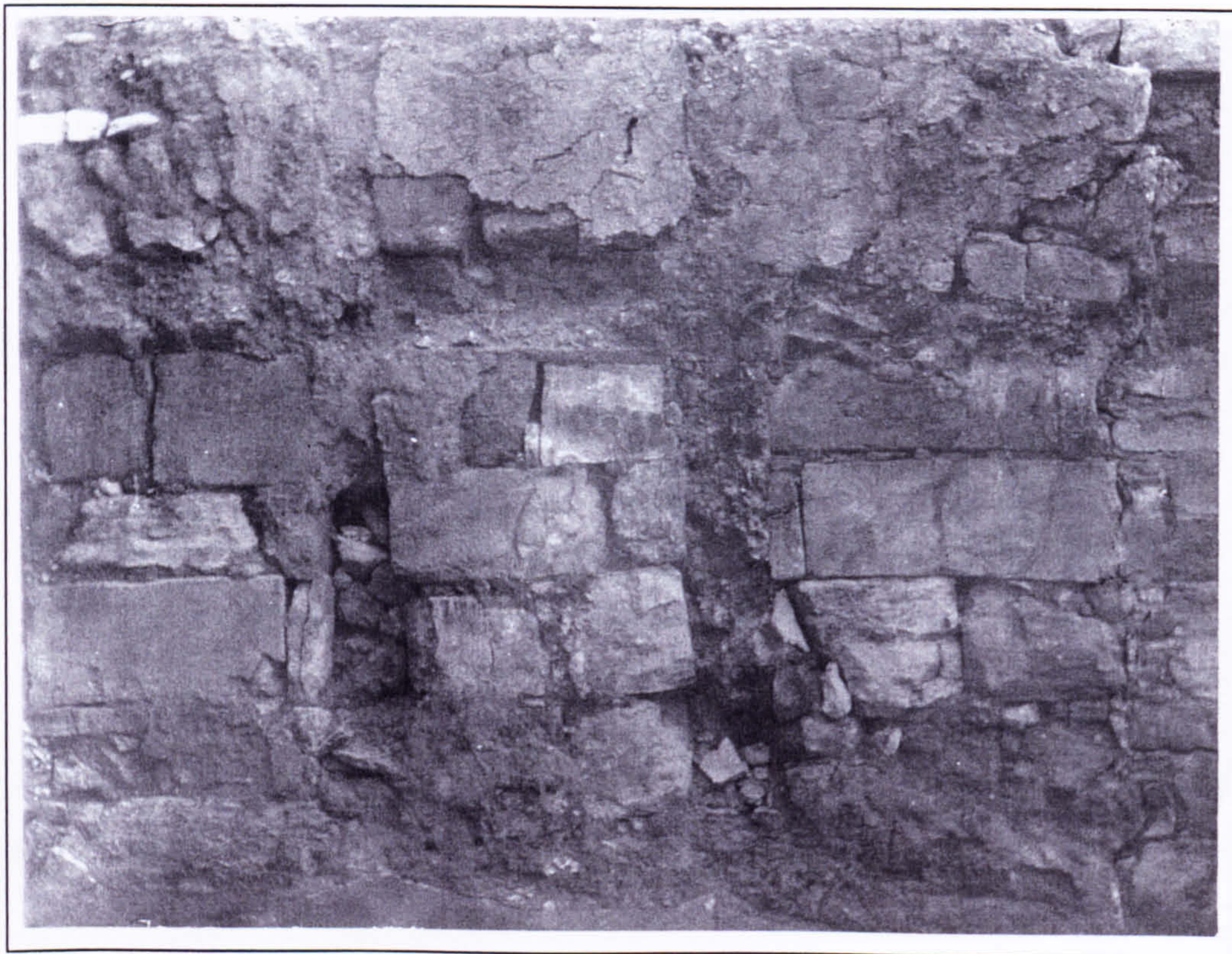
Plate 148 South wall of the Hall of the Double Axes after its excavation in 1901 with the cavities left by the rotted timber reinforcement beams.
