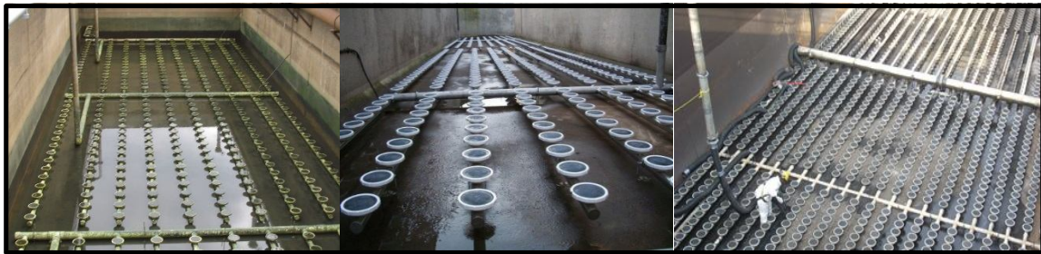
Figure 2.5: Sparger aerators
