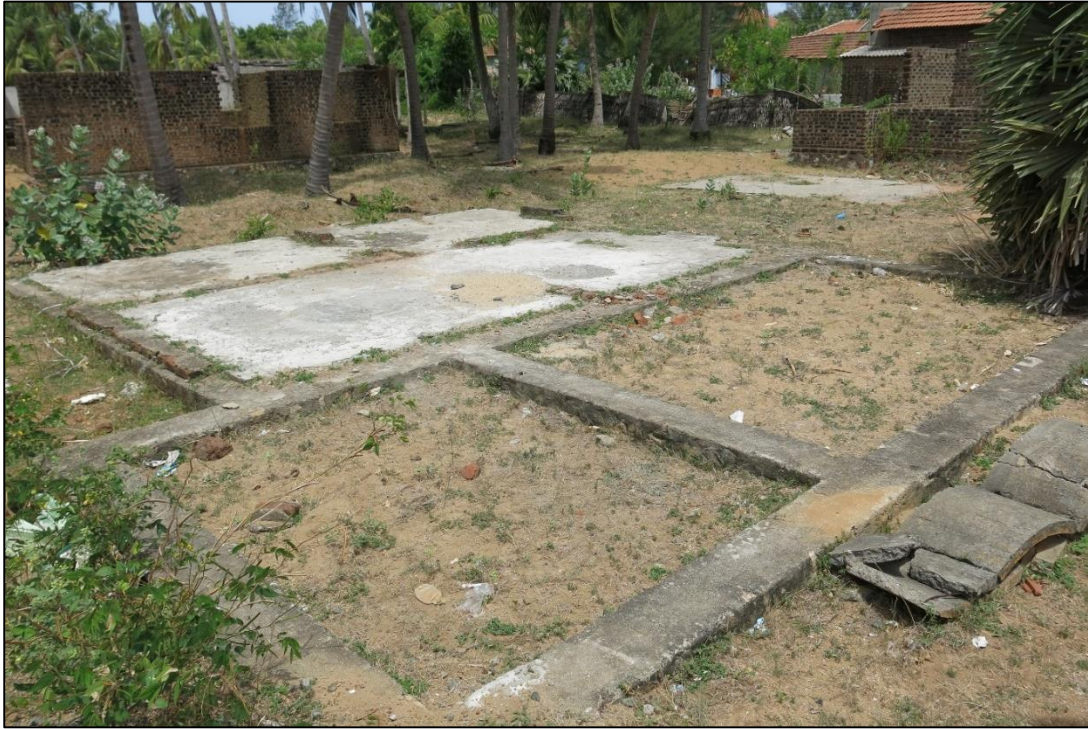
Figure 7.i Tsunami ruins, Arugam Bay. Photo: Author
