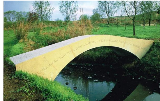
Fig. 8.20 Arched bridge with inscription: ARCH, n. A MATERIAL CURVE SUSTAINED BY GRAVITY AS RAPTURE BY GRIEF (Sheeler 2003, p32)
