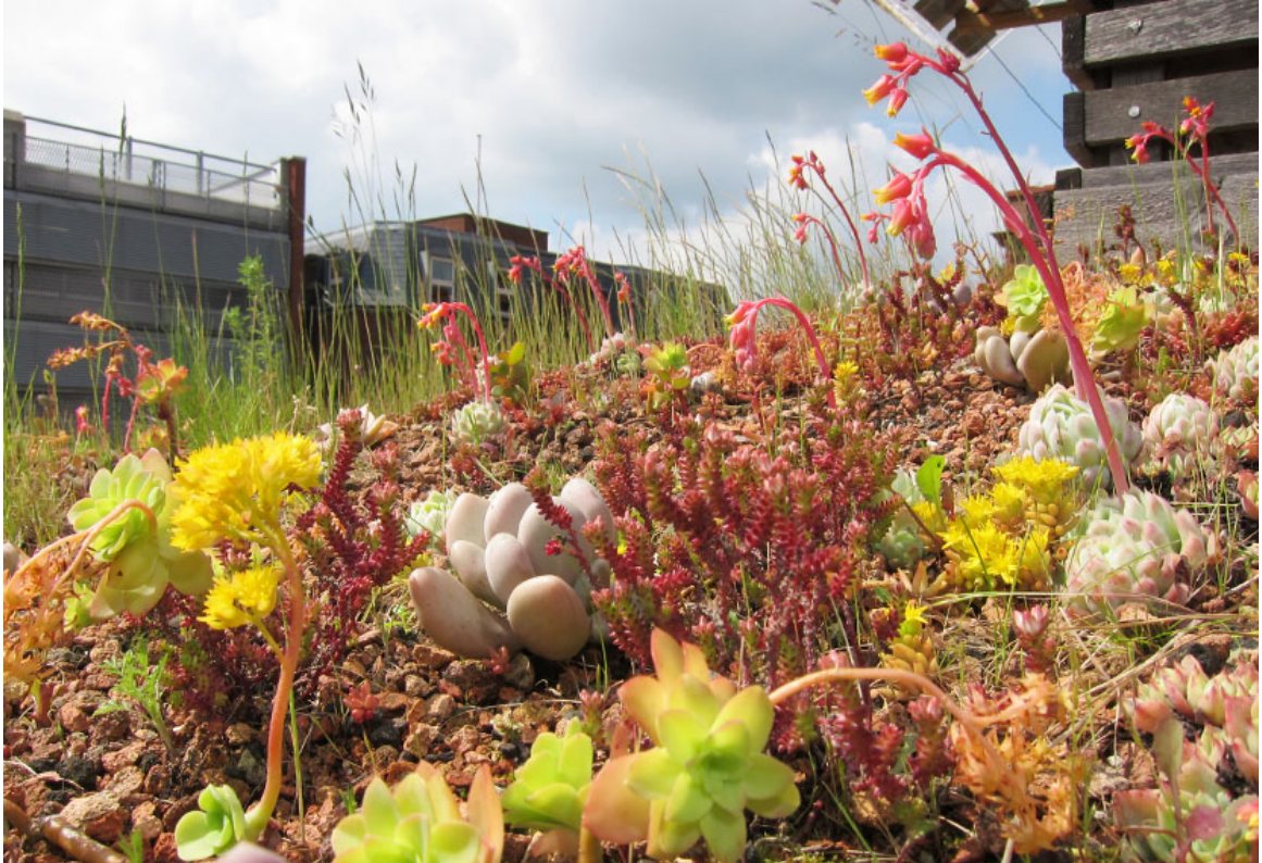
Figure 5.2.34 Sedum palmeri , S. reptans and E. elegans flowering at the first week of June 2014 on the Demonstration Roof of the Green Roof Centre of the University of Sheffield.
