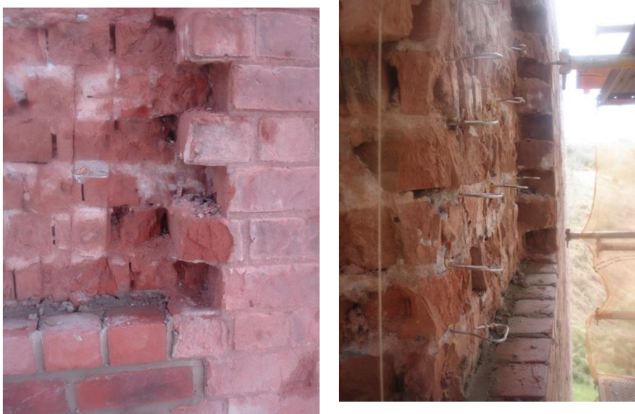
Figure 5.24 : Repair of the brickwork on piers of Larpool Viaduct, illustrating ties.
