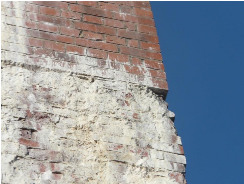
Figure 5.11: Pier rehabilitation works on Larpool Viaduct.
