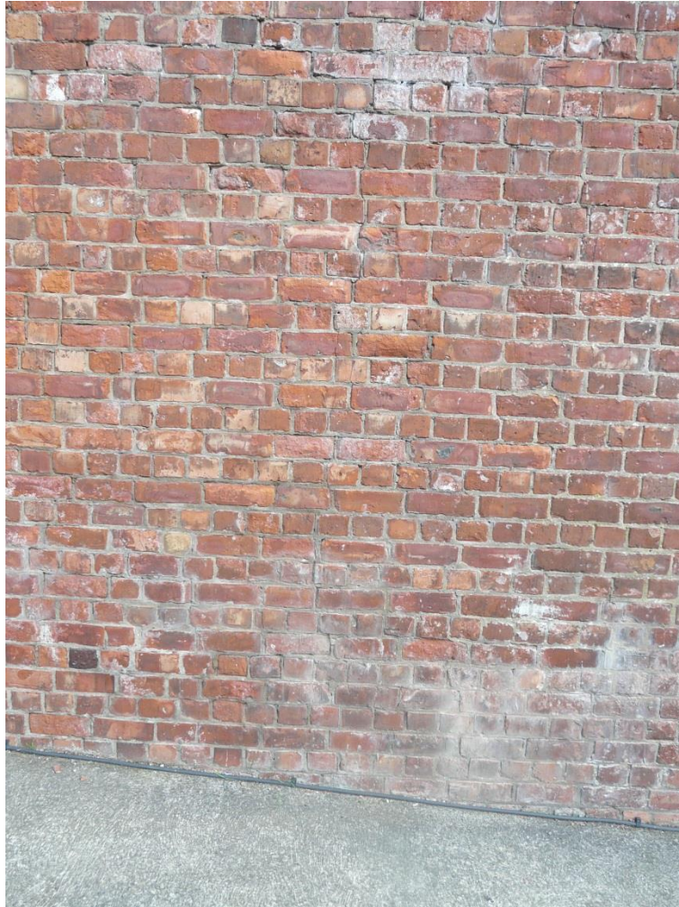
Figure F.7: Vertical cracks seen on the bottom 2.5 meters of the pier
