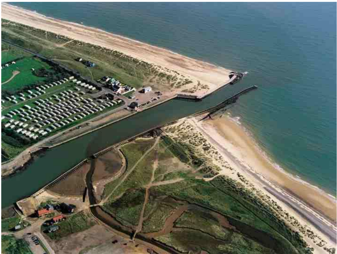
Figure 12, Oblique aerial photograph of Southwold harbour piers, looking NE. The material remains of older work are visible to the south side of the south pier (photo accessed via web)
