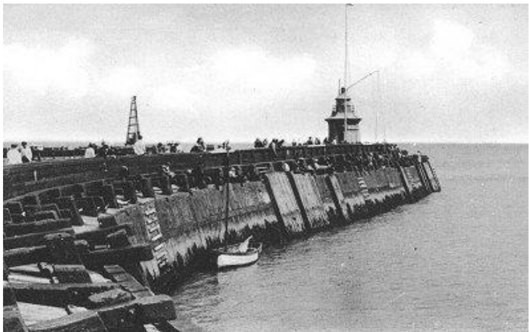
Figure 10, North Pier Great Yarmouth, earlier 20 th century. Note the short multiple stretches of tie-beam used to secure successive re-claddings (NOAH website)
