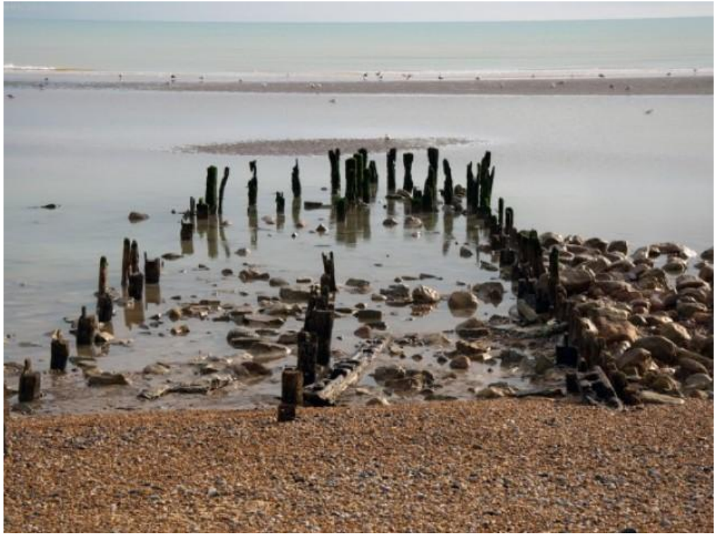
Figure 12, View of the head of the north-east pier of the 18 th century harbour, looking South-east *Photograph from Rye Museum website.
