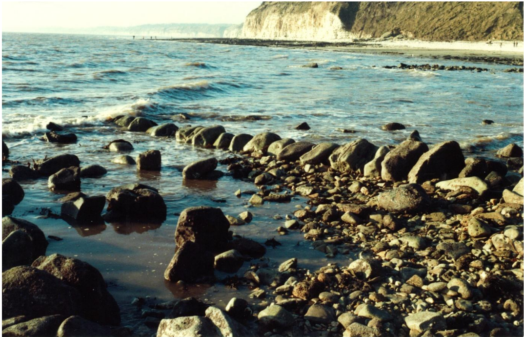
Figure 6, Part of the N.W. arm of Feature F3 at Flamborough – probable ‘rock armour’ for a pier toe. Remains of part of Feature F2 towards upper right.
