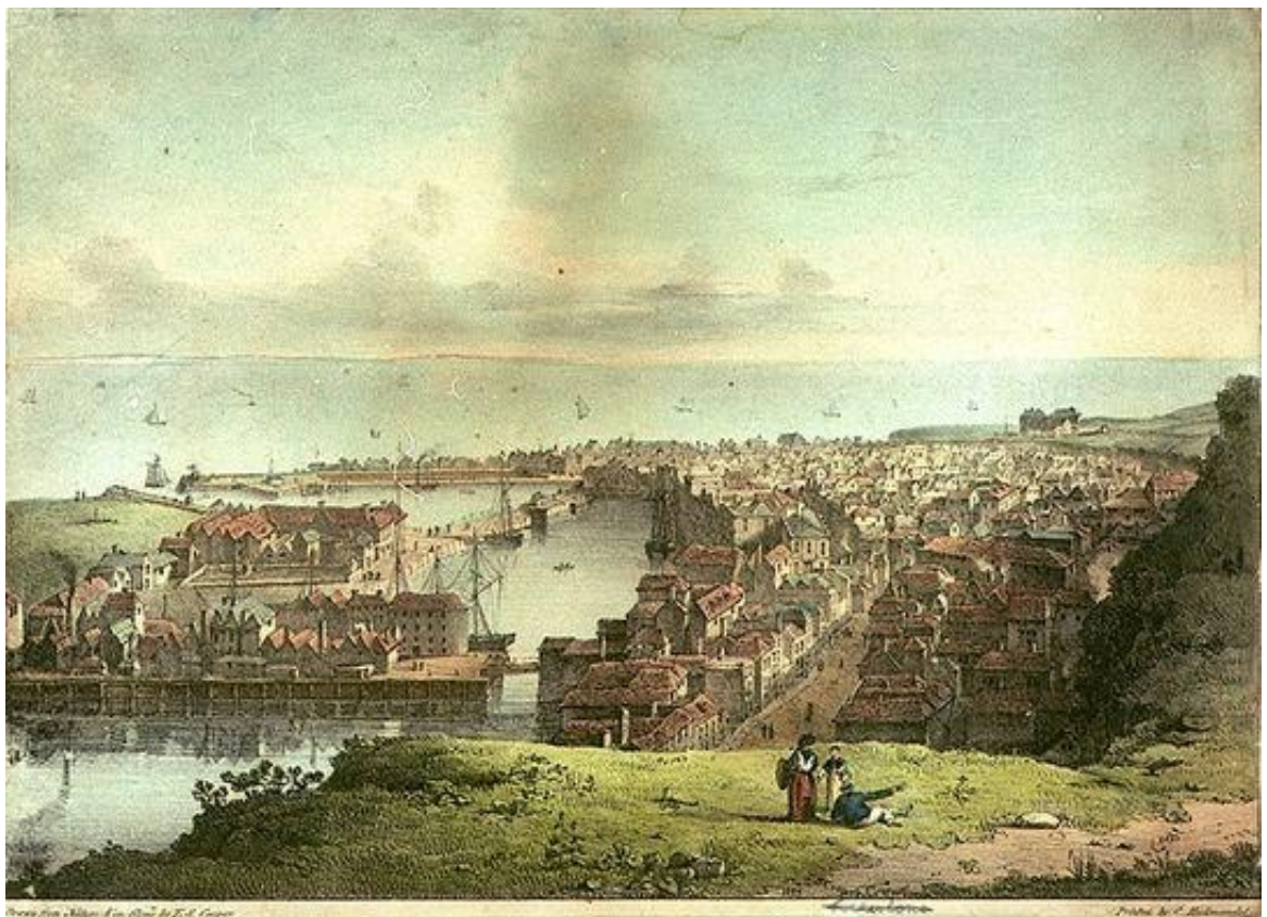
Figure 20, View of Dover Harbour looking south-west, 1825 (National Maritime Museum PUO 982)
