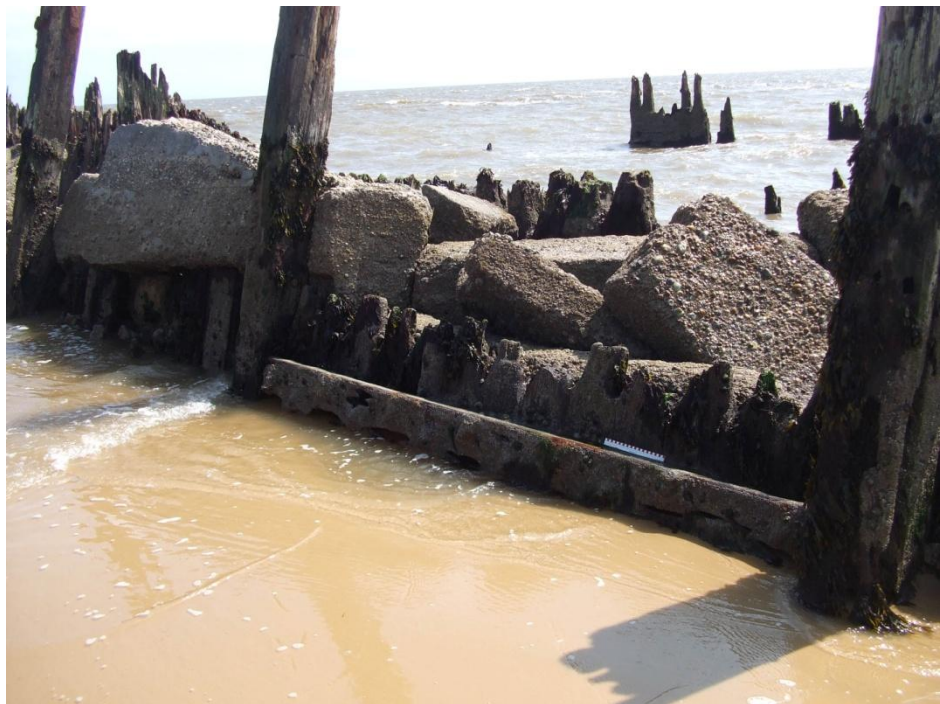
Figure 11, Detail photograph of the staggered projection to left side of photograph above. Angle driven main (tall) 300mm square piles, each spaced 3.50m apart. Close
