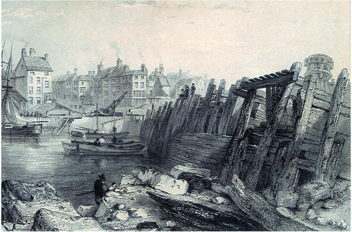
Figure 11, Inner face of the north pier in the early 19 th century showing lateral division within the pier (East Riding Museum Service)
