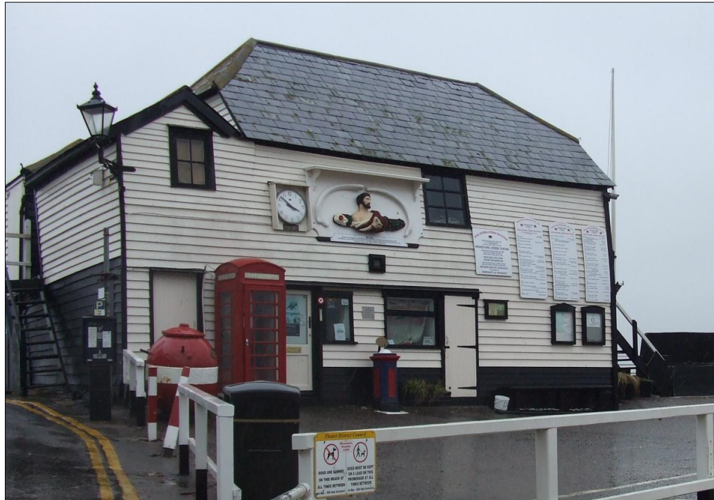
Figure 17, Look-out and Stores/Boathouse, looking East
