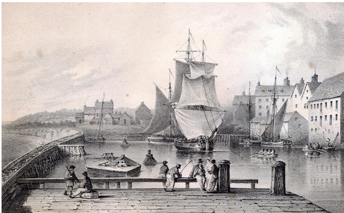
Figure 9, View of the south pier, looking west (East Riding Museums Service)
