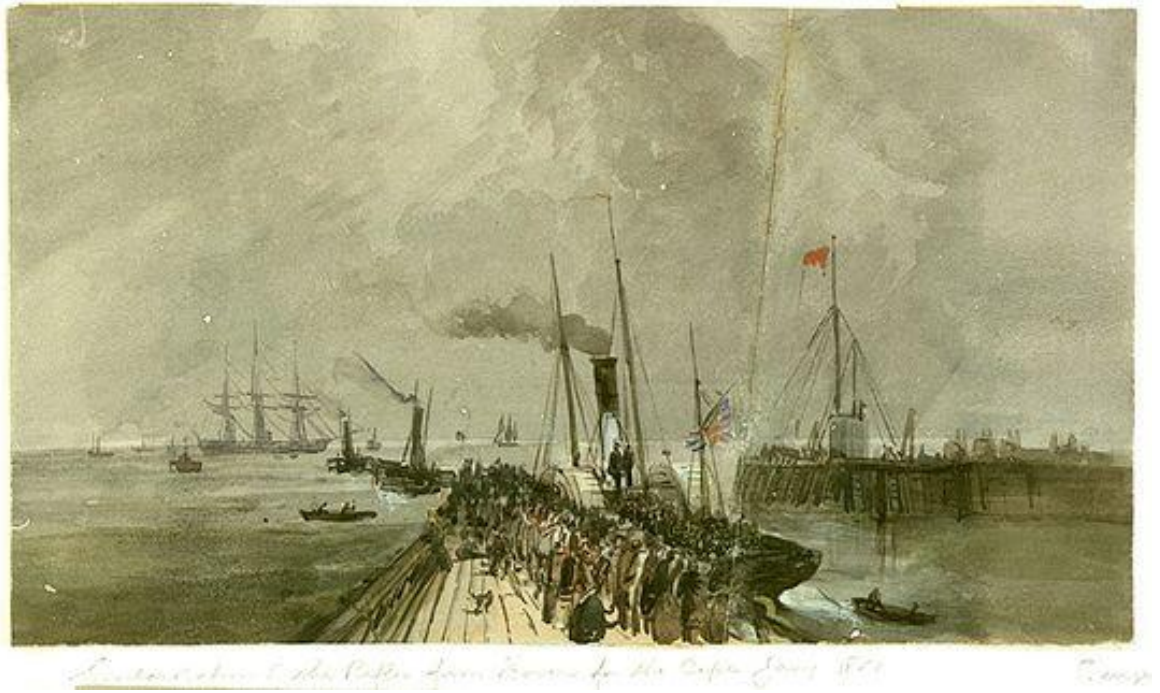
Figure 22, View of the pier heads at the entrance to Dover Harbour in 1851, looking south (National Maritime Museum PUO 982)
