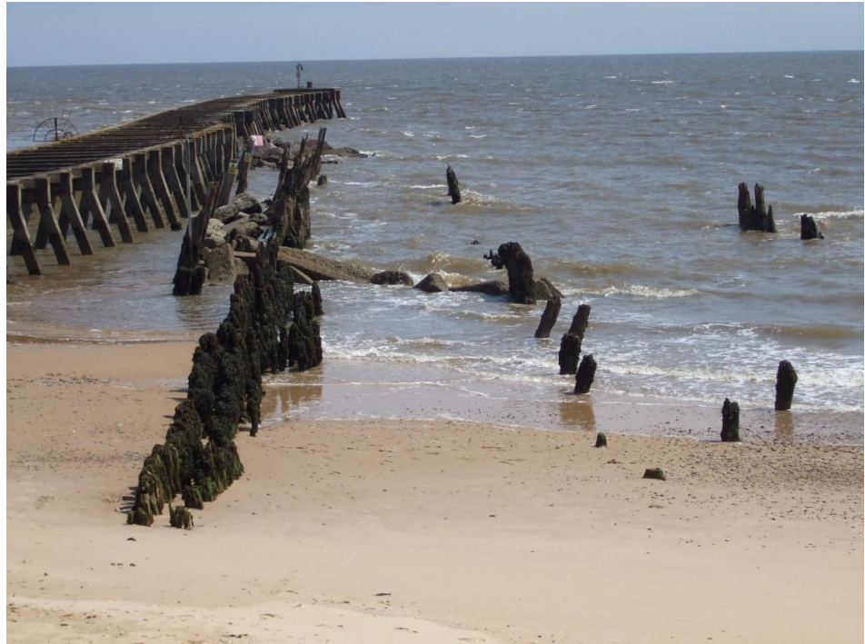
Figure 10, Remnants of the last of the timber south pier? (staggered line to left representing inner side and line of piles to right of this the outer side? Piles to extreme right may relate to piles to south of 1936 pier in old photograph above?)
