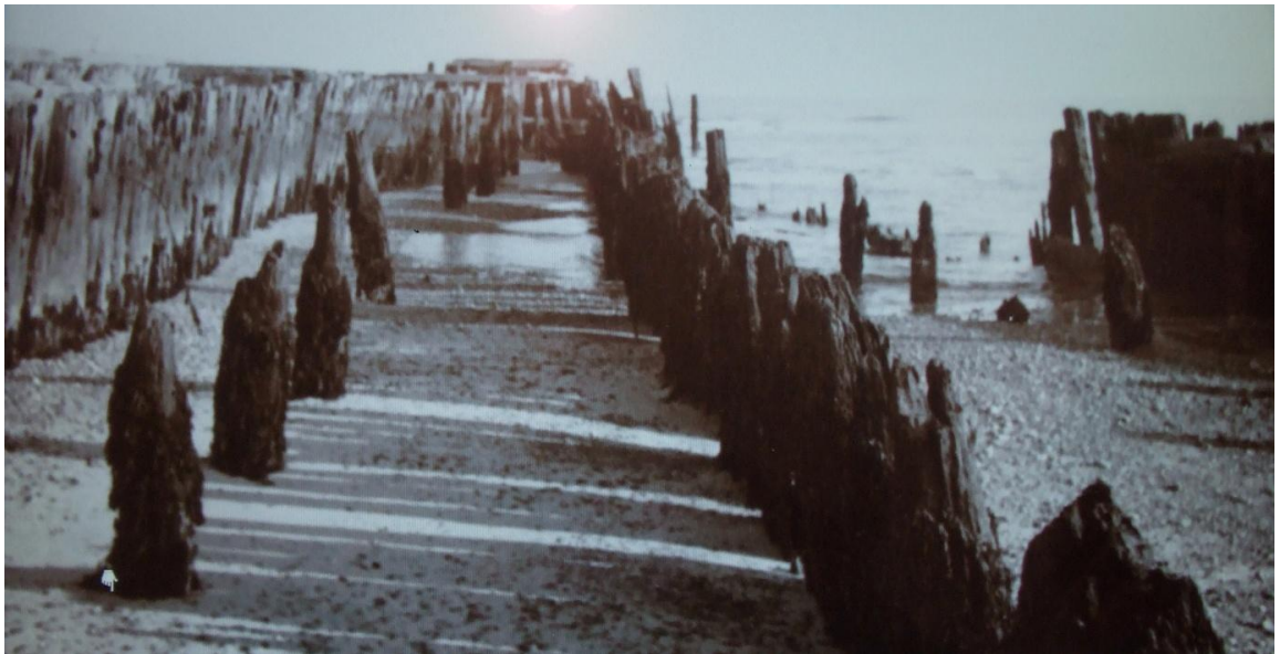
Figure 9, Last of the timber pier. Photograph of 1936 showing landward end of south pier with adjacent parallel pile alignments (Southwold Museum)
