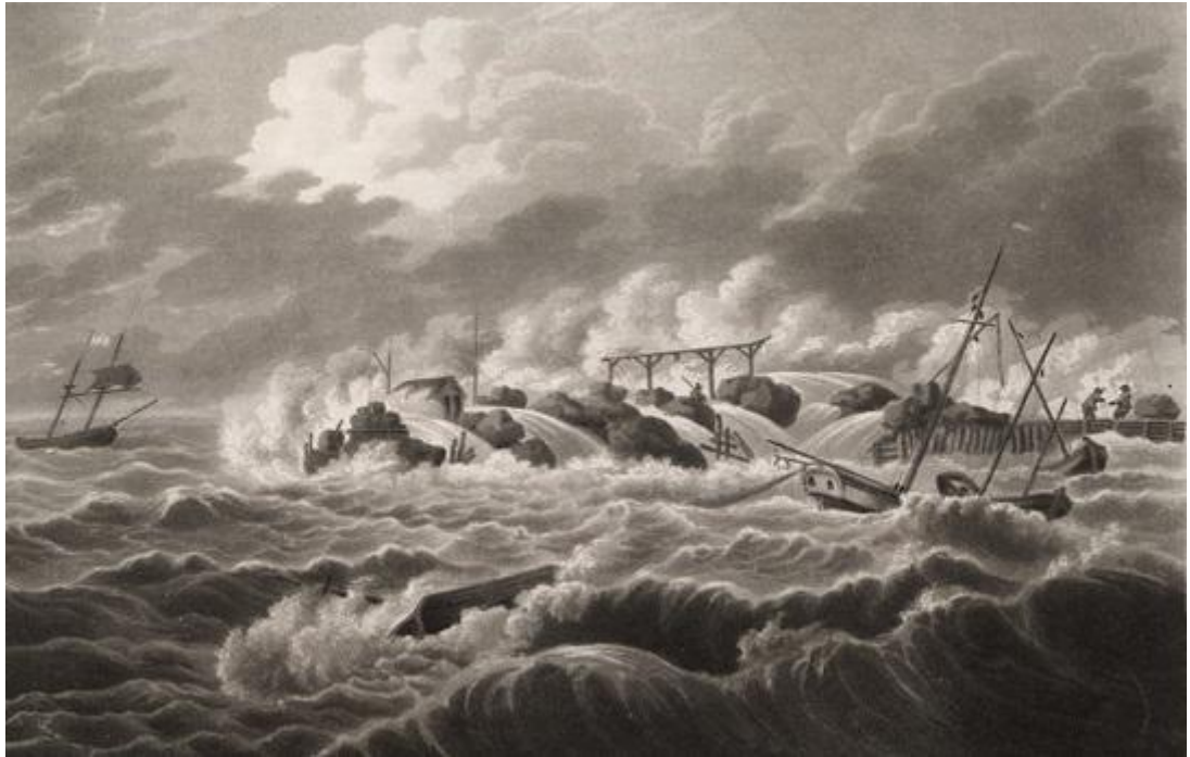
Figure 93, The stone clad pier at Margate destroyed by storm in 1808 (British Library, Ktop XVII 4-f-2)
