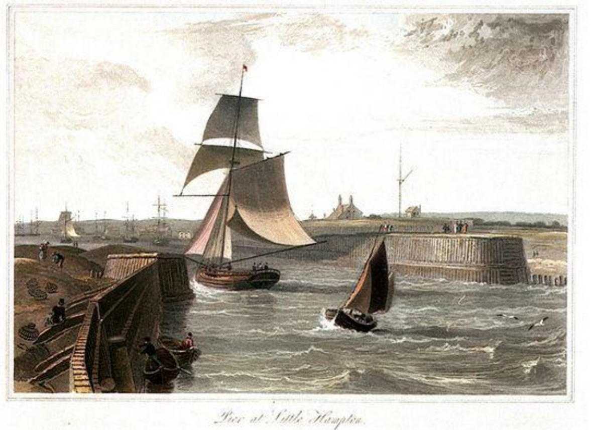
Figure 97, Piers at Littlehampton, 1823. Constructed of slightly angled close set piling with horizontal rails part way down the wall (National Maritime Museum: PU1052)
