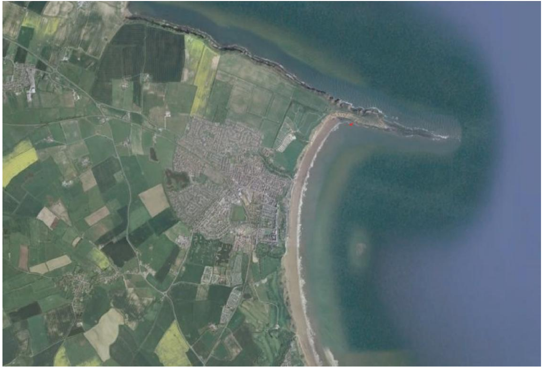
Figure 73, The setting of the pier remains at Filey (red) in relation to Filey Brigg and town (source: Google Earth)
