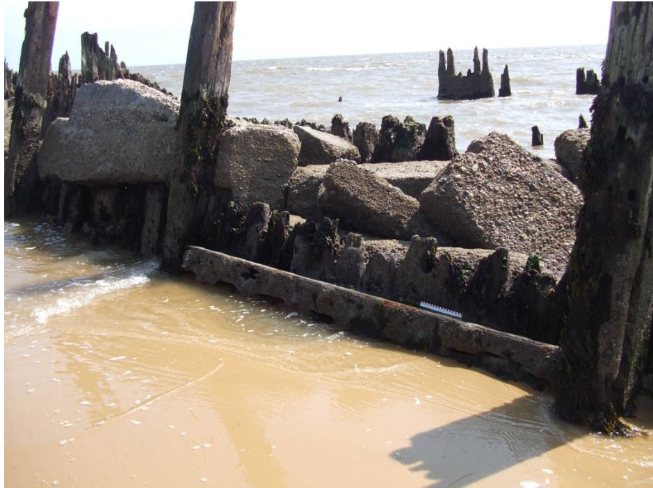
Figure 24, Photograph detail of extant pier remains, Southwold. In the foreground early 20 th -century work of the north side of the south pier at its point of junction with older pier remains behind. Tall angle driven main piles can be seen. Between these are edge to edge driven timber sheet piles bolted between ‘waling’ to front and rear. The large blocks behind are in fact concrete with that directly behind the timber being cast directly against it. Looking South-east
