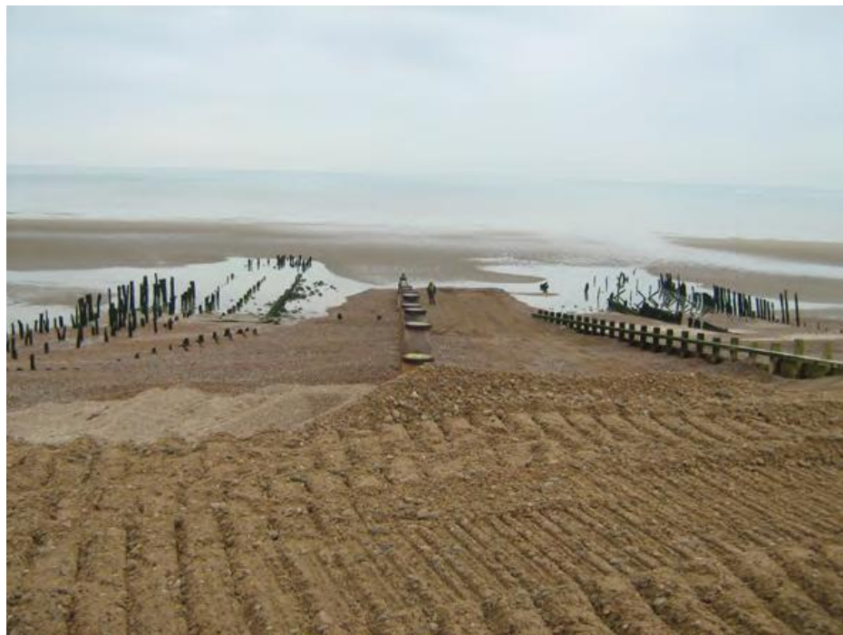
Figure 46, Rye. Photograph of the mouth of the 18 th -century harbour between two pier extensions of timber, looking south-east (later groynes also present) (Photograph reproduced from ASE 2008)
