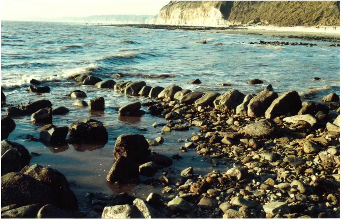
Figure 53, Part of the N.W. arm of Feature F3 at Flamborough – probable ‘rock armour’ for a pier toe. Remains of part of Feature F2 towards upper right. Looking south.
