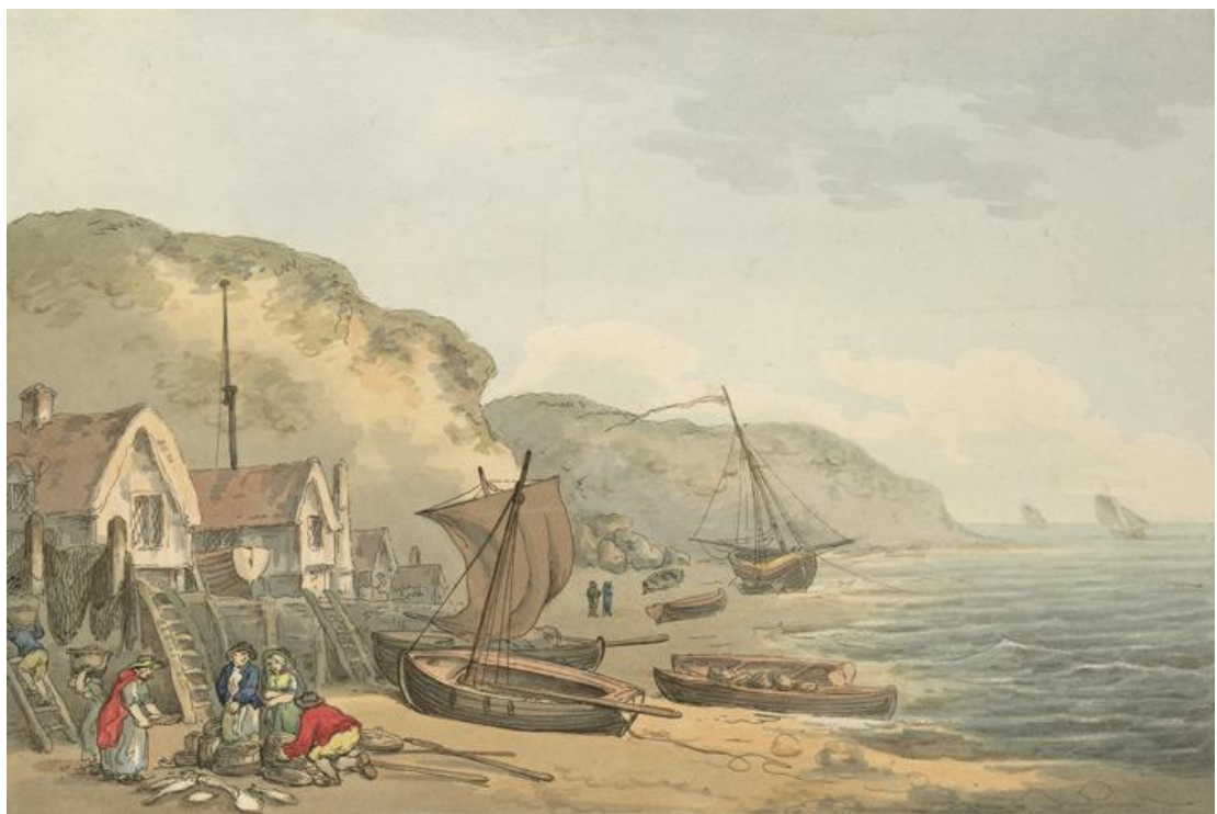
Figure 45, Folkestone. View near the Stade, looking east. Note the timber revetting work comprised of posts with horizontal planking behind. 1790 (British Library: kotp XVI, 55e)
