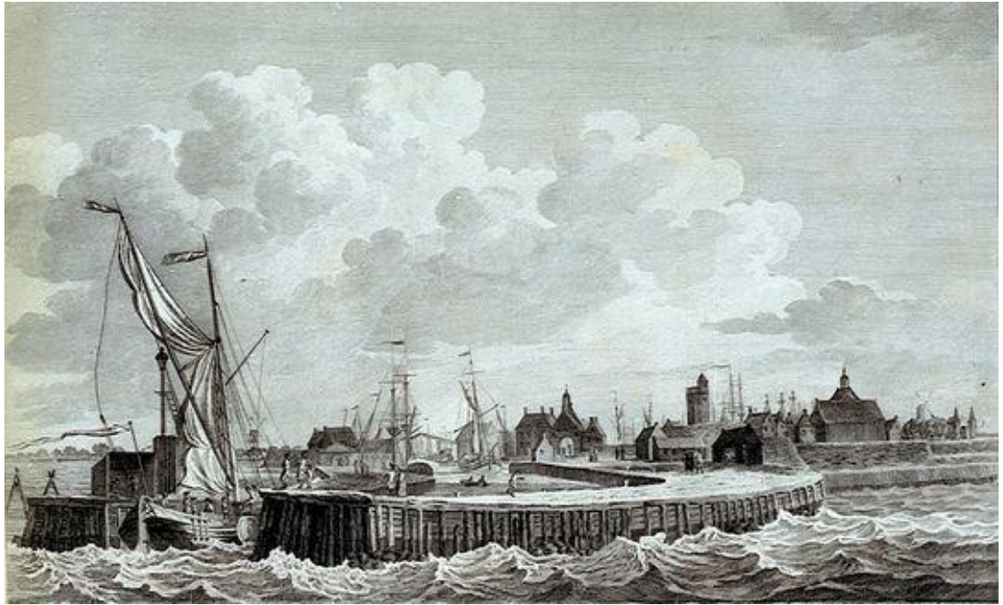
Figure 109, Twin piers at Harlingen, 1781. (National Maritime Museum, Greenwich: PW7388)
