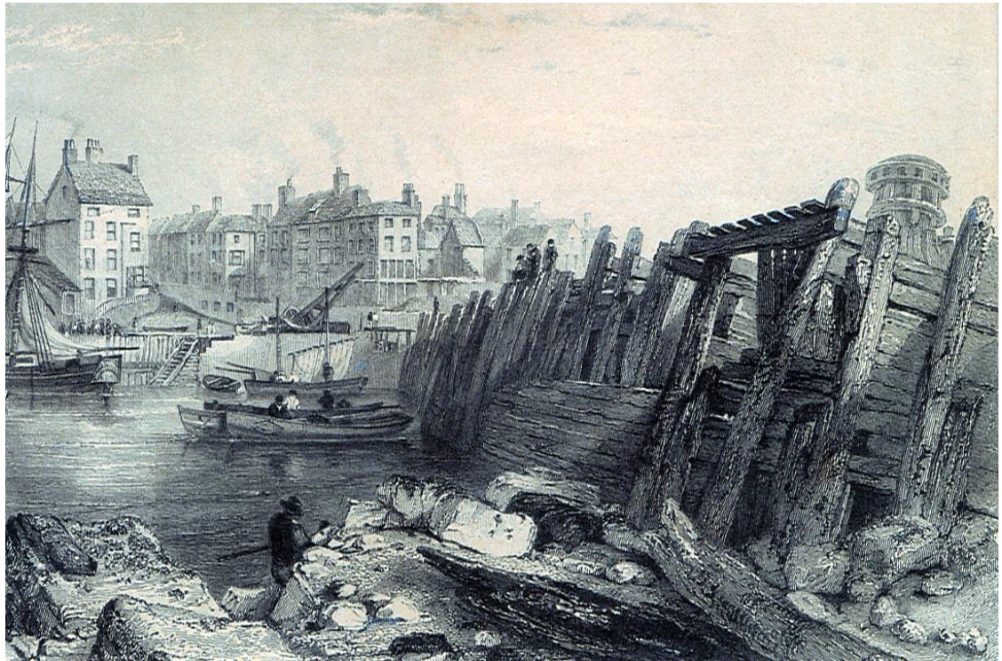
Figure 15, Inner face of Bridlington north pier in the early 19 th -century showing lateral division within the pier (East Riding Museum Service)
