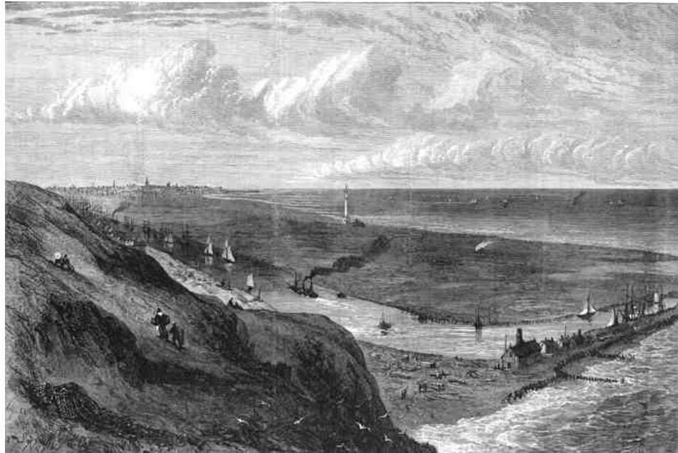
Figure 79, Topographic setting of Great Yarmouth haven, 19 th -century. The River Yare flows between the mainland and spit, turning sharply to reach the sea between the piers. The spit south of the haven had long disappeared by this date and groynes had been placed to prevent further erosion. (Norfolk Online Access to Heritage website)
