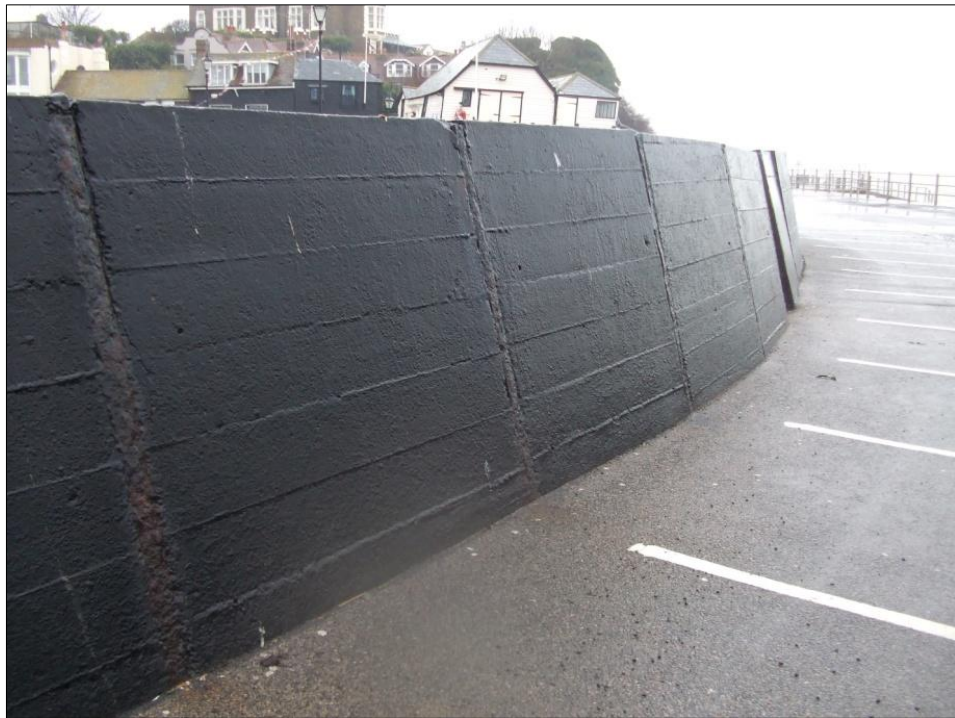
Figure 33, Broadstairs. Photograph detail of elevated walling (in position of former outer face of pier) now in concrete
