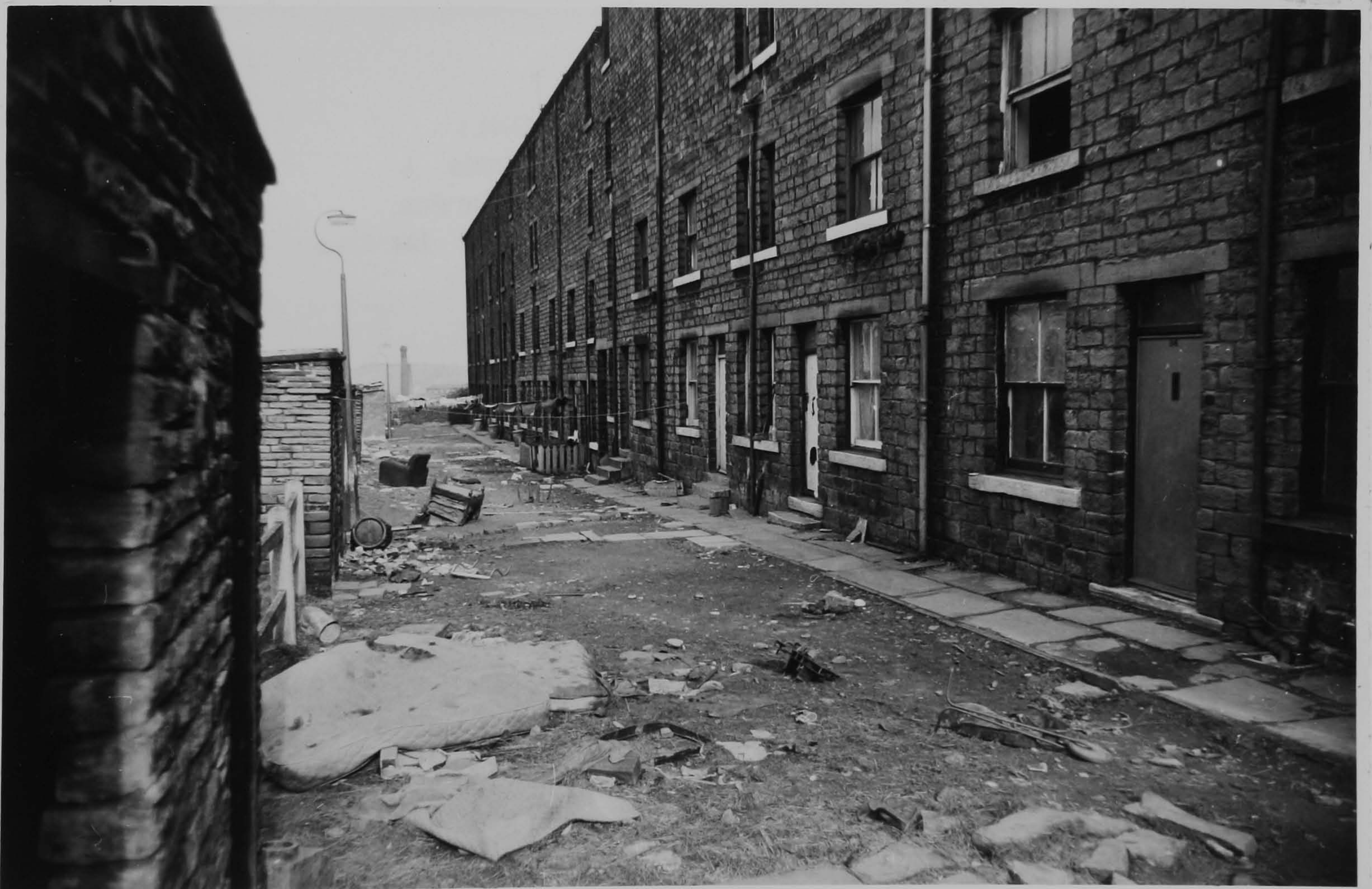
16. Back Orchard St (1968) The bottom portion of a terrace built on 999-year leases from Lockwood Proprietors in early 1880s boom. There are of back-to-back houses.
