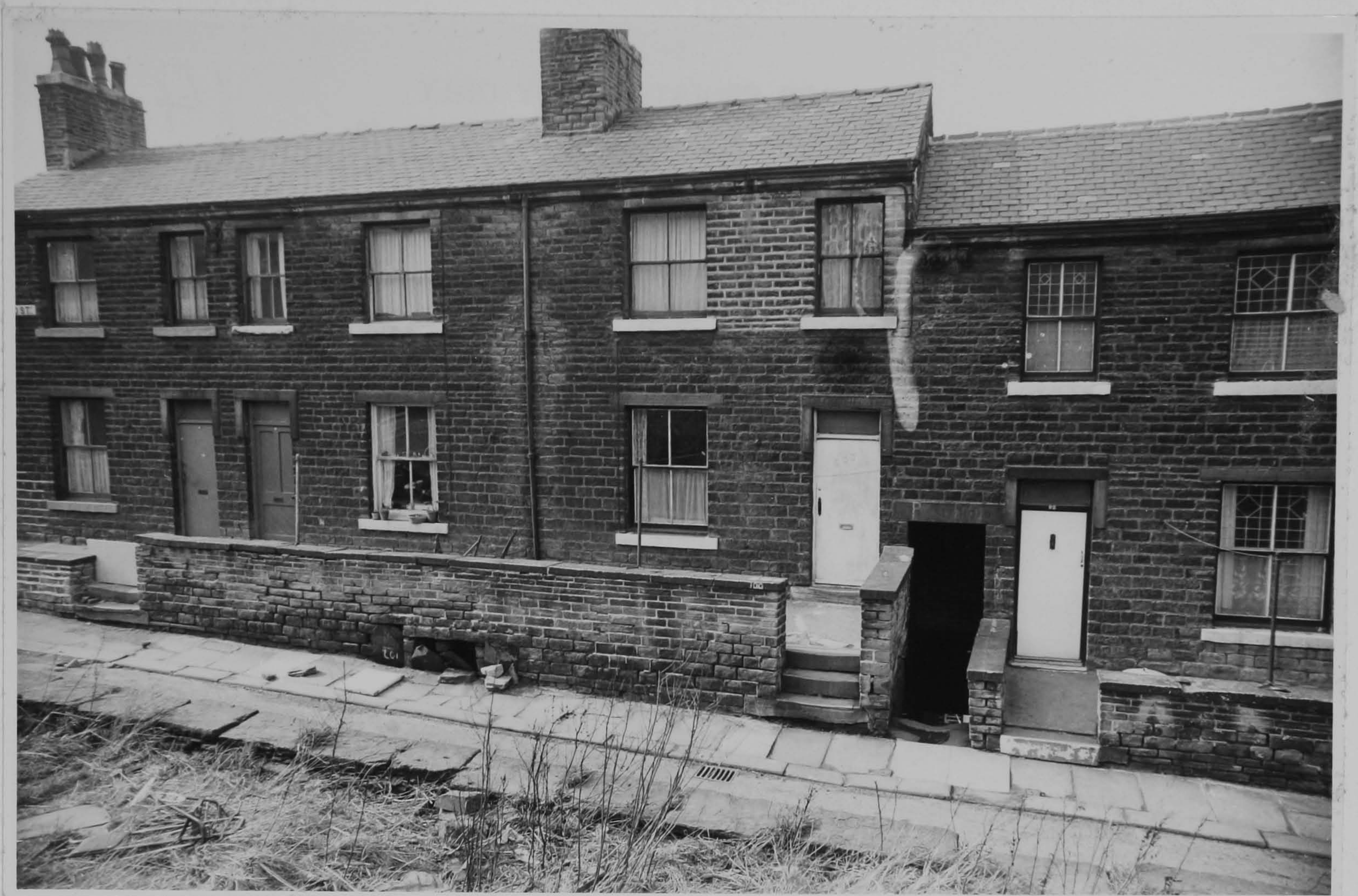
15. Orchard St (1968) The top position of terrace of back-to-back houses built on Lockwood Proprietors land. A tunnel every 4 houses conformed with byelaw regulations.
