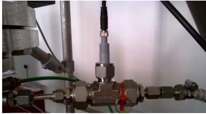
Figure 4.8 The photo of T-type tube fitted with the humidity sensor
