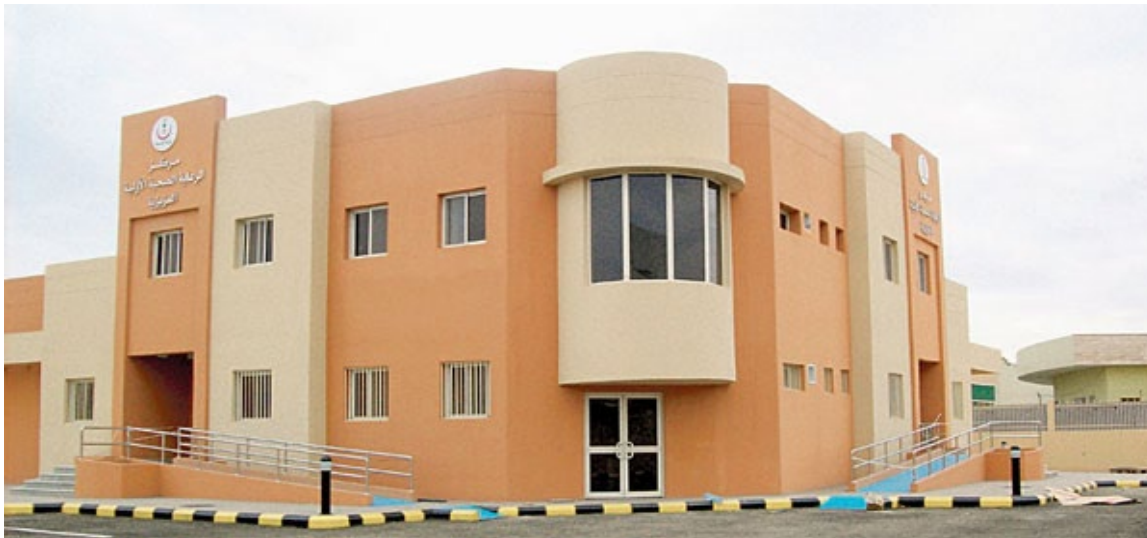
Figure 5.2 Exterior view of one of the PHCCs in SA
