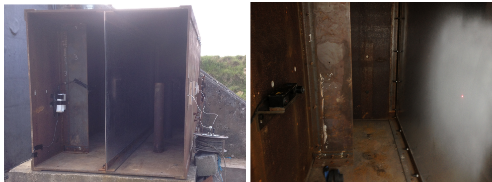
(a) Panel in position along centre of box
