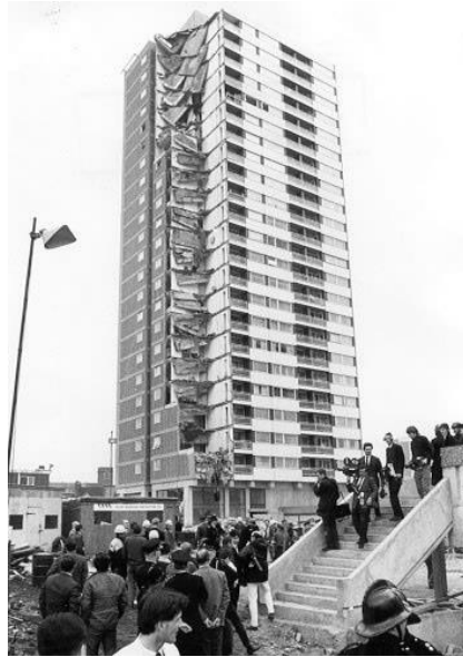
Figure 2-1 Ronan Point building after the May 1968 collapse [22]
