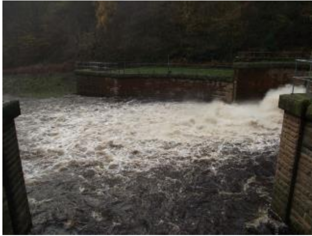
Figure 3-4. The stilling basin at Digley Reservoir during a release. Water is discharged at high pressure out of the pipe (right hand side of image) with considerable force, again oxygenating the water as seen in the later results sections.
