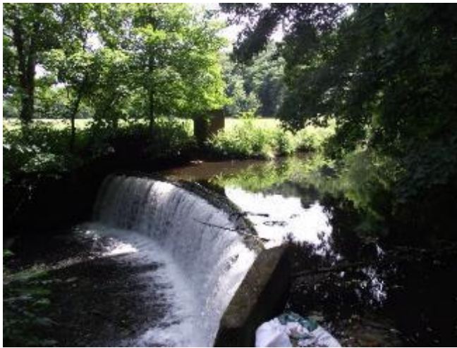
Figure 3-3. Photo of a weir on the River Holme. Numerous weirs such as this act to oxygenate the water as it flows downstream and maintain high river stage.
