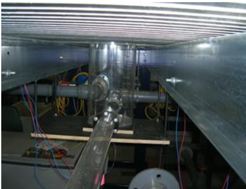
Figure 25 - Main pipe (branch A) First manhole (downstream view)
