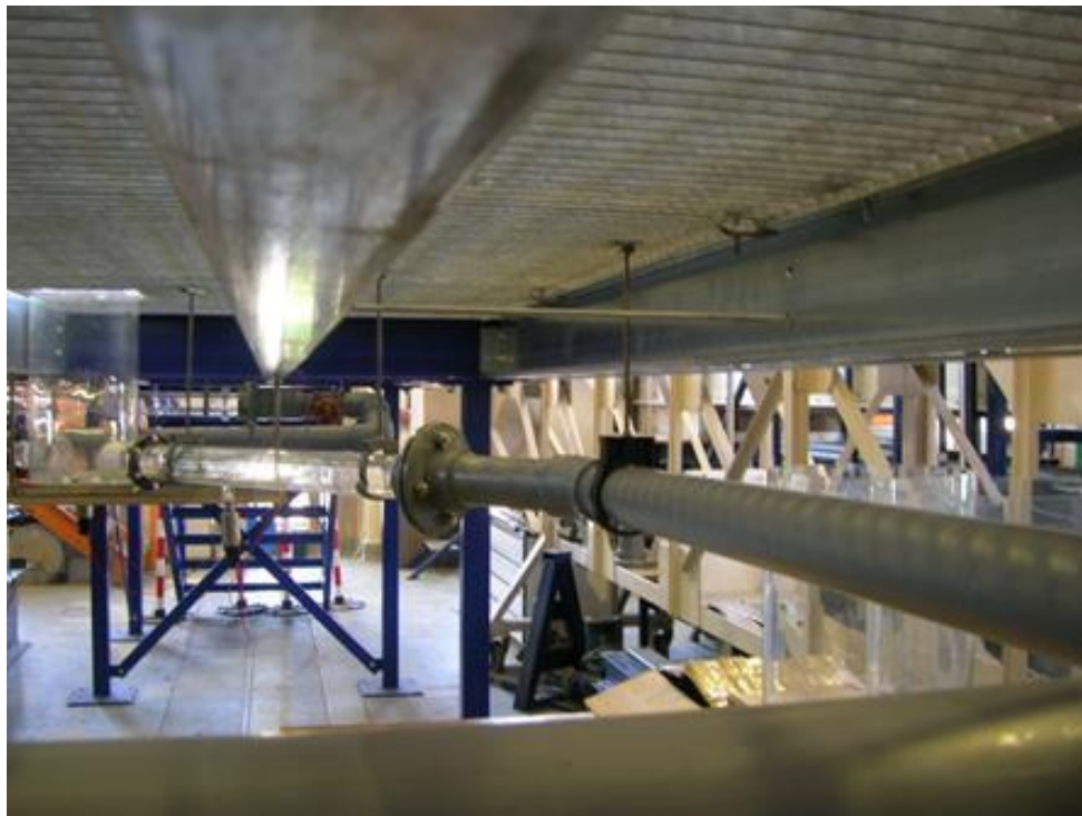
Figure 27 - Branch "C" (upstream view)
