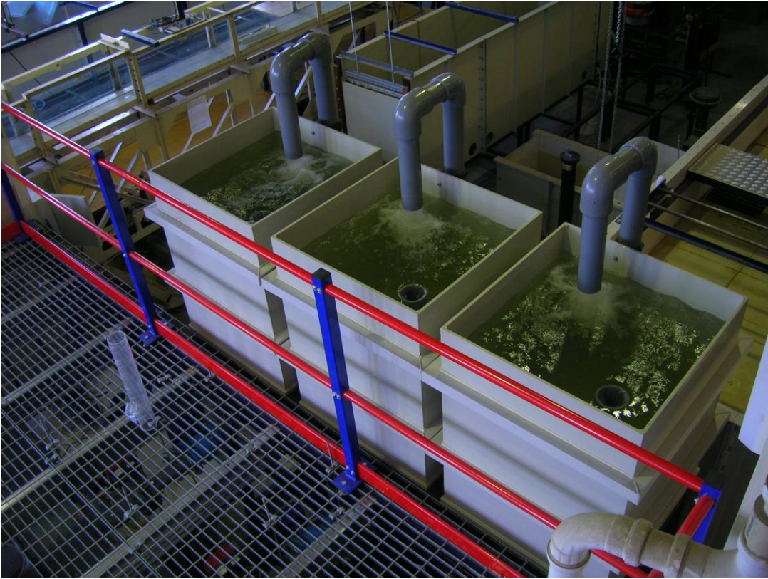
Figure 32 – Particular detail of the three tanks being filled with water.
