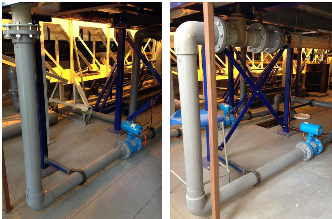
Figure 48 - “T” connection utilized for pipe downstream urban surface as well as sewer system.
