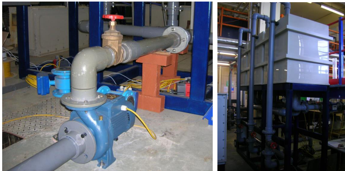
Figure 31 – Particular detail of the pump (left) used to fill the three feeding tanks (right).
