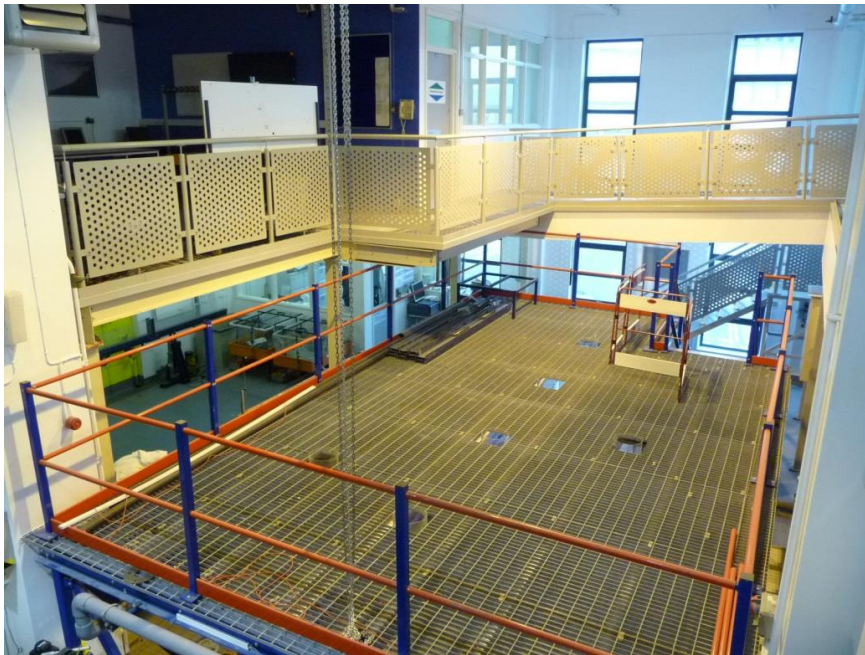
Figure 28 - Birdseye view of the whole system prior the construction of the urban surface (from “upstream”).
