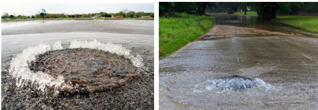
Figure 2 – Examples of system surcharge and exceedance flow generation. Left) Central Texas, Herald/TJ MAXWELL, Right) Waynesville, Aug. 9, 2013 Steve Zumwalt/FEMA
