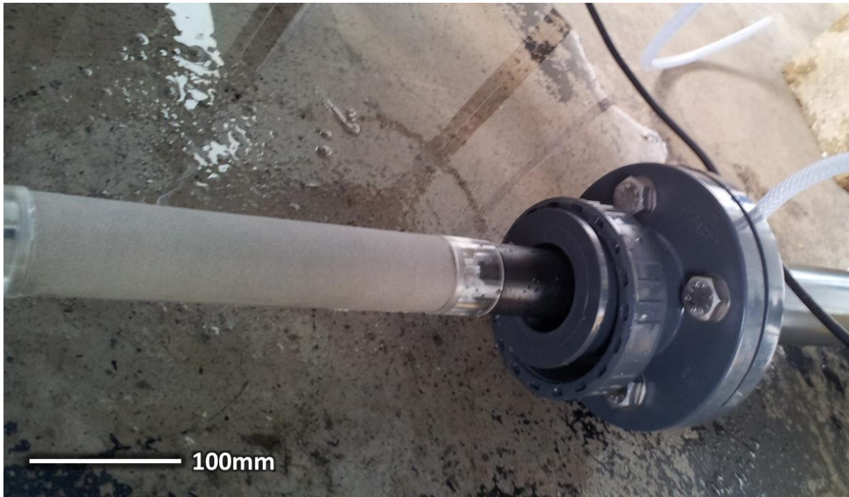
Figure 12: A photograph of the ozone dosing lance fitted into the corporation cock ready for insertion into the column.
