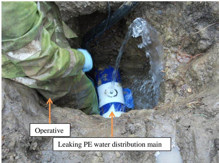
Figure 1-14 Tapping-tee failure causing leak to mains pipe
