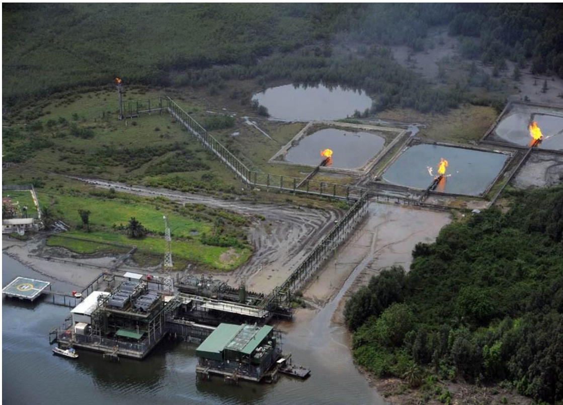
Figure 7.2: Gas flaring in Rivers state (Source National Post, April 5 2013)
