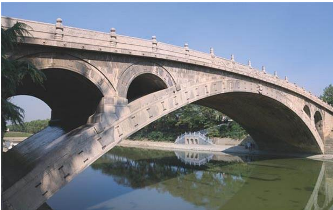
Figure 2.8: An example of stress arching in building construction (Zhaozhou Bridge in China).
