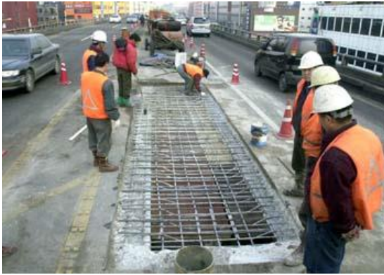
Figure 1.5 A maintenance work to fill a large pot hole (Source: http://blog.donga.com/laputa4/archives/4 )
