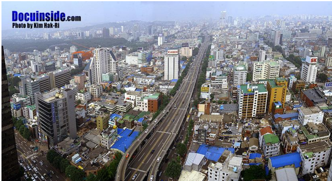
Figure 6.15 CGC Street and CGEH before the restoration project (source: http://www.docuinside.com )
