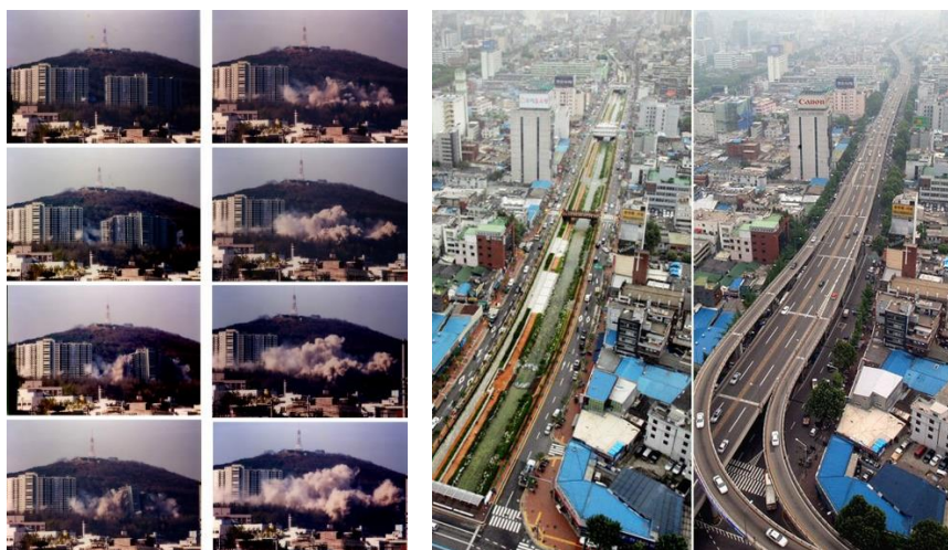
Figure 6-2 (left) The series of images of demolition of the Foreigner's Apartments in Namsan Mountain in 1994. The demolition was live streamed across the country (Source: http://blog.naver.com/photok1/150080462861 ); (right) After and before the Cheonggyecheon Stream Restoration Project, which remove 5.8km of the elevated highway and restore the stream. This restored stream now attracts an average of 64,000 visitors daily, of those about 1,400 are foreign tourists (Source: Seoul Metropolitan Government: http://www.seoul.go.kr/ ).
