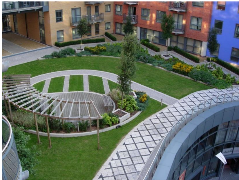
Figure 1.2: Typical semi-intensive green roof located on Sharrow School, Sheffield, UK. Substrate depths vary from 60-300mm. Photo by Jeff Sorrill, University of Sheffield.
