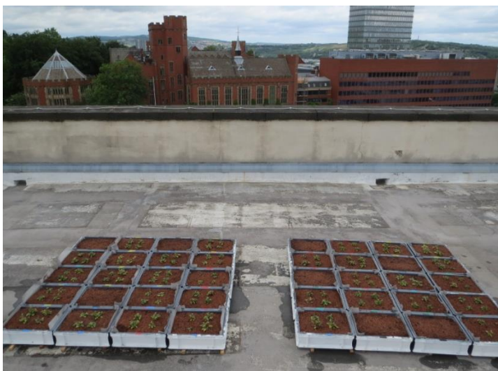
Figure 4.2: Installed green roof modules with Prunella vulgaris plugs planted
