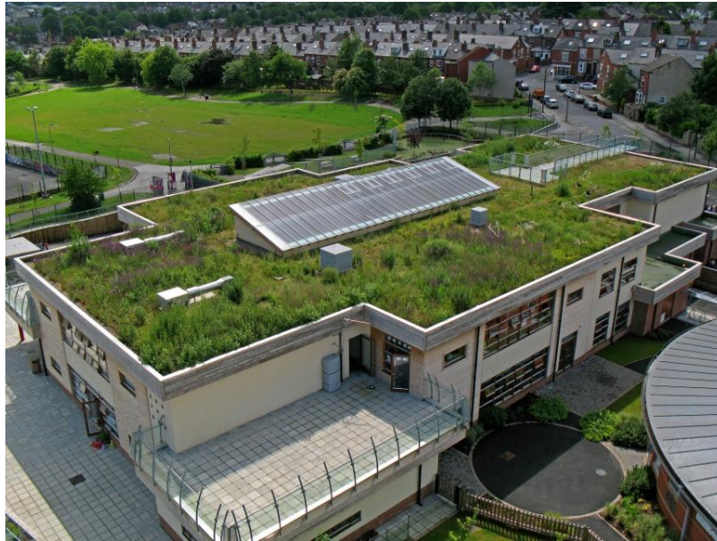
Figure 1.2: Typical semi-intensive green roof located on Sharrow School, Sheffield, UK. Substrate depths vary from 60-300mm. Photo by Jeff Sorrill, University of Sheffield.
