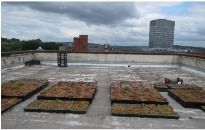
Figure 4.1: View of the test site on the 9 th storey of the Education Building, University of Sheffield.
