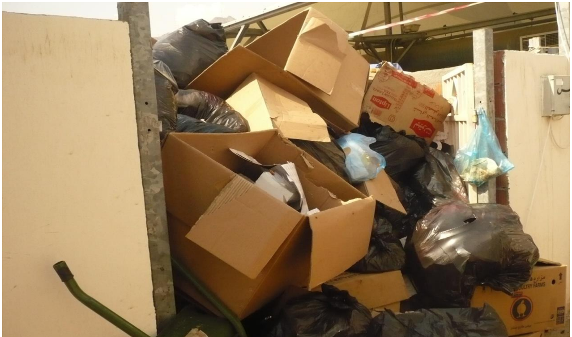
Figure 1-22 Compactor box is buried under the waste pile, which prevent the access to the switches
