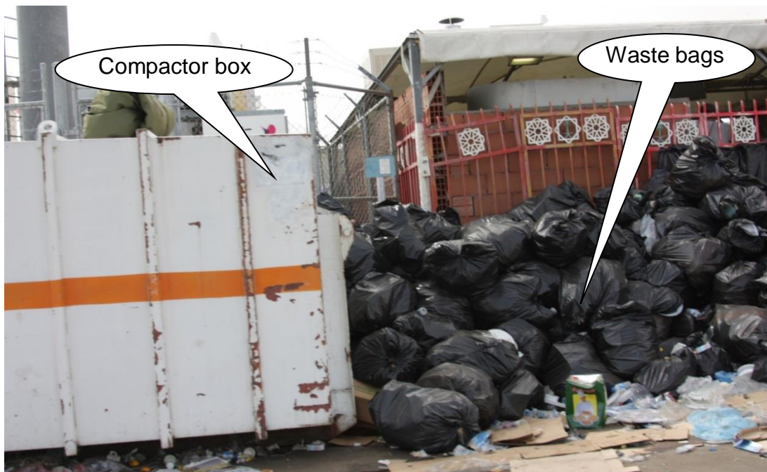
Figure 4-5 The method of collecting waste in the compactor box, where waste is collected in waste bags and disposed of in the compactor box
