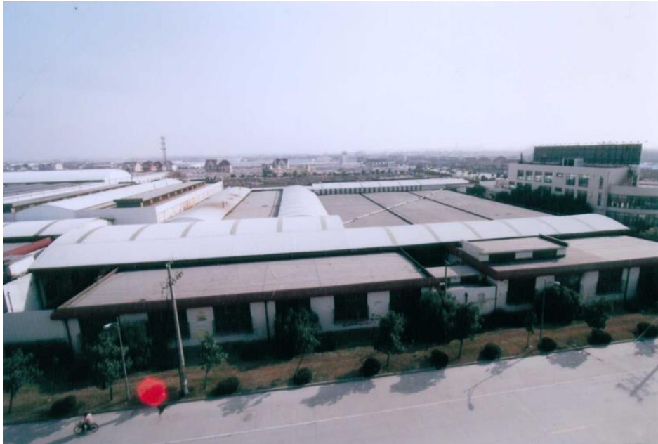
Figure 7.2 Urban villages of this nature are characterised by a mixture of land use: factories, farmland and scattered villages. The buildings in this photograph were demolished as part of the Hongqiao redevelopment
