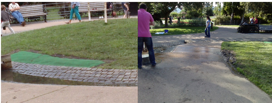
Photograph 21: Big muddy area and temporary solution on the left, and problem with muddy area and water features on the right (August 2013 - taken by the author)
