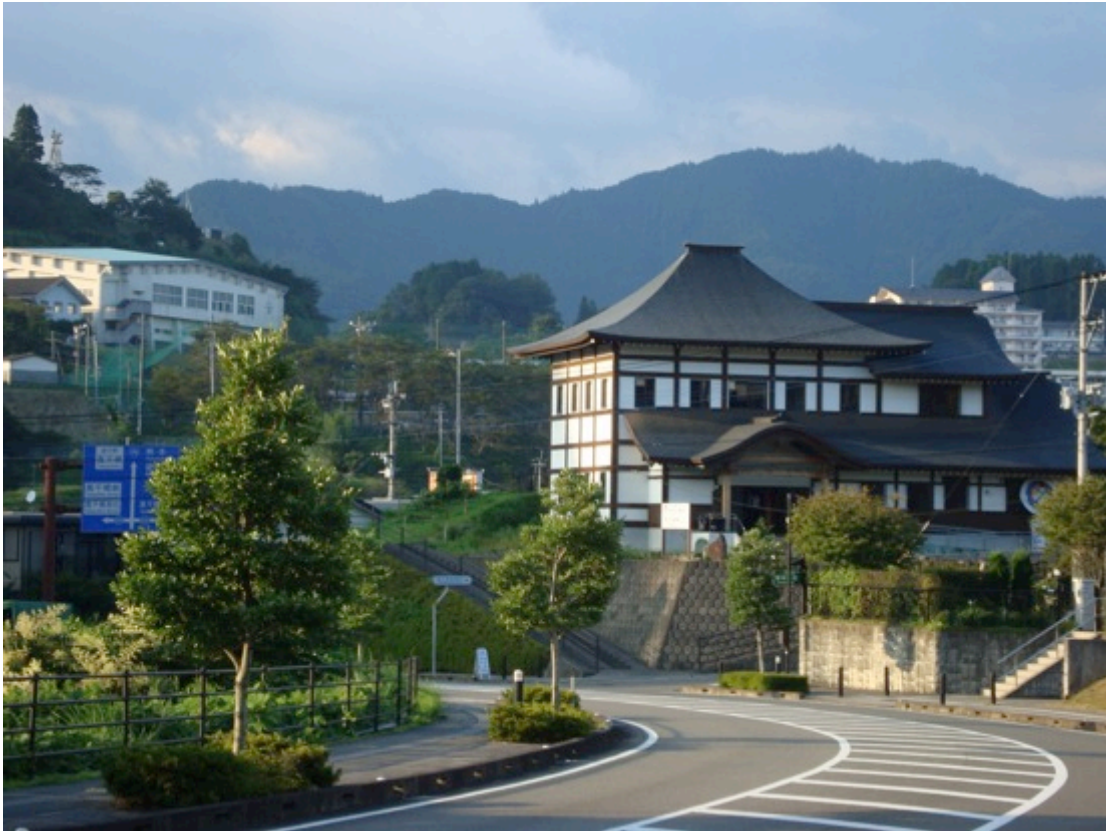
Figure 6.3 The newly built temple in town (opposite Takachiho shrine)
