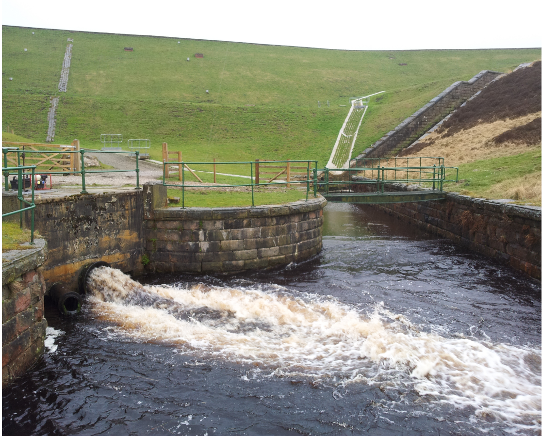
Figure 5.15: Artificial Flood in progress at reservoir C.
