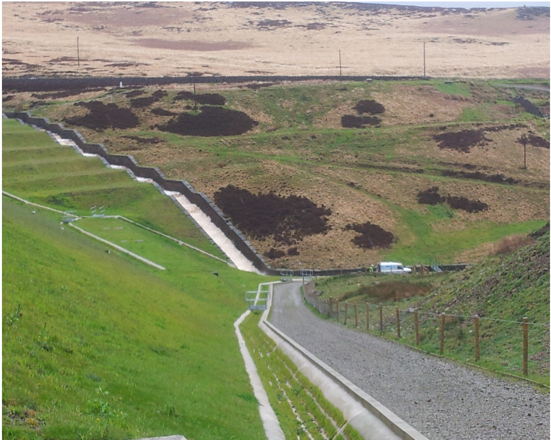
Figure 5.14: Water cascading down spillway at reservoir C.
