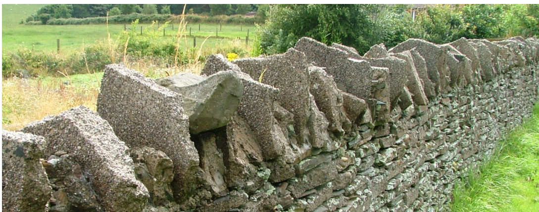
Figure 32: Wall along main driveway at Knockaloe. Constructed of concrete rafts from the camp. ©
