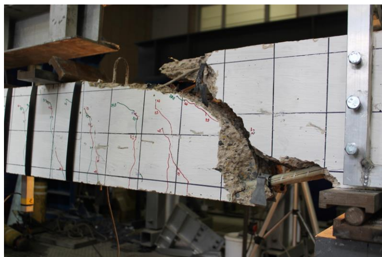
Figure 4-8 Diagonal tension failure of GB50-P150
