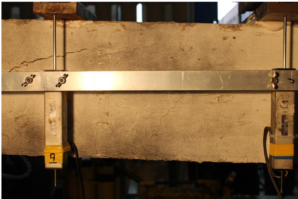
Photo from the back of the beam
