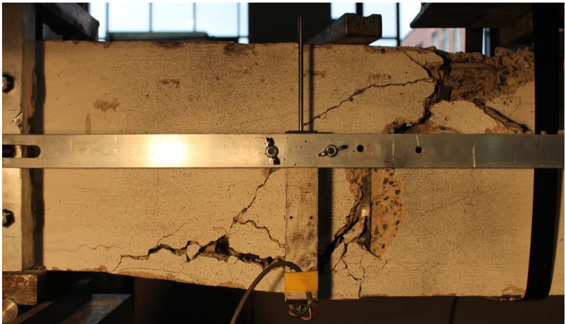
Photo from the back of the beam
