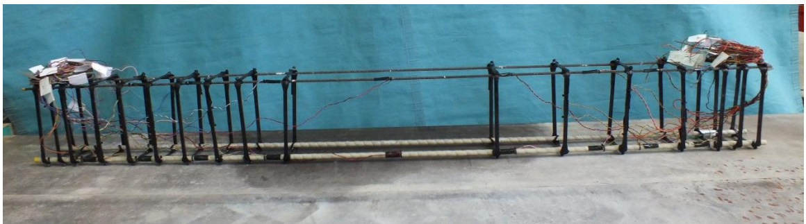
Figure 3-6 Reinforcement cage for beam CB51
