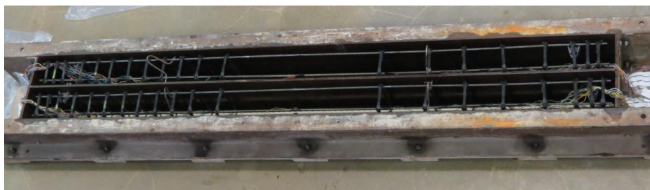
Figure 3-7 Beams ready for casting
