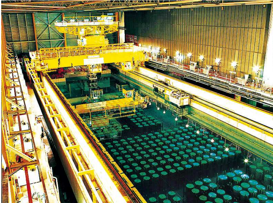
Figure 1.5: Nuclear fuel storage tanks prior to the reprocessing process, courtesy of Sellafield Ltd.
