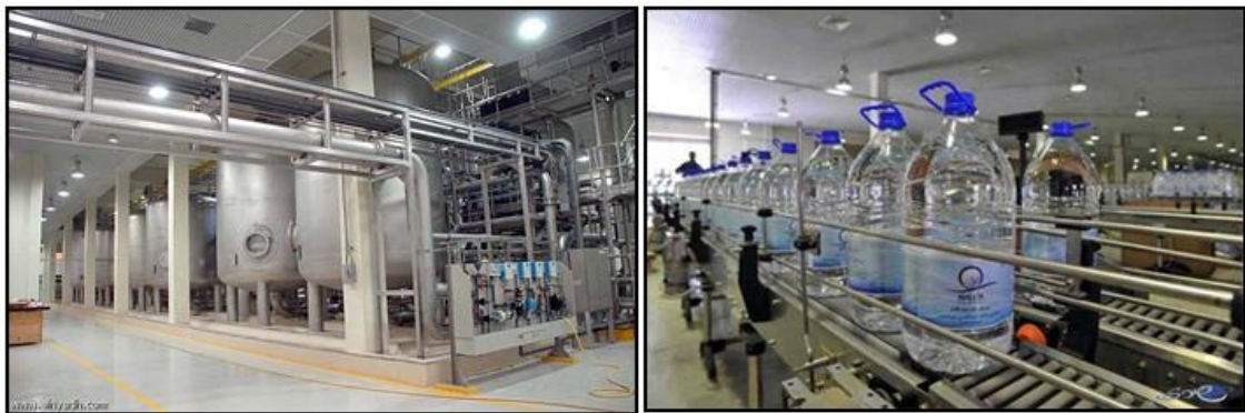
Figure 3. 13: Zamzam water bottling plant
