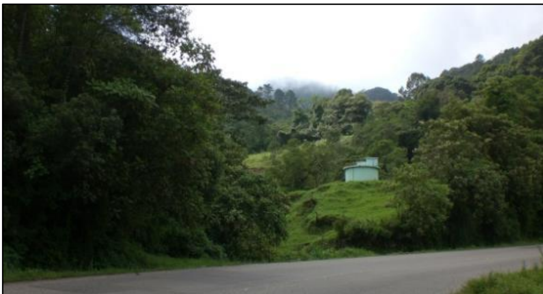
f) Las Flores community water tank located near the international highway.
