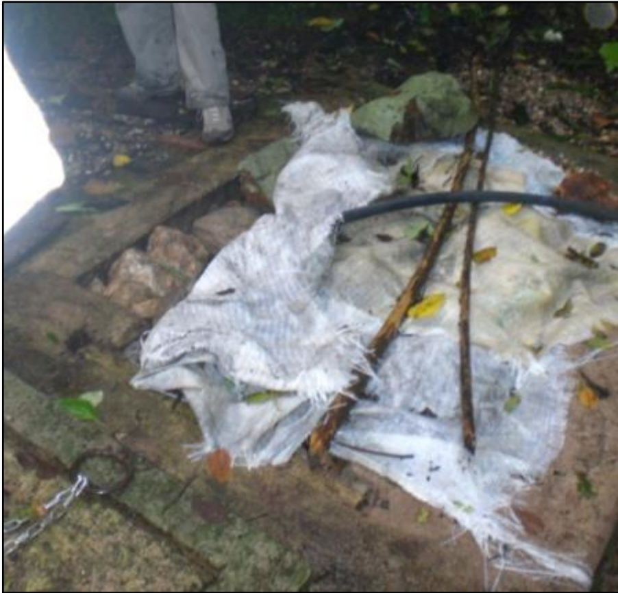
e) La Granadilla community box-style water source with stone filter covered by sack cloth.
