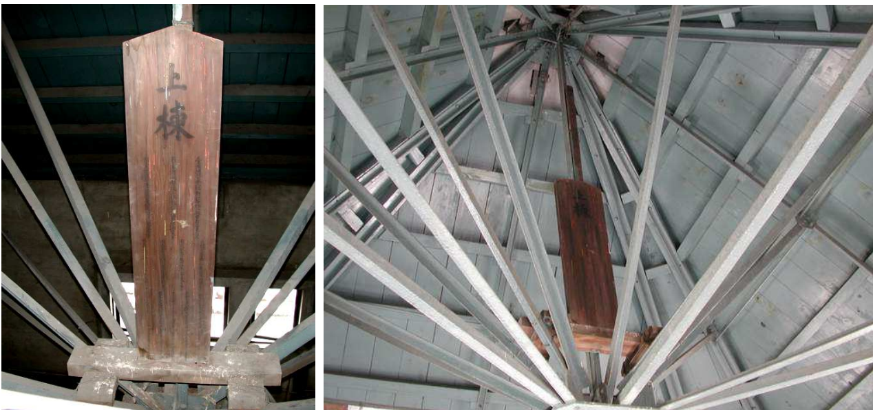
5.70. and 5.71. Cypress tablet for beam raising ceremony. (Courtesy of C. Y. Li Architecture & Engineers)
