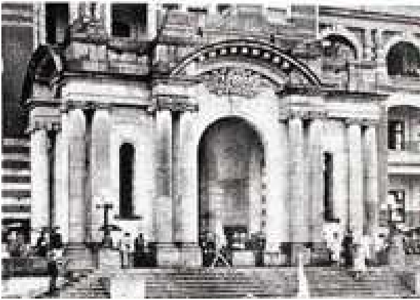
5.57. Official entrance Portico. Source from Huang, J., 2004.
