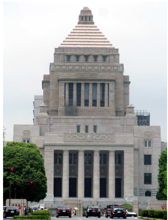
5.99. The Imperial Diet Building's tower, Tokyo. (Photography by Author)
