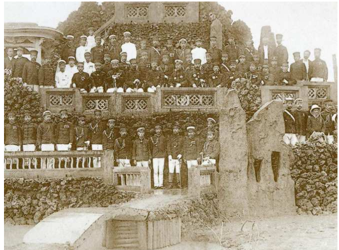
4.1. Japanese Officials within the rock garden at the Old Taiwan Governor-General's Office, formerly the Taiwan Provincial Administration Yamen. Source from Shue and Huang, 2003.
