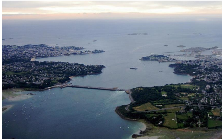
Figure 1-14 - La Rance Tidal Barrage, France [26].
