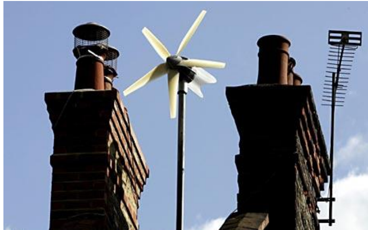
Figure 1-10 – Inappropriately-located wind turbines damage public opinion and may never repay the energy used in their manufacture.
