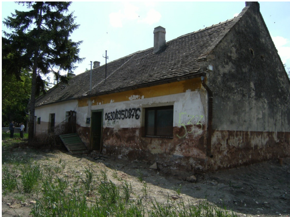
Figure 2.9 - Digital photograph of house in Devecser awaiting demolition (May 2011)
