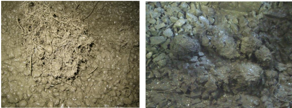
Figure 2.10 Fibre balling in concrete
