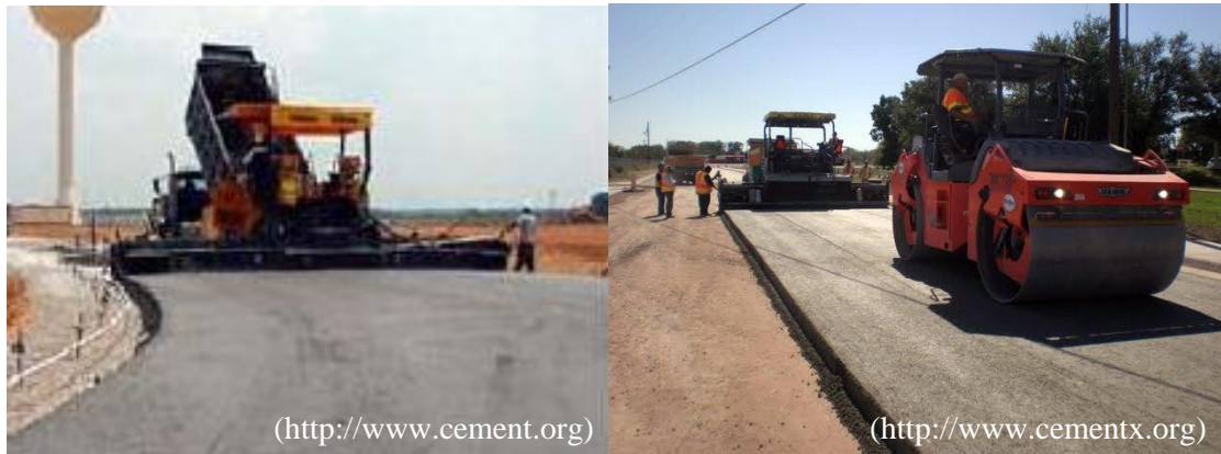
Figure 1.3 (a) Placing RCC; (b) Compacting RCC
