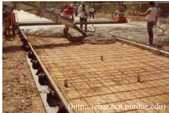
Figure 1.4 Placing CC for reinforced concrete pavements
