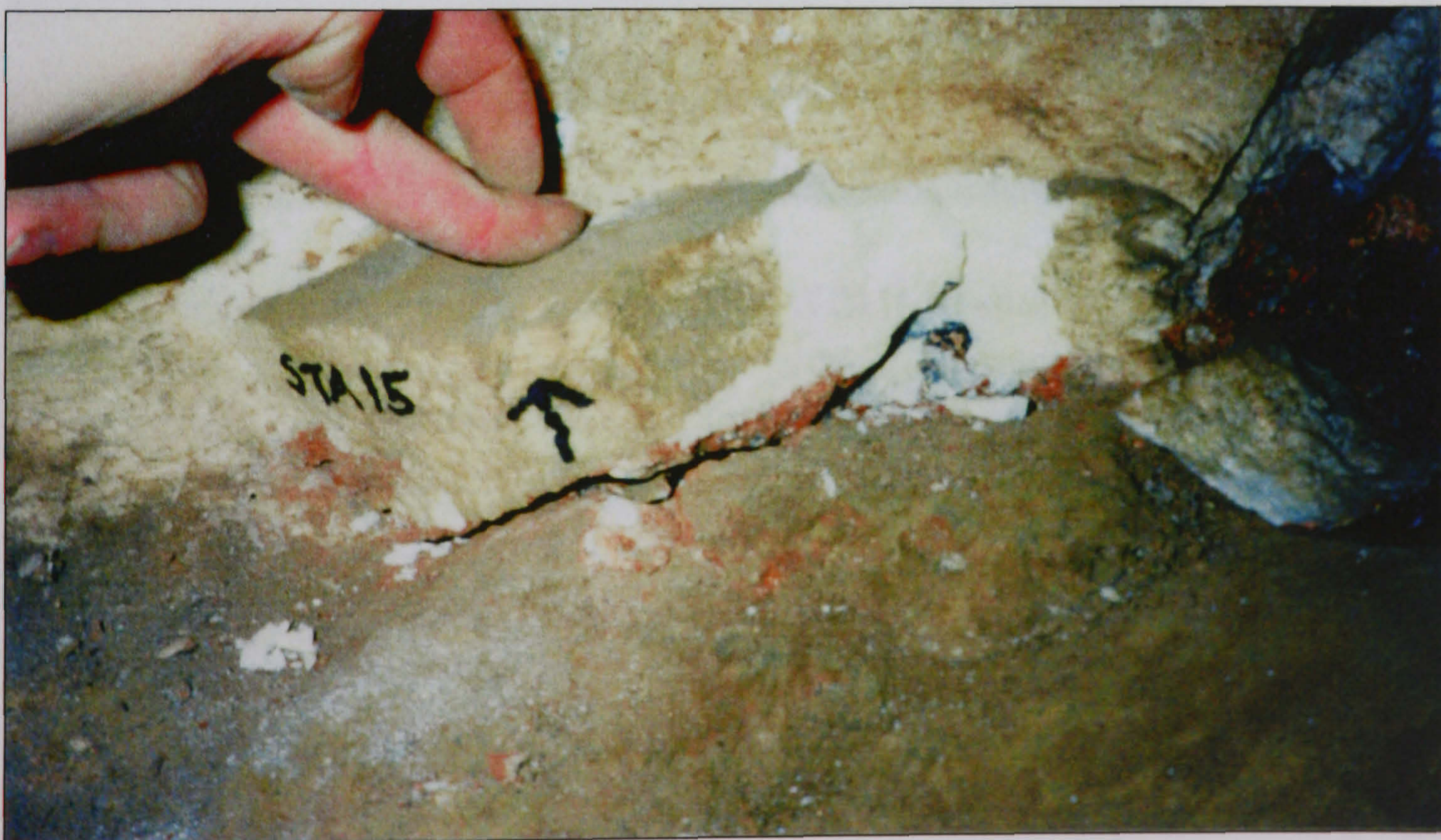
Figure A.12: Photograph of sample STA15 in situ, after removal.
