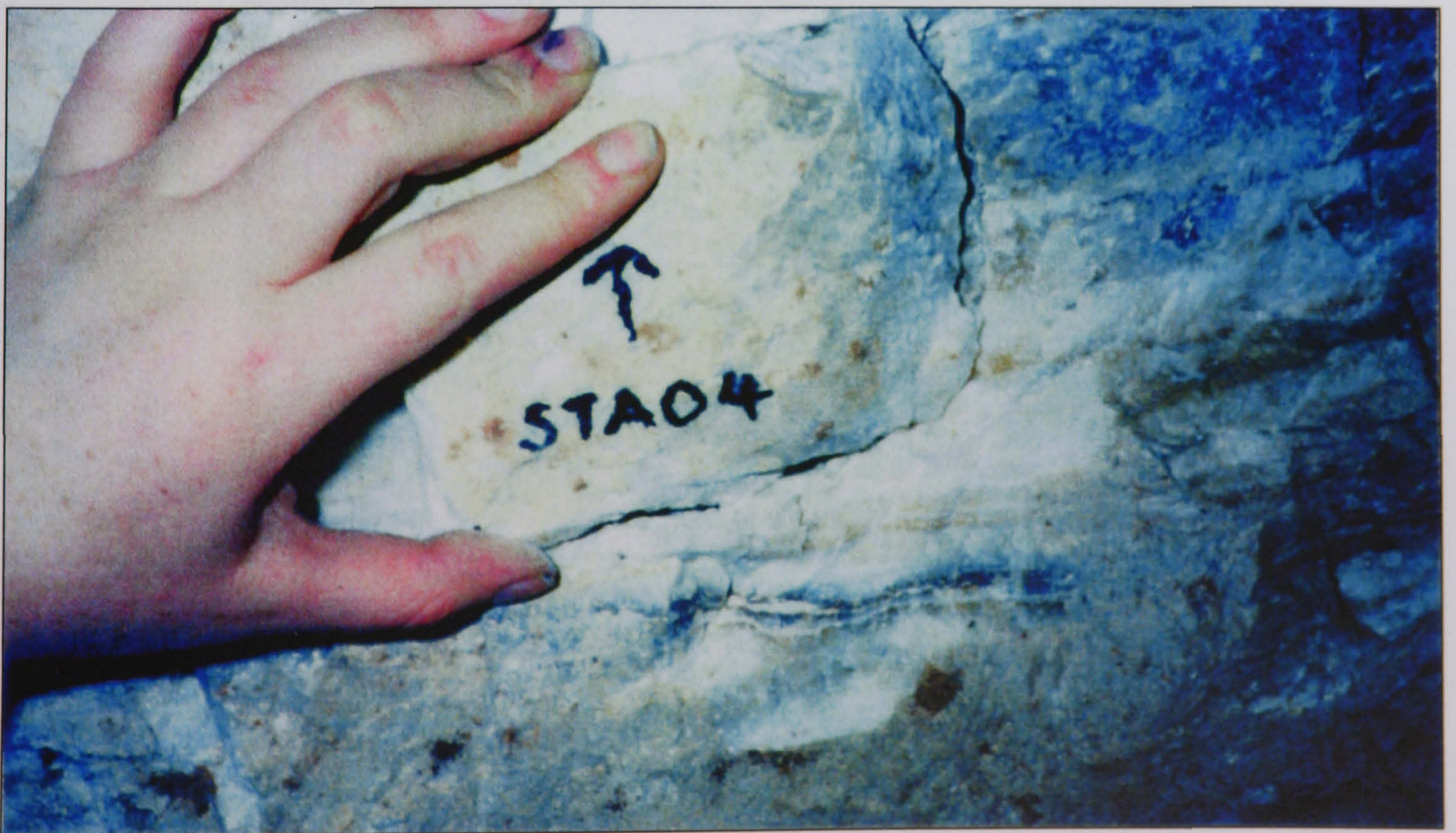
Figure A.6: Photograph of sample STA04 in situ, after removal.
