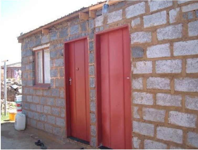
Figure 8-9: Temb 2's outside rooms (author's own 2011).
