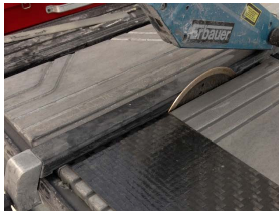
Figure 4.7: Cutting the edge of CFRP.
